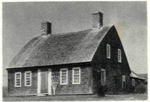
BOWED ROOF was originally a shipwright's fancy, made by bending green timbers over a rock. Later and less skillful builders produced the same form by carving two timbers to produce a continuous curve (see section, right).
