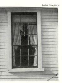
TYPICAL EARLY WINDOW has 15-light sash with nine panes in top frame, six in bottom. "Bottle glass" was used until improved blowing made larger panes feasible. Muntins were flat strips painted black, green or white, according to taste.
