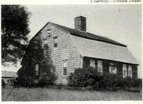
GAMBREL ROOF took house out of cottage category by providing a full second story. Otherwise construction and style were typically Cape Cod. Windows in this house were equipped with inside wind boards rather than shutters.
