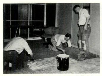
At last—the perfect commercial carpet! Cushionlok combines thick wool carpeting (in the famous-for-wear Gropoint weave) with a built-in sponge rubber back. As shown, it requires no preliminary preparation—can be laid directly on bare concrete, linoleum, wood or plywood!
