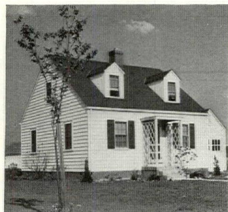
EXPANDED COTTAGE which approaches two-story size, wastes under-eaves space, requires expensive dormer windows in order that occupants may see and breathe.
