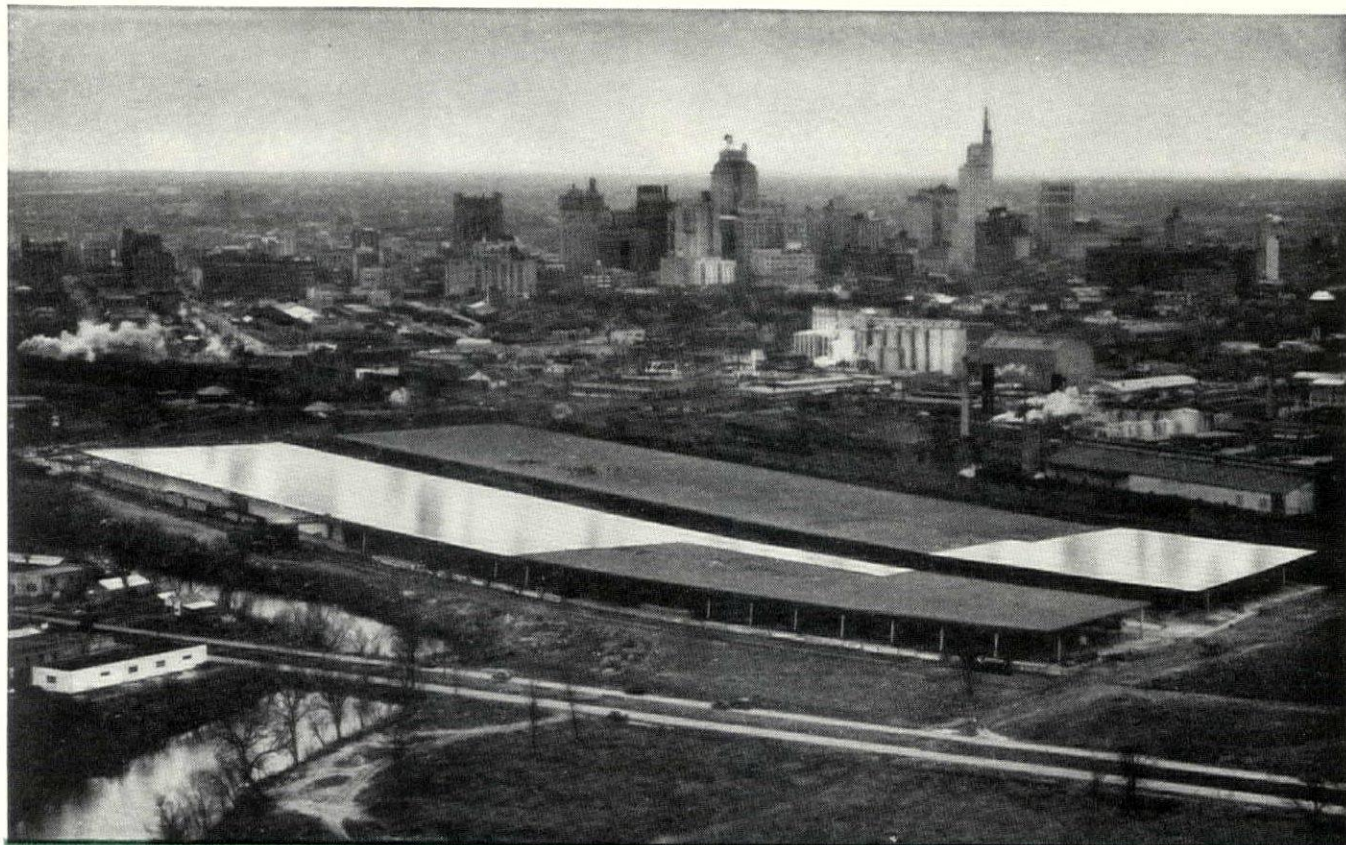
ALFORD REFRIGERATING WAREHOUSES, DALLAS, TEXAS — NOW UNDER CONSTRUCTION, ROOFING CONTRACTOR: LLOYD GRAY, MT. AUBURN ROOFING COMPANY. SPECIFICATIONS FOR THE 23 ACRES OF BUILT-UP ROOF: 2 PLIES OF REYNOLDS .004" EMBOSSED ALUMINUM OVER 30 LB. FELT
