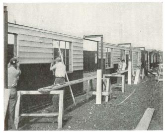
At Peoria, Byrne set up open-air shop, having discovered that rain on the site stops the job even though a roofed-over shop could go right on working. He also introduced aluminum siding above).
