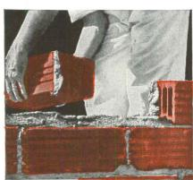
Method 2. A full head joint should be thrown ontone edge of the tile in place and also onto the opposite edge of the tile to be placed.
