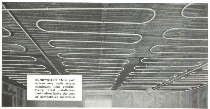
**Bundyweld\*** Steel Tubing is really hot for radiant heating installations.
