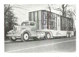
On the Road! Trailer is loaded with structural units and parts on a "first-off, first-up" basis to speed erection at the house site.
