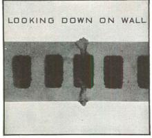
Enough mortar should be used to cause excess mortar to ooze out of the joints on both sides of
