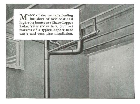
FAST... economical installation has made Chase Copper Tube for soil, waste and vent lines a favorite with builders coast-to-coast! Here's why: You reduce many connections because Chase tube is available in 20 foot lengths. Its light weight makes pre-cutting and pre-assembly possible . . . makes maneuvering and handling quicker!
