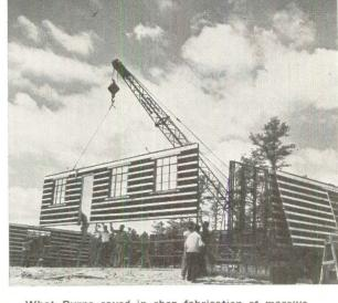
What Byrne saved in shop fabrication of massive steel parts was eaten up by the heavy cranes and trucks necessary to move and erect them on the site.
