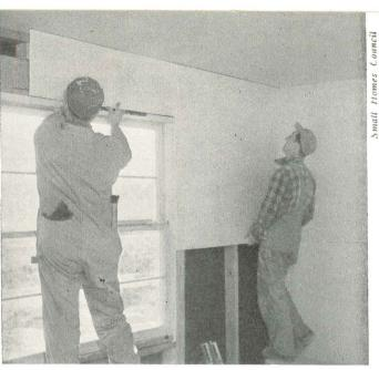
**STUDDING** spaced 2 ft. on center simplified the application of 4 x 8 ft. sheets of plaster board and minimized waste of this material. Absence of partitions facilitated this operation. Note, however, that use of non-modular windows (left) required extra framing members.
