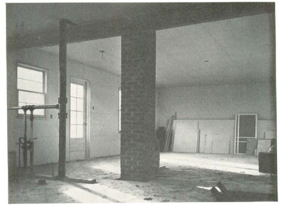
ONE BIG ROOM results when walls and ceiling are dry finished. At this stage partitions were framed on the floor and tilted up. To avoid ceiling damage, they were made a fraction of an inch short and then wedged in place. Millwork was painted prior to installation.
