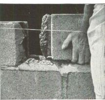
Method 2. A full head joint should be thrown onto one edge of the block already in place and also cuto the opposite edge of the block to be placed.
