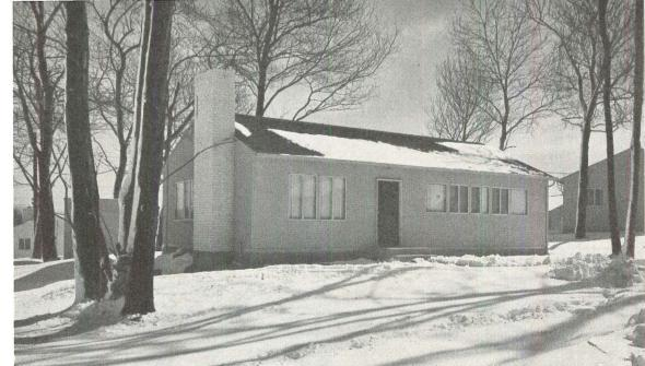
HARMAN HOUSE is steel framed and finished outside with painted steel panels. Large chimney improves its appearance, seems to anchor the house to the ground.
