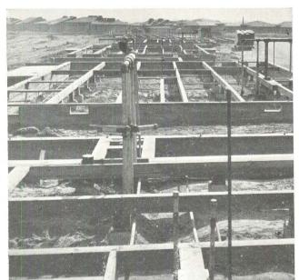
FLOOR BEAMS set flush with foundation top replace usual joist construction and bring house closer to grade to enhance its long, low appearance. Sub-floor of 2 in. tongue and groove planking is covered with oak finish. Burns details only one man to floor laying. "He doesn't waste so much time talking when he has no one to talk to." Plumbing tree is shop assembled.
