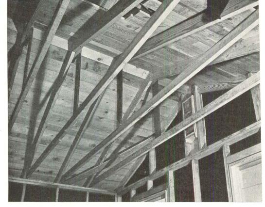
ROOF TRUSSES and gable ends were fabricated on the ground, placed on the plates upside down, then rotated into position. Economical in itself, this trussed roof construction set off a long chain reaction of additional economies. However, maximum economy of truss construction cannot be exploited in a house where framing is complicated by an L-shaped plan.
