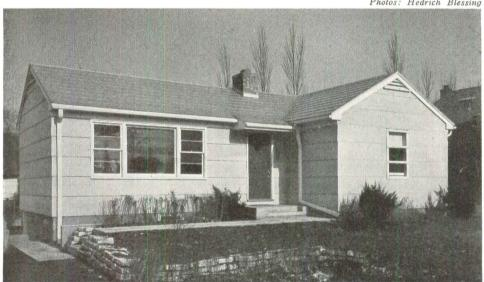
**TEST HOUSE** was built prior to six-house demonstration to gain experience in use of modular plan and framing system (see drawing). It was finished with experimental aluminum roof and cement asbestos panel siding. In actual demonstration (below) walls were framed horizontally and tilted into place.
