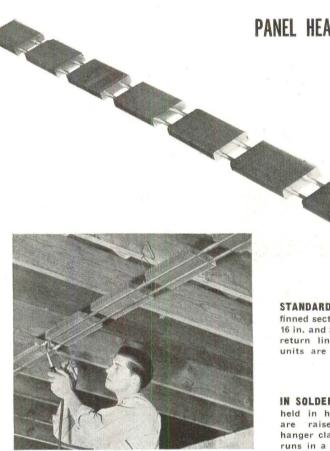
STANDARD 10 FT. KRITZER GOIL has finned sections which fit between 12 in., 16 in. and 24 in. o. c. joists. Supply and return lines as well as return bend units are joined to coil by sweating.
