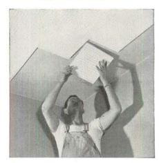
Fiberglas Acoustical Tile can also be easily and quickly applied with adhesives. Because of its low weight and dimensional stability, it offers a high safety factor
