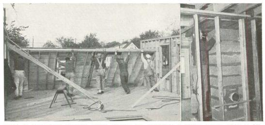
WALL IS SHEATHED BEFORE BEING TILTED UP. CHIMNEY IS BUILT AFTER ROOF IS ON
