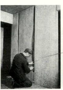
**STRIP OF INSULATION** is inserted in connecting recess between sections of wall before locking strip is set in to cover the Joint, insulation, and wiring.
