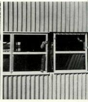
Aluminum windows are put in place, completing exterior of this 91/2 in. thick wall. Wall weighs 25 lb. per sq. ft., costs \$4.78.
