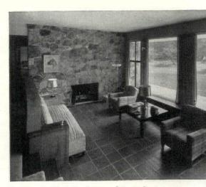
Hollow tile block in cherry red is used for the floors. Although not here an adjunct to radiant heating, it provides an insulated flooring with warm air constantly flowing into the open end panels from the cellar below.
