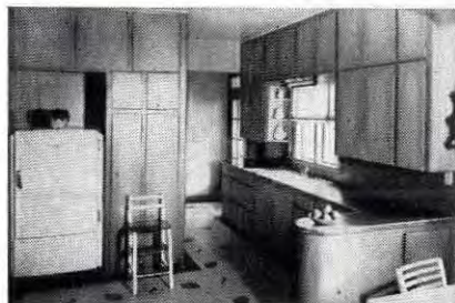
Cabinets, built-ins, storage-walls, sliding doors—whether shop-fabricated, built on-the-job, or constructed by the home owner—all can utilize stock plywood panel sizes.
