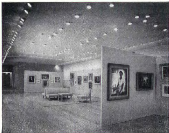
Lighting of main exhibition area above will be changed from incandescents in cans to a combination of cold cathode in coves and incandescent down lighting as in use in other sections.
