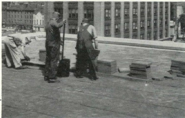
THE ROOF of this fine modern school building is insulated permanently with PC Foamglas. More than 26,000 square feet of 2" Foamglas were applied to the roof deck and covered with roofing materials.
