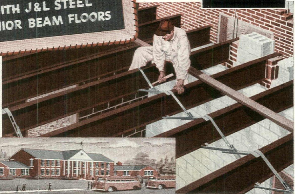
Right: Tightening the rigid bridging between the Junior Beams in the new Brunswick Township, Ohio, High School. Below: Architect's rendering of the new school, now under construction.
