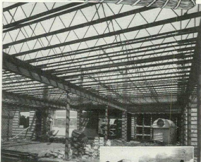
Ritenour High School in St. Louis County, Mo., shown under construction using Laclede Steel Joists. Architect: Wm. B. Ittner, Inc. Contractor: Lecoutour Const. Co. Architect's sketch at right.
