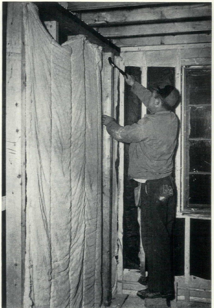
Installing Cellulite Acoustical Blankets The ease and simplicity of soundproofing with Cellulite is demonstrated in the above photograph, where it can be seen that the Cellulite "blankets" are being "hung" by weaving them in and out between the studs.
