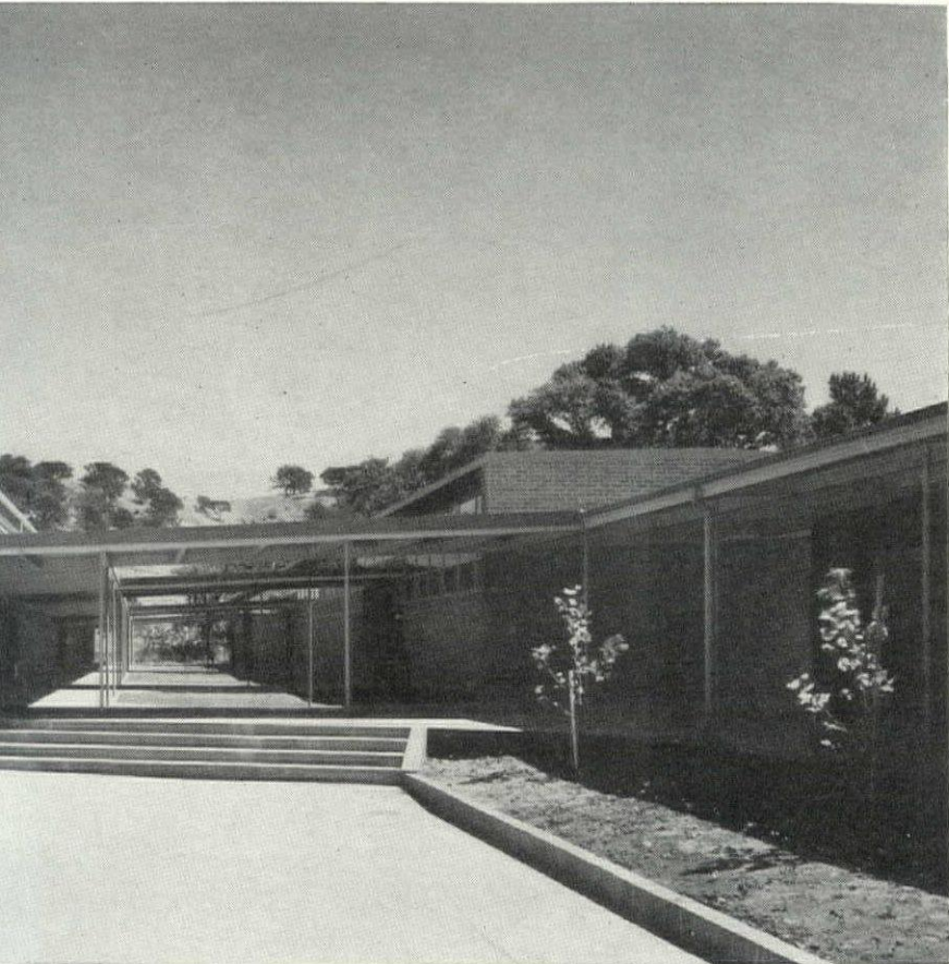
From court outside of multi-purpose room, a view to the west shows the open area and cross corridors between the two classroom wings. Below, an airview of the building with unfinished play yard at right.
