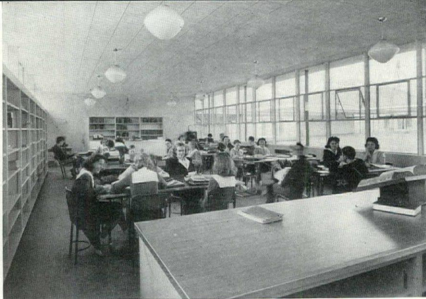
Interior of library shows continuous fenestration along north wall, with tilt-out panels for ventilation. Daylight is also admitted from strip of windows over bookshelves. All parts of room are evenly illuminated.
