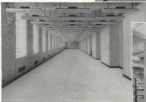
Laboratory—Flush Pilaster Partitions and Wall Lining. Can be subdivided into smaller rooms overnight.
