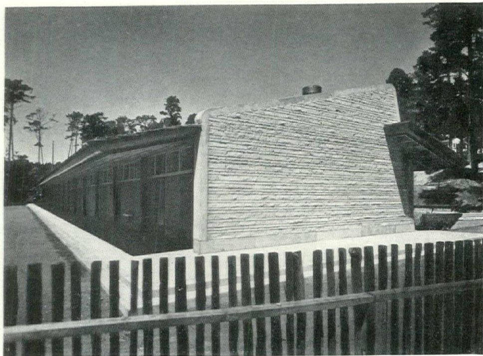
Deep overhang on south wall continues slope of gabled roof and shades south side of the building from direct sunlight.
