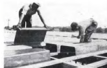
Erecting steelforms on open wood centering preparatory to placing reinforcing steel. Use of steelforms mean a saving in lumber.
