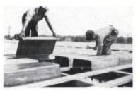
Erecting steelforms on open wood centering preparatory to placing reinforcing steel. Use of steelforms mean a saving in
