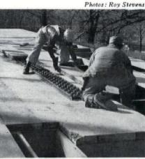
Impregnated felt strips are placed in the horizontal joints of curtain wall panels for waterproofing. On a large project, strips can be cut to size and stapled in place beforehand to speed operation.
