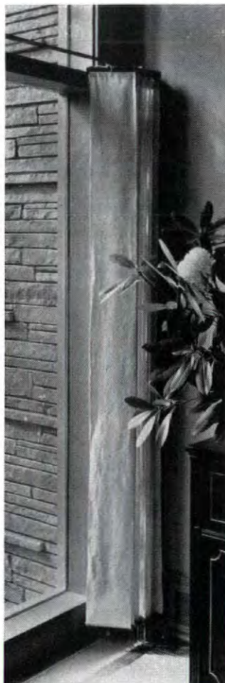
Blind is in two sections, above, for long glass surface. Adjustment of two halves above is different to show how light can be deflected without being barred from room. Blind is particularly effective on east and west exposures.
