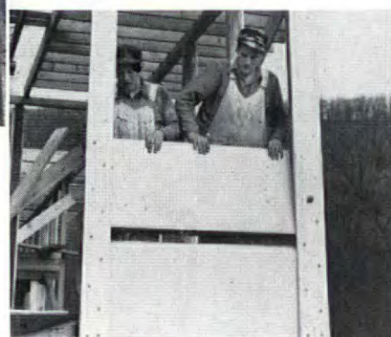
Curtain wall panels, tongued and grooved on the long edges are slipped into place. Mastic is applied along batten edges to insure waterproof joint.
