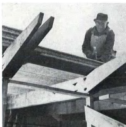
Large lightweight roof planks are easily handled by two men, but roller conveyors assist in moving them long distances.
