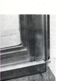
Weatherseal above is in closed position. Below it has been retracted into the jamb to free the sash for turning.
