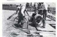
Concrete is being poured here over the steelforms and around the reinforcing steel. The final step is removal of steelforms and step is removal of steelforms lumber after concrete sets.
