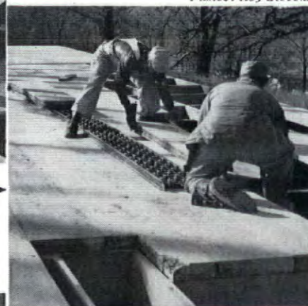
Large lightweight roof planks are easily handled by two men, but roller conveyors assist in moving them long distances.
