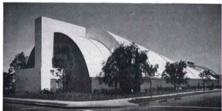
Air-conditioning is handled by a series of grills surrounding the proscenium. Exterior duct and air cleansing plant at rear of theater are clearly visible above.
