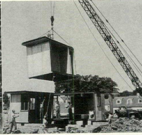
On site, high-boomed crane puts sections in place, with five-man crew, in an hour. House above is older model, rests on piers instead of slab used with 1950 version.
