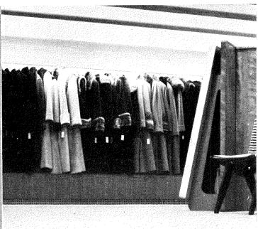
Flexible fixtures are based on L-shaped metal frame into which can be fitted various drawer, hanging rod and display elements, also light fixtures and perforated metal light shields.
