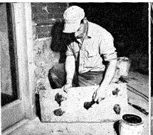
Spotting granite base slab with plasticized resin bonding cement.
