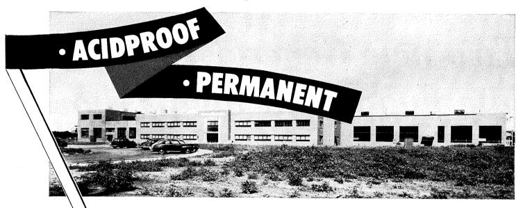
AT THIS LAMINATED PLASTICS PLANT of the General Electric Company, Coshocton, Ohio. PC Foamglas was used in the core walls of storage and processing rooms to help control temperature and humidity. Being a true glass in cellular form, Foamglas is unaffected by moisture . . . is vaporproof. Engineers & Builders: The Austin Company, Cleveland, Ohio.
