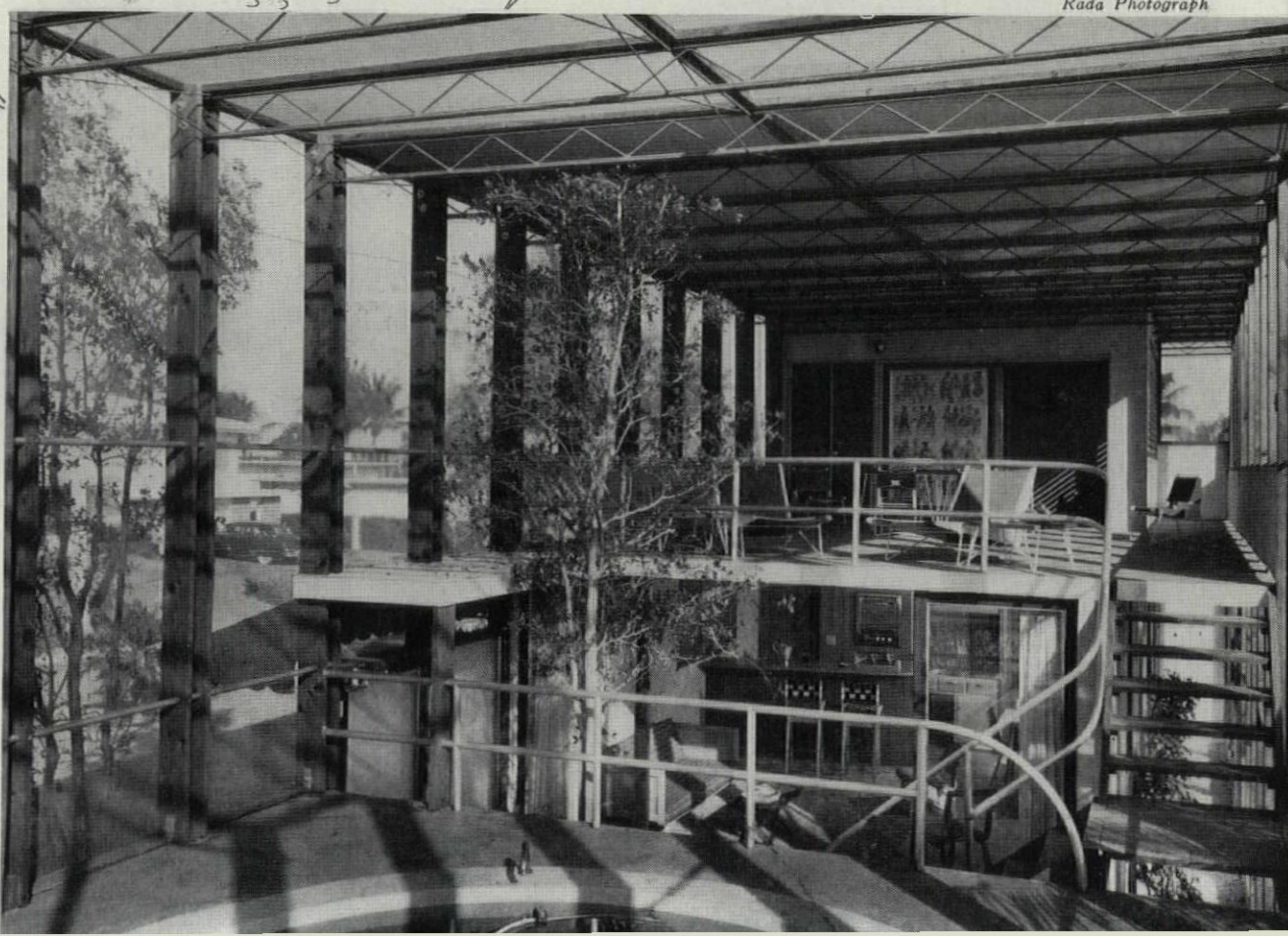
Cut away drawing shows how small the four room house inside the bird cage is—a bedroom, kitchen, and half-open living room below, a lanai with one sliding glass wall behind the porch above. Photo below shows the house across the roofless swimming pool. Note how the overhang is concealed inside the bird-cage frame.
