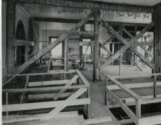
LINCOLN STUDY, on second floor, shows type of support that was used to bolster White House.
