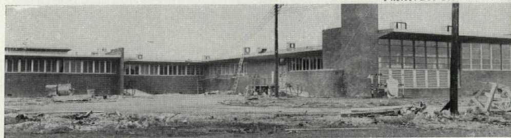
North view with service wing at right
