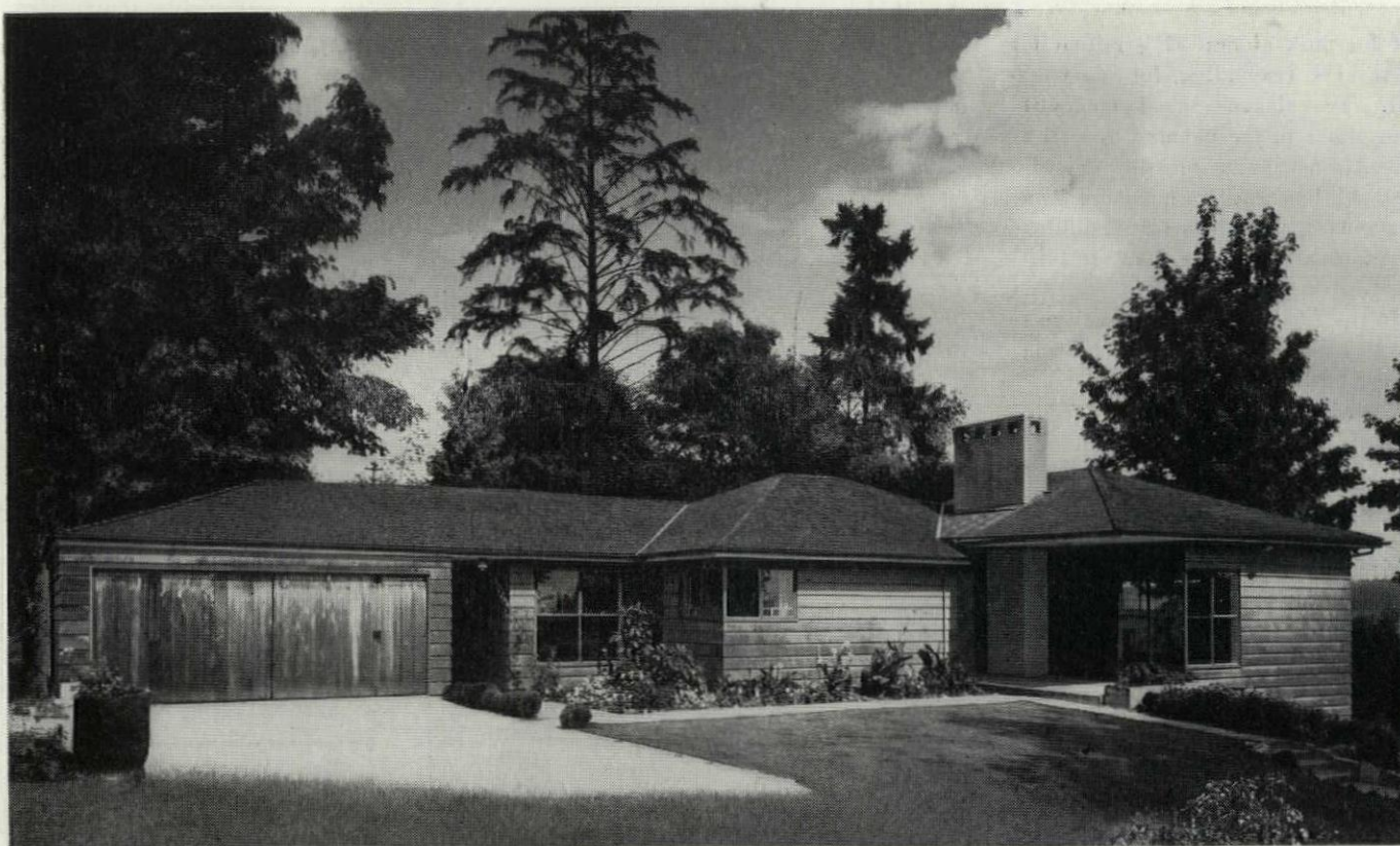
Lloyd Ulrich, Architect
