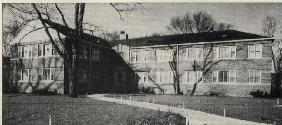
EUCLID, O., APARTMENT, Jos. Augustas, builder and architect, 25941 Lake Shore Blvd. City Plumbing & Heating, pioneers and largest installers in the midwest of radiant heating, were contractors and engineers for this installation also. Dr. S. T. Thomas is the owner. The Baird-Foerst Corporation, Cleveland, is the A. O. Smith distributor.
