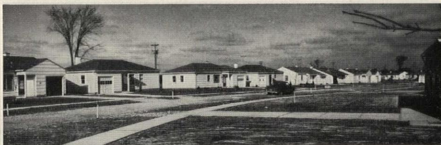
100 SMALL HOMES in Parma Heights, Cleveland, are equipped with A. O. Smith gas-fired, forced-circulation hot water boilers for radiant floor panel installations. Precision Housing Corp., Morris Fishman, president, built the hundred houses in 1949. One hundred more of these homes will be built in Parma Heights this year.
