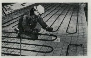
Preshaped fittings are welded to straight piping for radiant panel. Another kind of Redi-Bend is merely coupled to the pipe with a monkey wrench.
