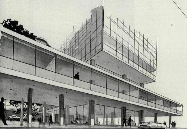
and a movable scaffold system to wash windows and spandrels alike from the outside. It will cost \$6 million to erect its 4,000,000 cu. ft. on leasehold land—nearly three times as much per cubic foot as some Rockefeller Center units erected in the depression.
