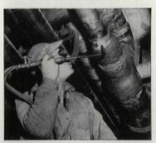
Installing a Walseal fitting at UN, on location; note operator progressively heats small section of the fitting
