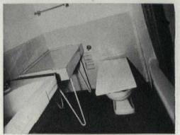
Dressing stand in bathroom was a bright idea, finally dropped to save cost of extra mirror, and align all plumbing fixtures back-to-stack.
