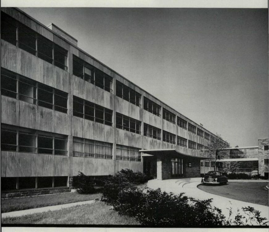
The north face of the building allows glareless light into all laboratory room Its free-standing, glass-enclosed entrance portico is dignified and emphatic wi out taking up valuable building space. The animal building (right) is of so masonry with small windows provided in case of air conditioning breakdow
