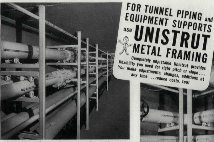
Unistrut steel channel and fittings, roller pipe supports and concrete inserts at work in a tunnel installation at G. D. Searle & Co., Skokie, Illinois, manufacturers of ethical pharmaceuticals.
