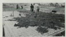
Here SISALKRAFT is shown laid over subfill, with concrete mix being spread over SISALKRAFT and reinforcing rods.
