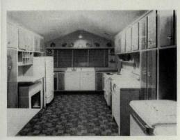
Kitchen is lined with equipment, has gabled ceiling to accommodate air conditioning ducts.
