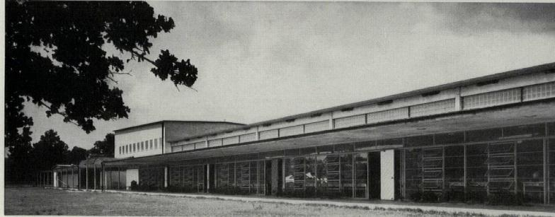
The all-glass wall, with a recessed clerestory to bring light farthe into the room, faces east because of the requirements of the lot. The wide canopy over the outdoor passage is cantilevered to avoid the disturbance of posts in front of the classrooms. Plants take the place of the usual window-sill wall in cutting off outdoor glare.
