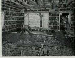
From 1½ to 2 in. of concrete surround the ducts. Pipes are protected from wheelbarrows and other heavy loads during the concrete laying process.
