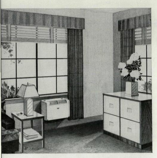
Interior sketch shows how the builder's unique installation takes full advantage of the flexibility of Frigidaire window type air conditioners. Although these units are primarily designed for window installation, here they are actually sealed into wall apertures below the window—giving them an attractive, built-in appearance.
