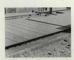
HEATING SYSTEM detail in picture above shows steel panels in place before sheet metal is welded to header void, providing a completely closed circuit. System is zoned. Layout of system (right) shows that supply channels were
