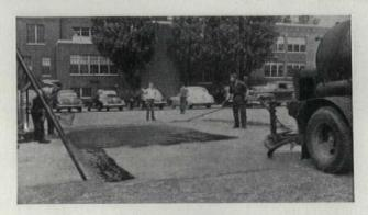
A stone base is sealed with hot-mix asphalt, then covered with ½ in, of ground rubber which is rolled to impregnate rubber particles into asphalt.
