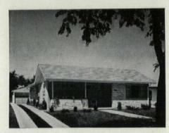
L-SHAPED HOUSE PLAN (above) can be reversed to provide two distinct elevations from street side. House above shows eave line to street, with slight change from basic plan in main-entrance detail.
