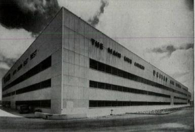
New United Air Lines maintenance base has maintenance-free walls of J-M Corrugated Transite.
