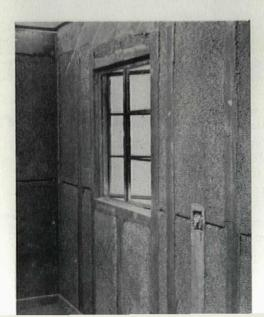
Unfinished interior shows stud spacings after planks have been removed. Conduits are cut into wall easily before plastering.
