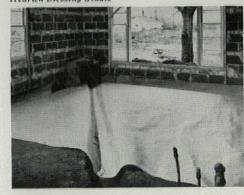
Key to proper installation is moisture barrier under slab of waterproof, reinforced paper or 55 lb. roofing felt. Joints must be sealed.
