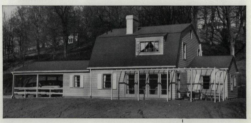
In this home, Reynolds Aluminum is used in 21 forms. These include windows, insulation, gutters and downspouts, thresholds, storm doors and windows, duct work, louvres, nails, weatherboard corner pieces, basement grills, flashing, trim molding, screens, aluminum paint for prime coating. Details of major building products are presented above.
