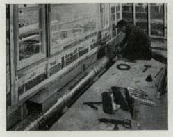
Sheet metal forms hold the ducts in place while concrete is poured. Register openings are covered to keep out dirt during construction.
