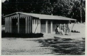
Aluminum vacation house goes up fast, needs no finish. Tension cleats assure rugged assembly.
