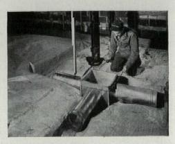
Warm air furnace sits on top of pit or plenum chamber. This installation has three radial ducts rather than four which are more usual.
