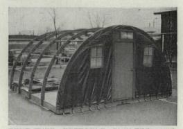
TENT-TYPE PORTABLE SHELTER, envisioned as one type of emergency housing in case of war, was developed by Army Quartermasters. Made up of preassembled wood floor panels, rigid arch framing, and insulating blanket cover, it is of knock-down construction, and can be erected by five men in one hour. Basic unit is 16 x 16 ft., can be increased in length to 24 ft.
