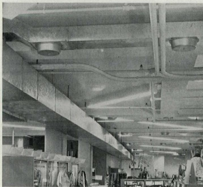
Two header ducts run the length of each floor carrying air to a dozen 14 x 7 in. run-out ducts that fit under beams. When ducts were painted to match ceilings they became much less conspicuous.
