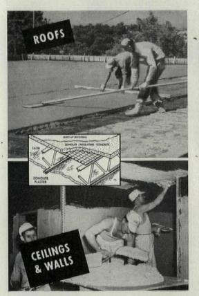
Illustrated above (upper) the use of Zonolite concrete for the roof deck and (lower) of Zonolite plaster for walls and suspended ceilings. Combinations of 2" vermiculite concrete topping with a 1" vermiculite suspended ceiling over face of metal lath have received a 4-hr. fire-rating from Underwriters' Laboratories.
