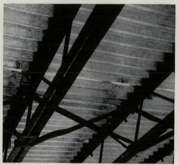
—because Corruform was developed to provide an extra-tough, secure steel base which maintains structural principles and structural integrity.
