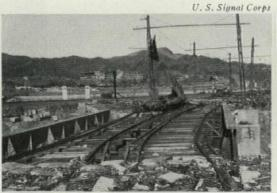
840 FT.: from "ground zero" (point beneath explosion) terrific blast moved bridge 3 ft., bending rails but leaving steel poles standing.
