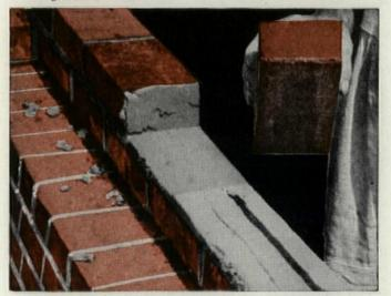
A good bond was not secured here because the brick on which the mortar was spread had sucked the mortar dry, before the brick was laid.
