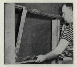
4. Aluminum ventilators of projected type are inserted into openings of wood frame in a bed of glazing compound. Wood screws hold them in place.
