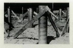
Simple lumber bracing devices will keep the fiber forms aligned as the concrete is poured into them.
