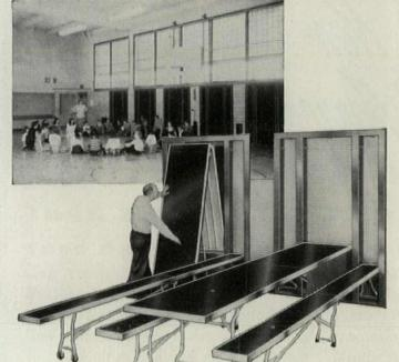
Tables and benches for 200 can be rolled down from the wall in 8 minutes.
