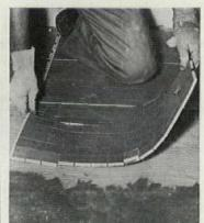
When a "floating" process is used, mastic is spread 1/16 in. thick.
