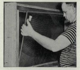
5. Thermopane (standard  $42\frac{1}{2}^{\prime\prime} \times 22\frac{1}{2}^{\prime\prime}$  unit) is installed in aluminum ventilators as in any other face-glazed metal sash. Aluminum screen is installed from inside.
