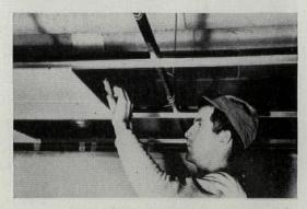
runner. Each tile is thus rigidly supported by an I runner flange and two reinforcement T spline flanges, yet may be removed easily at any time for access to area above. Tiles  $12 \times 24$  in. are applied with the long dimension parallel to the runner. Erection costs are about 10 cents per sq. ft. for labor,  $9\frac{1}{2}$  cents per sq. ft. for materials exclusive of tile.
