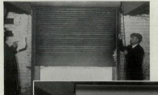
The door at left has been in continuous service since 1903—for 47 years! The picture was taken this year, just before curtain slats were replaced and a few minor repairs made. In the photo below, the door is ready for many more years of efficient service and protection.
