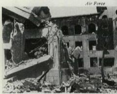
1300 FT.: reinforced concrete school suffered roof collapse when columns on blast side gave way. It was completely burned.
