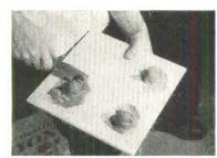
First, with a putty knife or small trowel, a little of the cement is scraped onto the tile to serve as a primer for the spots where the cement will go. Then, the cement is applied in heavy gobs, about the size of a walnut—four to a square-foot tile. Gobs should be kept about an inch from outside edges.
