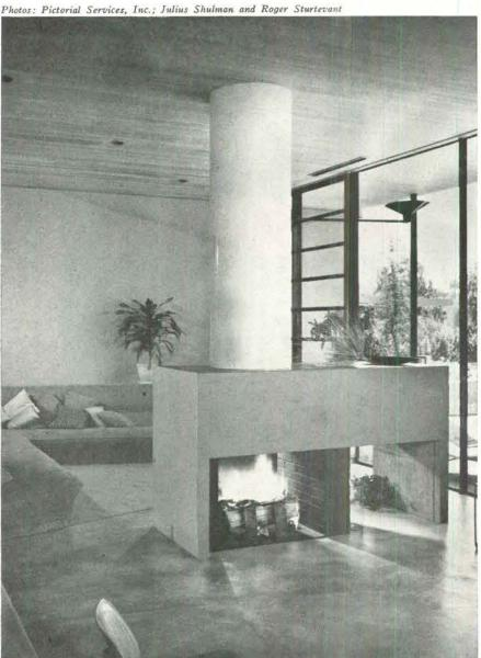
Middle-of-the-room fireplace, designed by Architects Eero Saarinen and Charles Eames, demonstrates clean, open effect that can be achieved with non-masonry fireplace construction. Flue is asbestos board.
