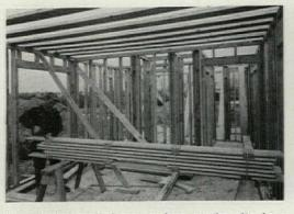
window wall frame arrives at the site in a single package. Two men can assemble and tip it into a prepared opening in about 20 minutes.
