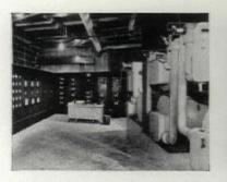
Equipment room of a large office building where Trane centrifugal refrigerating units supply chilled water in an extensive Trane "undivided responsibility" air conditioning system.
