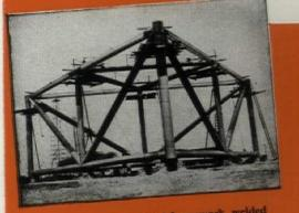
3. Completed framework, welded and watertight except for the corner verticals, which will accommodate anchor spuds.
