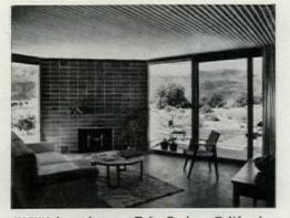
IN THIS desert home at Palm Springs, California, Kaiser Aluminum corrugated roofing is used in the living room ceiling to diffuse sound and carry the attractive exterior corrugation design inside the house. The corrugations deflect and hinder movement of sound waves.
