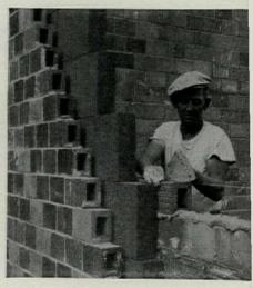
• PC Foamglas is widely used for freestanding walls and partitions and in corewall construction between inner and outer masonry as shown here at the new meat processing plant of Stadler Packing Company, Inc., Columbus, Ind. Foamglas acts as a long lasting barrier to vapor and heat transfer ... helps maintain required operating temperatures. Architects: Johnson and McKenney, Columbus, Ind.
