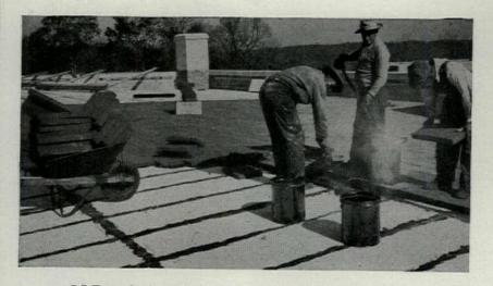
• PC Foamglas is used to insulate this roof of the new, modern synagogue for Adas Israel Congregation, Washington, D. C. Architects & Engineers: Frank Grad & Sons—General Contractors: M. Cladny Construction Co., Inc.—Roofer: Warren-Ehret Company—all of Washington, D. C.
