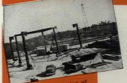
Construction of ipe frame float 30' nigh, 80' long on each side of the triangle.
