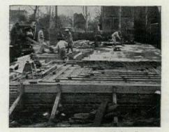
Today steel pipe coils are embedded in floors or ceilings during initial construction to provide advantages of radiant heating.
