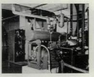
This Trane Condensing Unit is perfectly matched with Trane Direct Expansion Coils to form the heart of a Trane system for the coffee shop of a large hotel.
