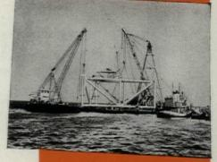
5. Launching the 60ton float. Note work platform erected 10 feet above framework.
