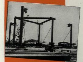
2. Closer view of the starting framework, showing 22" diameter steel pipe being used.
