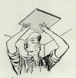
7. First, cement a single acoustical tile to the painted ceiling surface, and leave it there for a 48-hour period.
