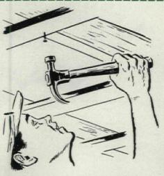
Wood joists or studs. Cross-fur with 1" x 3" strips, on 12" centers, and level for application by nailing or screwing; or fur on 16" centers and apply gypsum base. Either of these methods can also be used when preparing metal ceilings.
