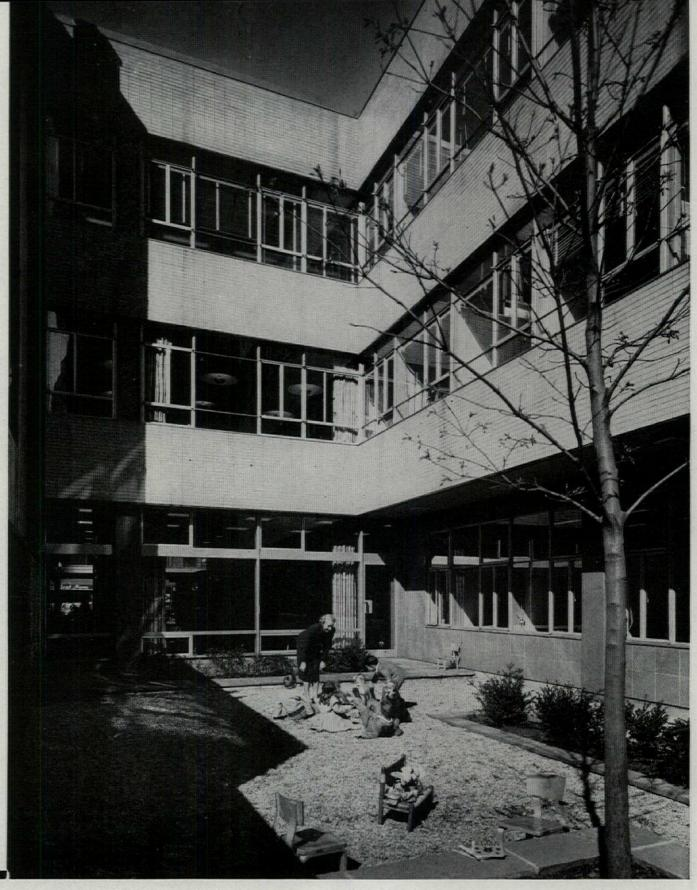
cluding even the structural angle lintels over the windows. We believe this is the first such use of aluminum lintels; but with the advent of aluminum windows this seems a reasonable step. It is hardly economical to swing a scaffold over the face of a building merely to paint lintels.
