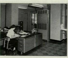
Available in both 3- and 5-ton sizes, these Frigidaire self-contained air conditioners can actually be employed to handle almost any air conditioning need. With the addition of optional heating coils, they provide year round service.
