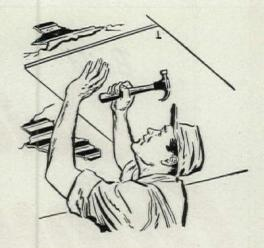
Unsound plaster. Repair by nailing 3/8" thick gypsum lath directly over the plaster. Nails should be driven into joists. If wood joists are not available, cross-fur with wood strips on 16" centers and nail gypsum lath directly to furring.
