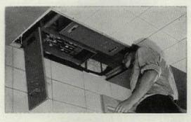
Dark runs on either side of the ceiling mark paths of bus duct in Electrical Engineering Building. Westinghouse
