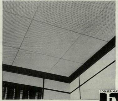
These are 24 x 24-inch Transite Acoustical Panels. Notice how precisely the beveled units come together to form a ceiling that is exceptionally flat and true. Transite Panels may also be obtained with square edges when it is desired to minimize tile lines and promote the appearance of an unbroken perforated area.
