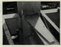
angle is shop welded to column for bolting beam in the field. Outside cover plates are then field welded to top and bottom flanges and the top plate to column in flat position with Lincoln"Fleetweld 5" electrodes. Bottom plate
