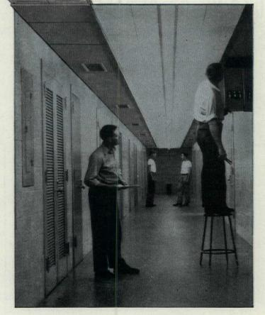
Ceiling panels provide access to entire length of duct.
