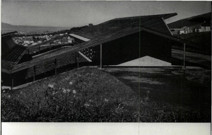
walls are of lightweight concrete blocks of integral buff color. (The buildings are on double flat slabs and are framed with light steel to permit wide openings for natural lighting.) And the ice plants covering the slopes are rich in texture.
