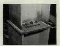
Fig. 1. Typical Welded Splice of all columns 12 to 12 and 12 to 14 WF column. Bearing plate is shop welded to lower column . . . clip angle for erection bolts is shop welded to upper column. All field welds are made in fast, easy downhand position
