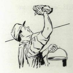
New plaster. Wash white coat finish with a 10% zinc sulphate solution to remove free lime. If porous, prime with Armstrong's Wall Size. Acoustical materials can also be applied direct to dry, thoroughly seasoned brown coat of plaster.
