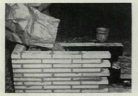
To assure complete fill of the air space, insulation is merely dun ped from bags into the cavity about three times during the progress of the wall.
