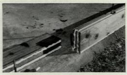
The planks may be erected on a slab (as pictured above) or over a conventional basement foundation. As each predrilled timber is passed down over the rods it is calked along the grooves for protection against the weather. Corners (below left) are formed by a 4 x 4" vertical member milled to fit the end-matching of the 4 x 8" horizontal wall members. Lag bolts tie the corners together. Door and window frames (below right) are held in place
