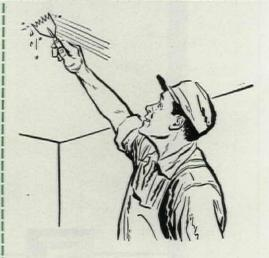
3. If the paint has softened, remove paint by scratching or with paint remover. Then acoustical tiles can be cemented.
