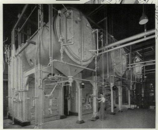
In a modern central heating plant at St. Mary's Hospital, LaSalle, Ill.; three KEWANEE Hi-Test Boilers are capable of producing 18 million Btu hourly.
