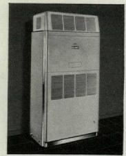
Three 5-ton units like the one in this anteroom are used to condition the 12th floor. Cooled air from the units is distributed to individual executive offices through insulated ducts placed in an attic space directly above the ceiling.
