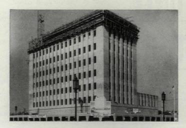
Forms were built by placing 5%"-thick PlyForm panels across 2"x4" studding, backed by double 2"x4" wales. Forms were built-up in 16-foot long sections which were stripped and recrected as pouring progressed. The plywood forms were re-used to job completion with an average of from 6 to 8 re-uses obtained from each of the panels.
