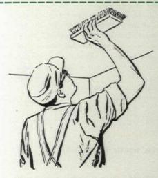
New concrete. Remove lime with zinc sulphate solution (1 lb. to 1 gal. of water), and allow to dry thoroughly. If oil has been left by concrete forms, remove by scrubbing with washing soda, rinse, and treat with zinc sulphate.
