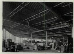
Standard joists span up to 32 feet and Longspan joists up to 64 feet. By using these maximum spans, the number of columns are reduced and more manufacturing area is made available.
