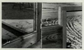
by the tongues and grooves of adjoining and top and bottom timbers. Fixed sash windows of all-cedar construction with adjustable ventilators may be obtained from Apex or purchased locally. The threaded collar (below left) beneath the top plate ties the timbers tightly together. Flat roofs are bolted into the wall in the same way as the wall logs are fastened to the foundation (below right) and
