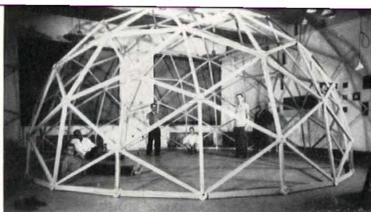
MIT student Zane Yost built simple geodesic dome frame (above) using only $22 worth of material.
