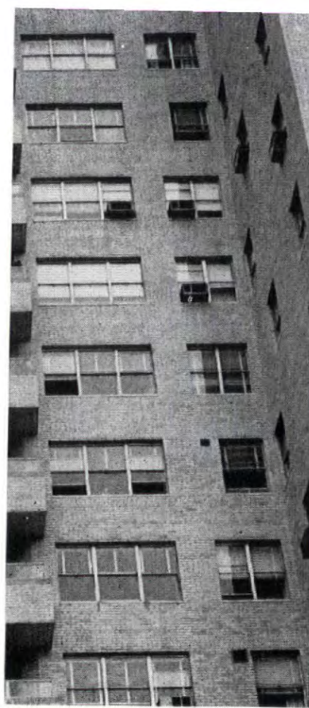
Typical new luxury apartment, left, shows the high proportion of tenants who put in air conditioning individually (note unit air conditioners in windows). In Rittenhouse apartments (above) small intake grilles in walls under windows replace unit boxes hung in windows.
