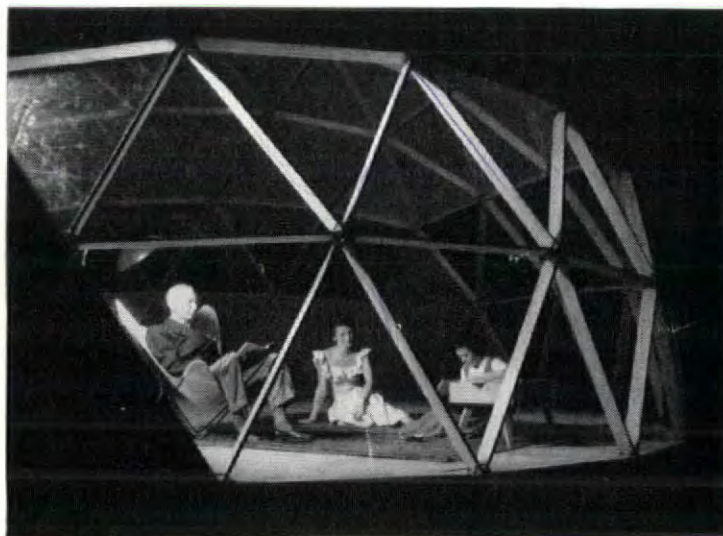
"Skybreak" dome sells knocked down in Montreal for $800. Made of plywood with plastic glazing, and foil insulated, the frame takes 60 man-hours to erect.
