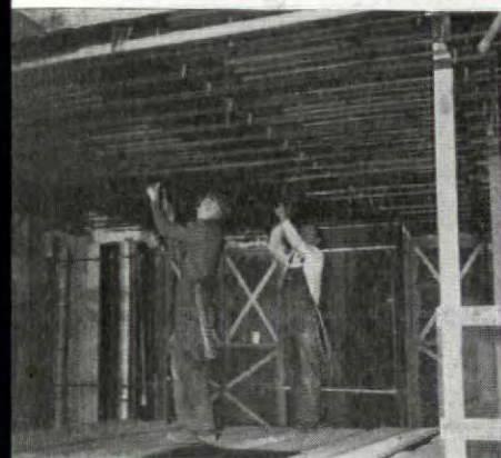
Photographs of Sinclair Oil Building in construction show how simple it is to fireproof steel beams with a hung ceiling instead of upholstering them individually.
