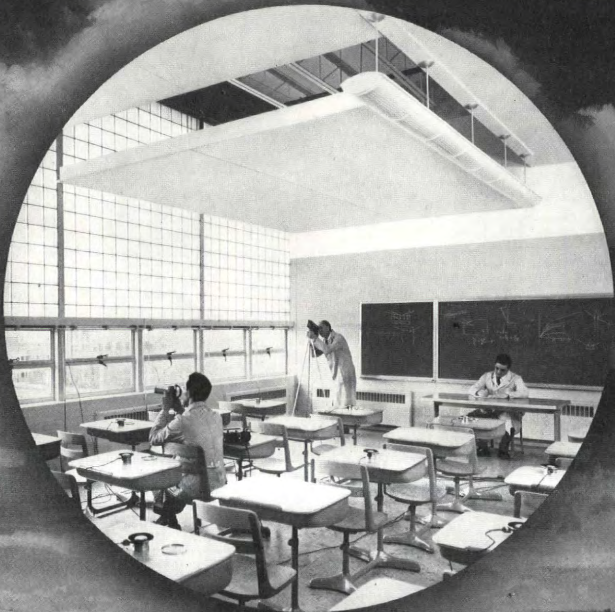
Technicians studying daylight illumination in the Test Room section of the Daylight Laboratory. Special light meters on desk tops read and automatically record illumination twenty-four hours a day throughout the year.
