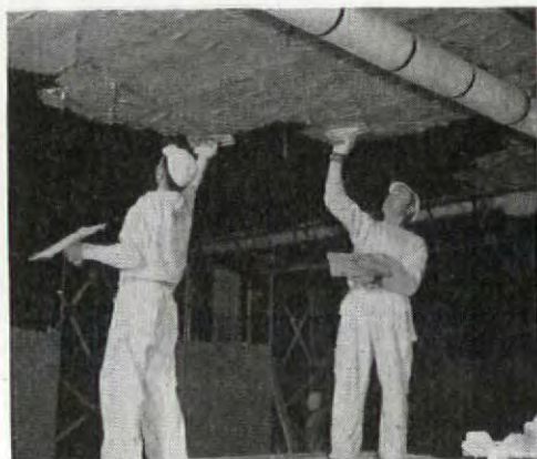
Photographs of Sinclair Oil Building in construction show how simple it is to fireproof steel beams with a hung ceiling instead of upholstering them individually.
