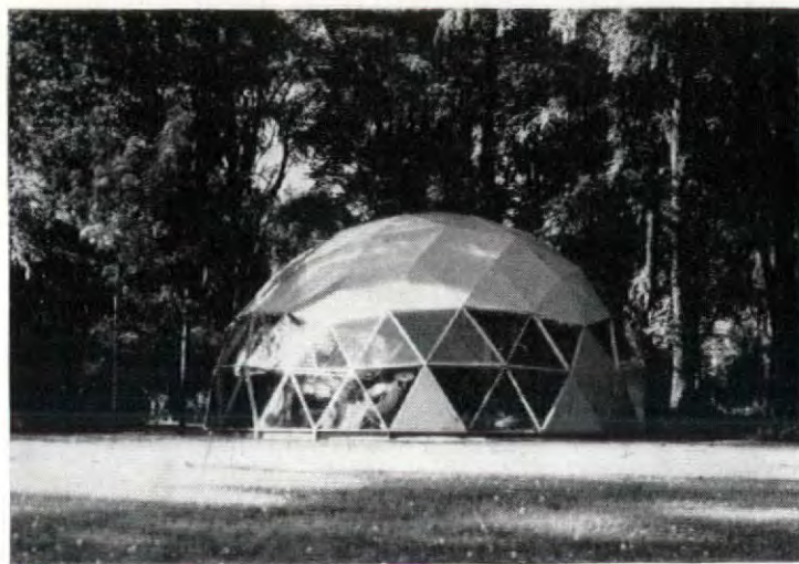
"Skybreak" dome sells knocked down in Montreal for $800. Made of plywood with plastic glazing, and foil insulated, the frame takes 60 man-hours to erect.
