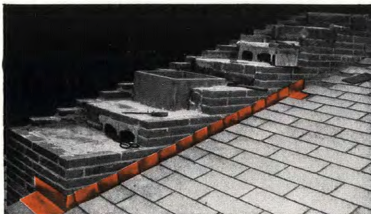
1 Copper base flashing being installed. Note how flashing is interlaced with shingle courses.
