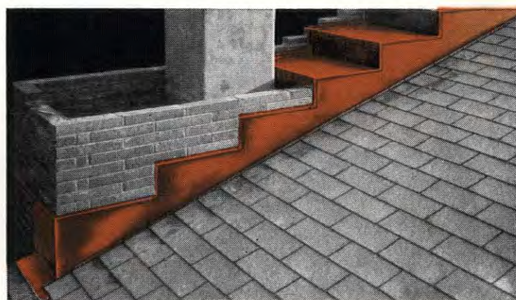
3 Brickwork resumed. Space within will be filled with masonry rubble.
