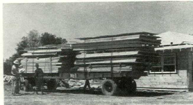
At Baton Rouge, panels for 8 houses a day are made on jigs, then everything for one house is loaded together on trailer. New Orleans is 90 miles away.
