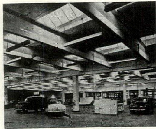
Typical of Europe's prestressed concrete achievements is the 165' x 230' Chevrolet Garage in Brussels, Belgium. It uses prestressed 66' girders (59" deep) and 44' prestressed beams (39" deep) to support the roof of hollow brick (prefabricated into slabs) and concrete skylight frames (cast in place). Few in number, the 20 x 20' columns are of cast-in-place concrete. (Photo: Portland Cement Assn.)
