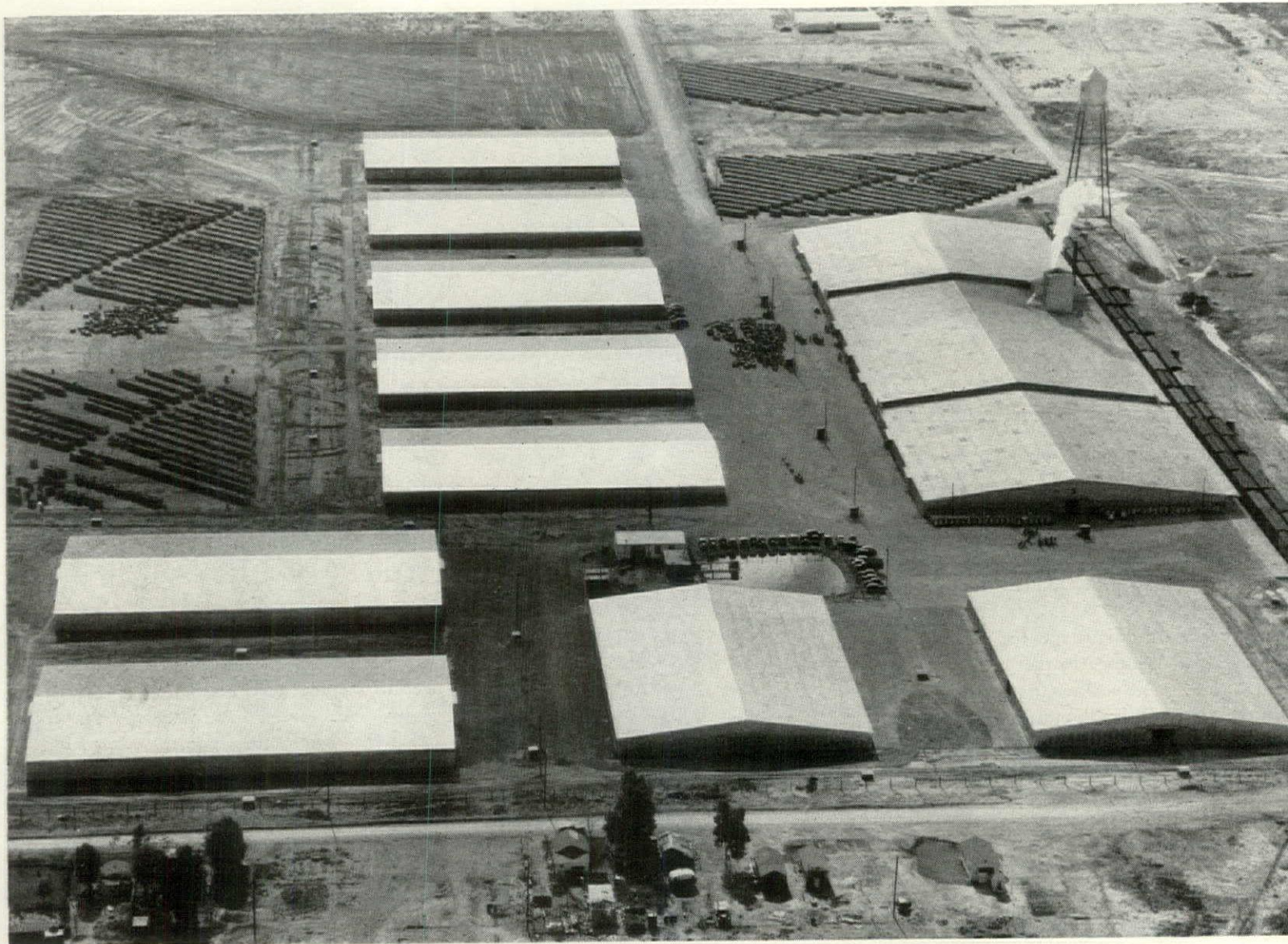
THESE TEN BUILDINGS of the Calcot Compress & Warehouse of the California Cotton Cooperative Association, Bakersfield, are entirely covered with Kaiser Aluminum corrugated roofing. One of the largest
