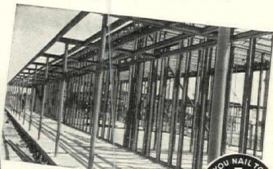
Corridor detail of school showing Stran-Steel Framing.
