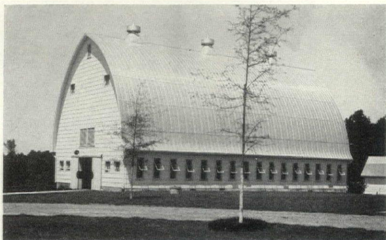
CONVENTIONAL STANCHION barn is framed with modern laminated wood rafters, but structural change does not produce new plan.
