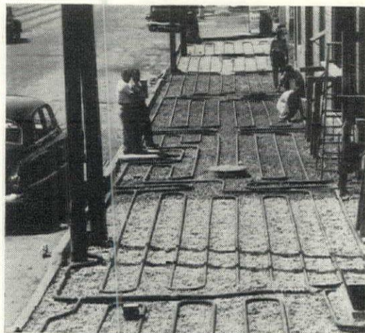
A typical sidewalk snow melting installation showing an effective layout of steel pipe coils.
