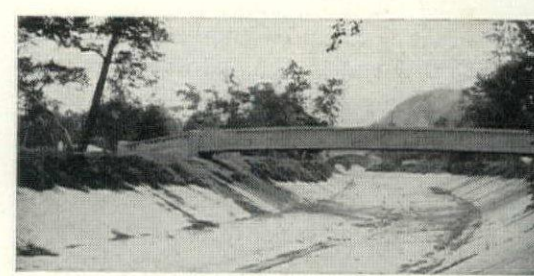
Pedestrian bridge spanning flood disposal channel in Arroyo Seco Park near Los Angeles is comprised of two 110' long prestressed concrete girders 68" deep with a 10" thick web and 20" wide flange. Before they were laterally tied together with a poured concrete deck, each girder was so limber it would flex under the weight of a man leaning against it. Even at that, the girders are admittedly overdesigned; they could be only 56" deep with a 6" web. (Prestressed Concrete Corp.)
