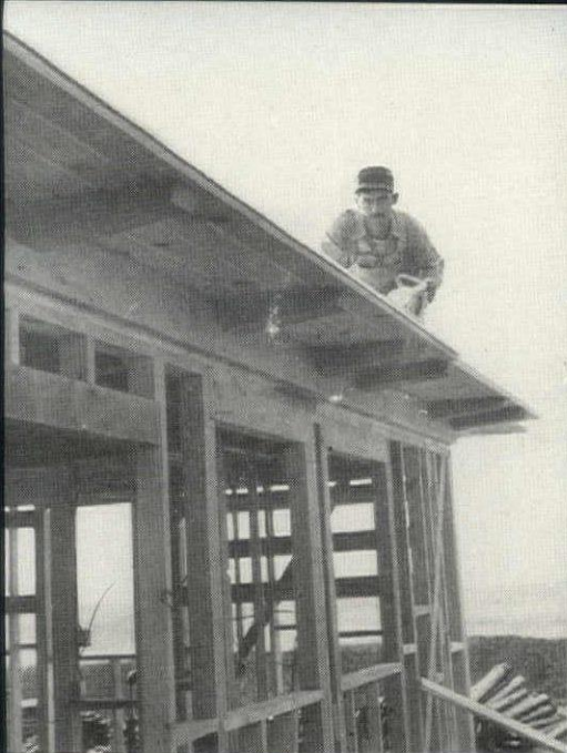
Flat roof saves material, gives safe platform for workmen. Man is sawing roof decking to accommodate fascia board that is also gutter. Drawing shows details.
