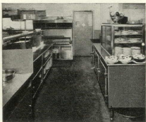
Gleaming main kitchen, with stainless steel salad table at right refrigerated by remote Frigidaire Meter-Miser compressor.
