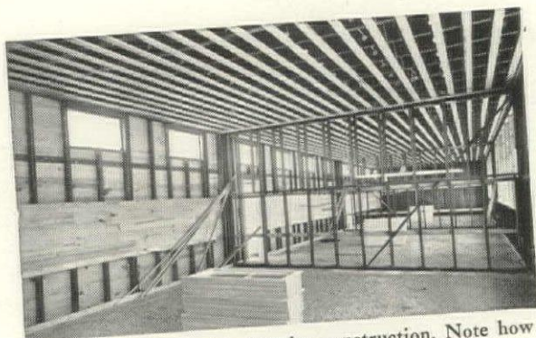
Exterior view of school. Electrical wiring is installed through factory-punched holes in frame members.
