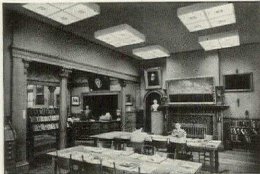
This high-intensity installation of surface-mounted SKYLIKE units was selected for the modernization of the Amesbury, Massachusetts Public Library. Note the low brightness levels at the light source . . . the 90° shielding . . . the absence of harsh shadows and sharp light cut-off lines.
