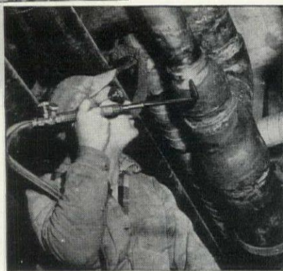
Installing a Walseal fitting at UN, on location; note operator progressively heats small section of the fitting.
