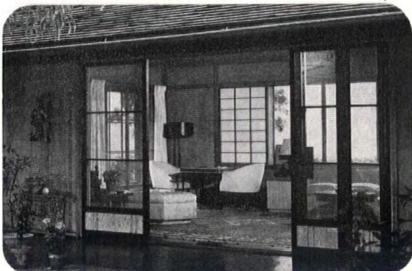
View into living room shows sliding screens and windows designed according to Japanese patterns.
