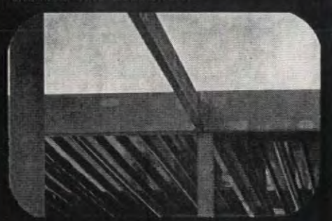
Complete steel deck was erected in 10-hours by 2 welders.
