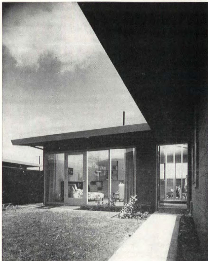
Entry walk from street through inner court is protected by 3' 6" overhang of bedroom-wing roof. Glass wall of living room looks out on private patio, gives interior added light and space.
