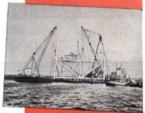
5. Launching the 60-ton float. Note work platform erected 10 feet above framework.
