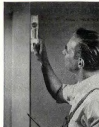
Viewed from any position, the vial-bubbles on both transparent plastic levels are plainly visible.
