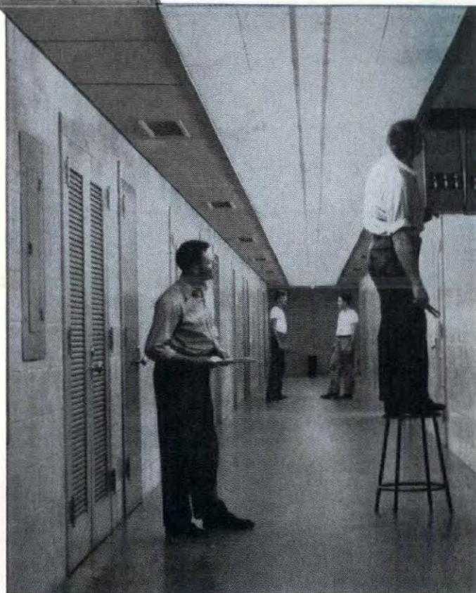
Ceiling panels provide access to entire length of duct.
