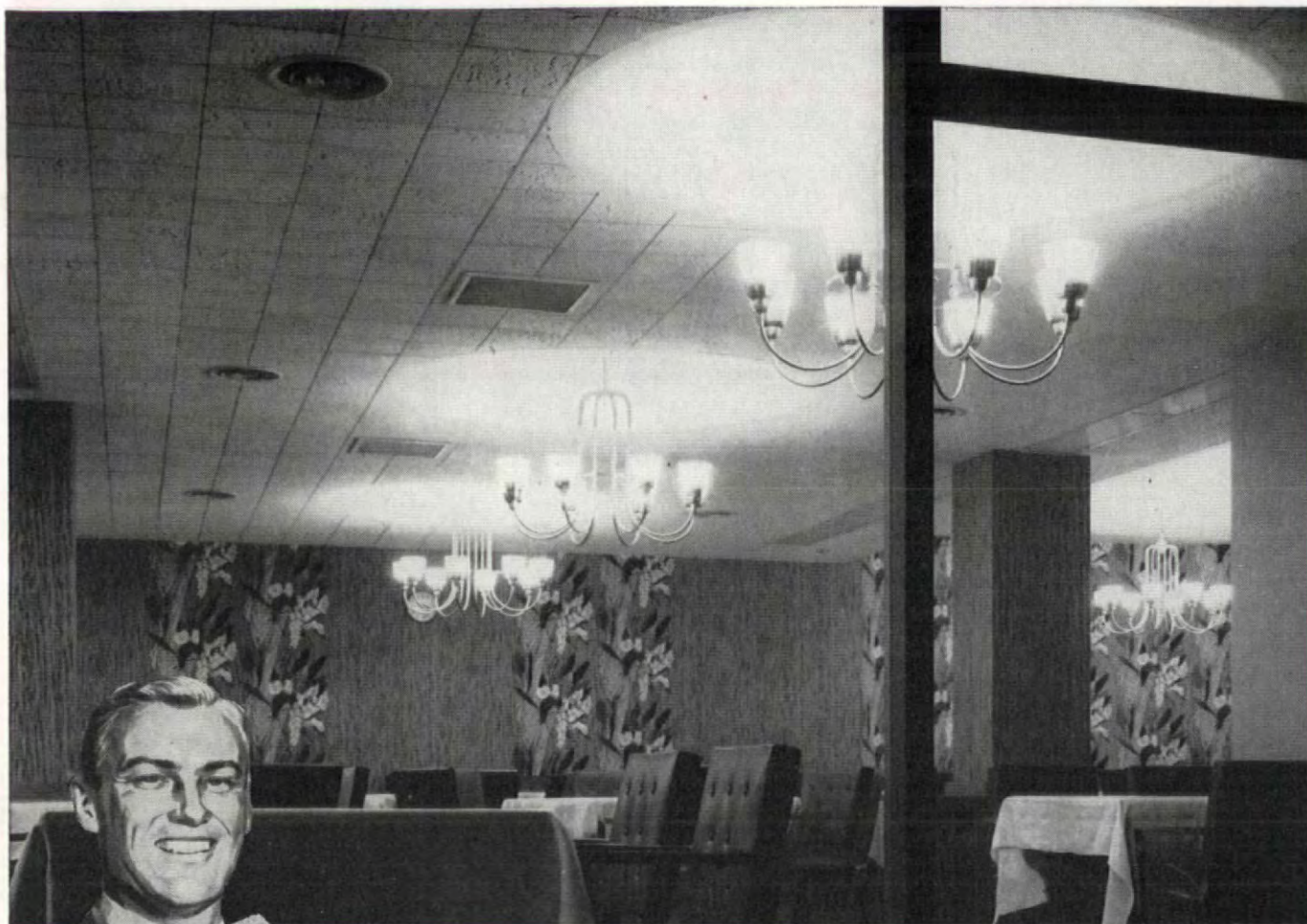
A Johns-Manville Permacoustic ceiling was selected for this staff dining room because of its striking textured effect, its non-combustibility and its superior sound-absorbing qualities.
