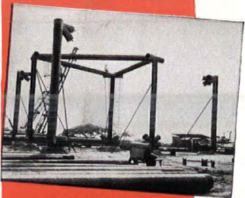
2. Closer view of the starting framework, showing 22" diameter steel pipe being used.
