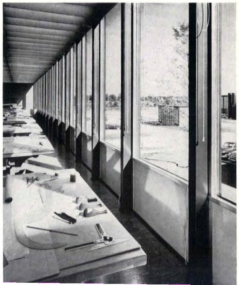
Structural columns match 5'-2" module of ceiling
