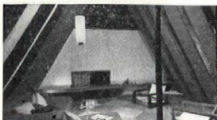
Full-scale week-end cabin by Campbell & Wong delighted art lovers with remarkable integration of sculpture, ceramics, interior decoration and landscaping. John Campbell and two associates built it in a week for $500. Rigid equilateral triangular 2 x 6's sheathed with waterproof wallboard form roof, spaced 2 x 3's the deck.
