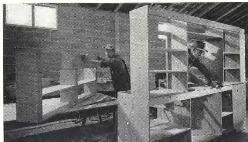
Workers at shop drill Finnish birch slab doors for hardware (above). Below, they pre-assemble kitchen cabinet units.
