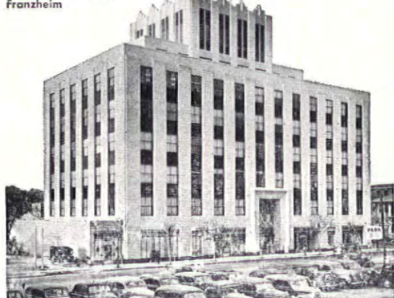
Spandrels of Alberene Serpentine. Continental Oil & Gas Building, Houston Texas. Architect — Kenneth Franzheim
