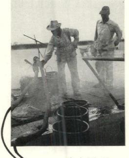
Gas-fired "kettle" or melting pot is still the basic supply of hot asphalt, but a two-way  $1\frac{1}{2}$ " pipe circulating system delivers 30 gals. of temperature-controlled material per minute to the roof. This circulating loop is connected by flextble couplings to both the supply and return level of the kettle and to drawoff cocks or valves just above the roof surface. Asphalt is then delivered by bucket on dollies to dispenser.
