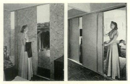
Sliding doors of pressed fibre board in 1950-51 house made closet construction cheaper, opened bedroom to living room.
