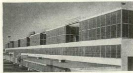
West elevation of The Glenn L. Martin Co's "B" building glazed Coolite, Heat Absorbing and Glare Reducing Glass.
