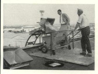
Delivery and application of the slag finish is continuous process, from dump truck to final surface, without stock piling or rehandling. Fed from a sluice gate on the rear of the elevated truck bed, the slag-skip travels on a fast, lightweight elevator which can hoist 9 tons or 4,500 sq. ft. of applied aggregate per hour, compared with  $2\frac{1}{2}$  tons or 1,125 sq. ft. by the old rope and bucket method.
