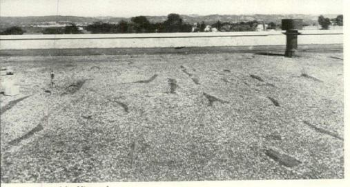
Typical buckling and erosion caused by blisters
