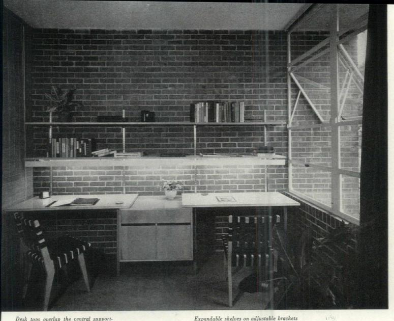
Desk tops overlap the central supporting cabinet to make a slip joint which allows for minor variations in spacing. Expandable shelves on adjustable brackets Light shelf eliminates lamp clutter
