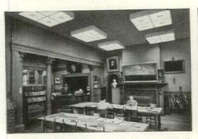
This high-intensity installation of surface-mounted SKYLIKE units was selected for the modernization of the Amesbury, Massachusetts Public Library. Note the low brightness levels at the light source . . . the 90° shielding . . . the absence of harsh shadows and sharp light cut-off lines.
