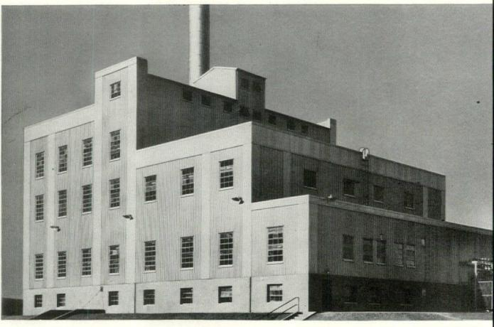
▲ 21,000 sq. ft. of Stainless Steel were used in the walls of this new power station built for the Northern States Power Company, Minot, N. D. Designed by Pioneer Service and Engineering Company, Chicago. Wall materials were fabricated and erected by The R. C. Mahon Company, Detroit, Michigan.
