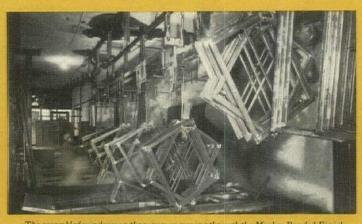
The assembled windows on the conveyor moving through the Mesker Bonded Finish tanks . . . degreased, cleaned, phosphate coated, dip painted, then oven dried.
