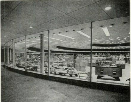
Jordan-Marsh has 150,000 sq. ft. under this dome and is building another 22,000 sq. ft. down the mall for furniture. Dome, 227' wide, is largest clear-span dome in U. S. Supported by 36 arched steel beams, it provides column-free first floor space. Store has split-level plan: mezzanines above first floor and basement create four selling levels.
