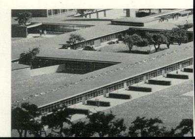
Besides providing a permanent, colorful exterior finish, these 2" thick panels are expected to 1) cost no more than an equivalent masonry wall, yet provide better insulation, 2) require a minimum of maintenance, 3) lower erection costs, 4) lighten the load on foundations—a special asset on this seaside site.
