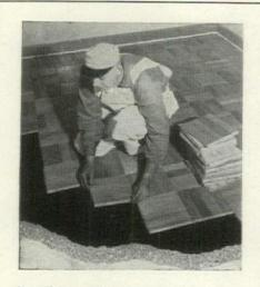
Install in mastic over concrete
