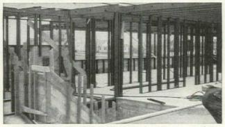
Interior view of Redfield (S.D.) hospital under construction. Stran-Steel framing comes pre-cut, pre-punched, treated with rust-inhibiting paint.
