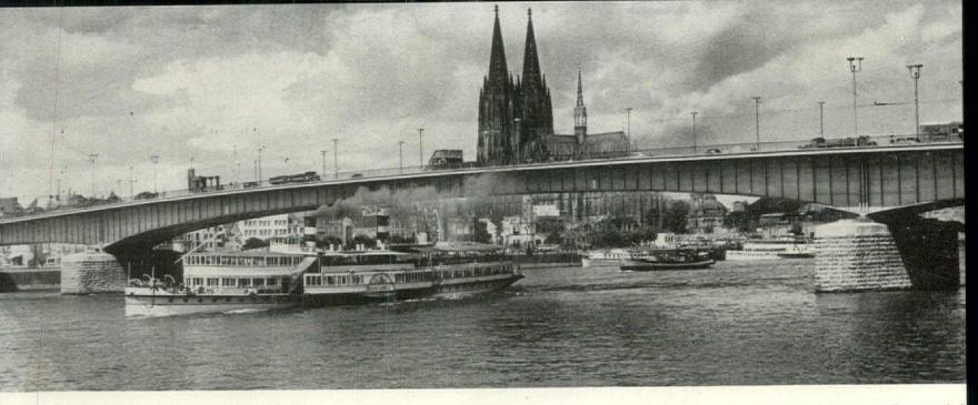
COLOGNE: Designed by Dr. Ing. F. Leonhardt, this new bridge across the Rhine is made up of a series of steel box girders, varied in depth to form shallow, paraboli
