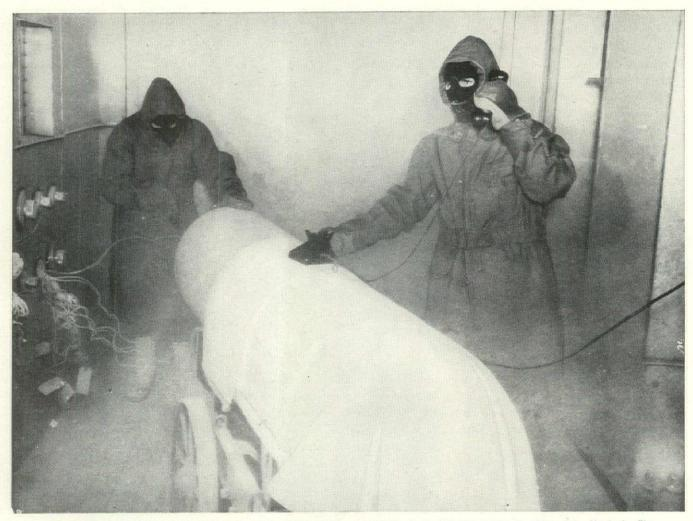
"We have to know that this new mine is going to do its job even after riding for hours under the belly of a plane or being stored long periods in sub-zero temperatures," said R. E. Hightower, chief of the Technical Evaluation Department, Naval Ordnance Laboratory, White Oak, Maryland. The desired temperature and humidity conditions are precisely provided by Worthington refrigeration. Contractor: Arthur E. Magher Co., N. Y., N. Y.
