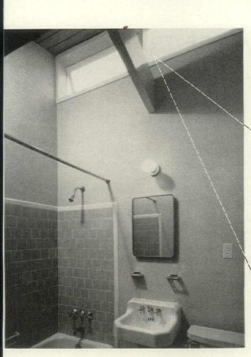
Grouping bath and kitchen equipment into a central service core saved on piping, made for a neat and efficient floor plan. Bathroom is well lighted and ventilated by clerestory window; "inside" placement gives complete privacy, saves out side wall and window space for the living rooms.
