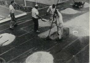
**OLD WAY** used many mops, many shovels, many buckets. Raw material was cooked on ground, hoisted up to roof (buckets were lifted one to a rope) and placed slowly.
