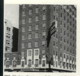
TEST: Glaring, direct rays of the sun made west rooms of Tulsa's Alvin Hotel uncomfortable, caused requests for space changes. Kaiser Aluminum Shade Screening was tested for a full summer on a few west windows and proved it blocked the sun without blocking light and air.
