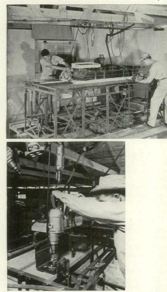
Heavy weight, raised and lowered by hand lever, holds door firmly in place. All power tools needed are hung from overhead racks. Fixtures, such as the drill jig, make errors almost an impossibility if workman lines up door properly. One man can square four edges, drill for hardware, rout for hinges and install hinges in seven minutes.
