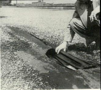
14 lbs. per sq. ft. of upward pressure are needed to separate the plies of a built-up roof, but there is no measure of the shearing effect of blisters between plies. Above, the scars which blisters leave.
