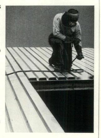
**DESCRIPTION**—Granco Steel Roof Deck has longitudinal ribs 1%" deep spaced on 5%" centers and is available in 18, 20 or 22 gage. The ribs are flared at one end permitting proper nesting at end laps. Granco Steel Roof Deck has a wide cover width of 28%" with a maximum sheet length of 14' 4". Positive attachment obtained by welding.
