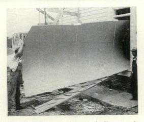
Easily bent through a doorway, the Upson panels (precut to size) are secured to the studs and ceiling joists without any visible fasteners.
