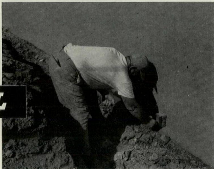
Al Loreti applies 2 coats of Thoroseal to concrete block foundation, as sure protection against rain and dampness.
