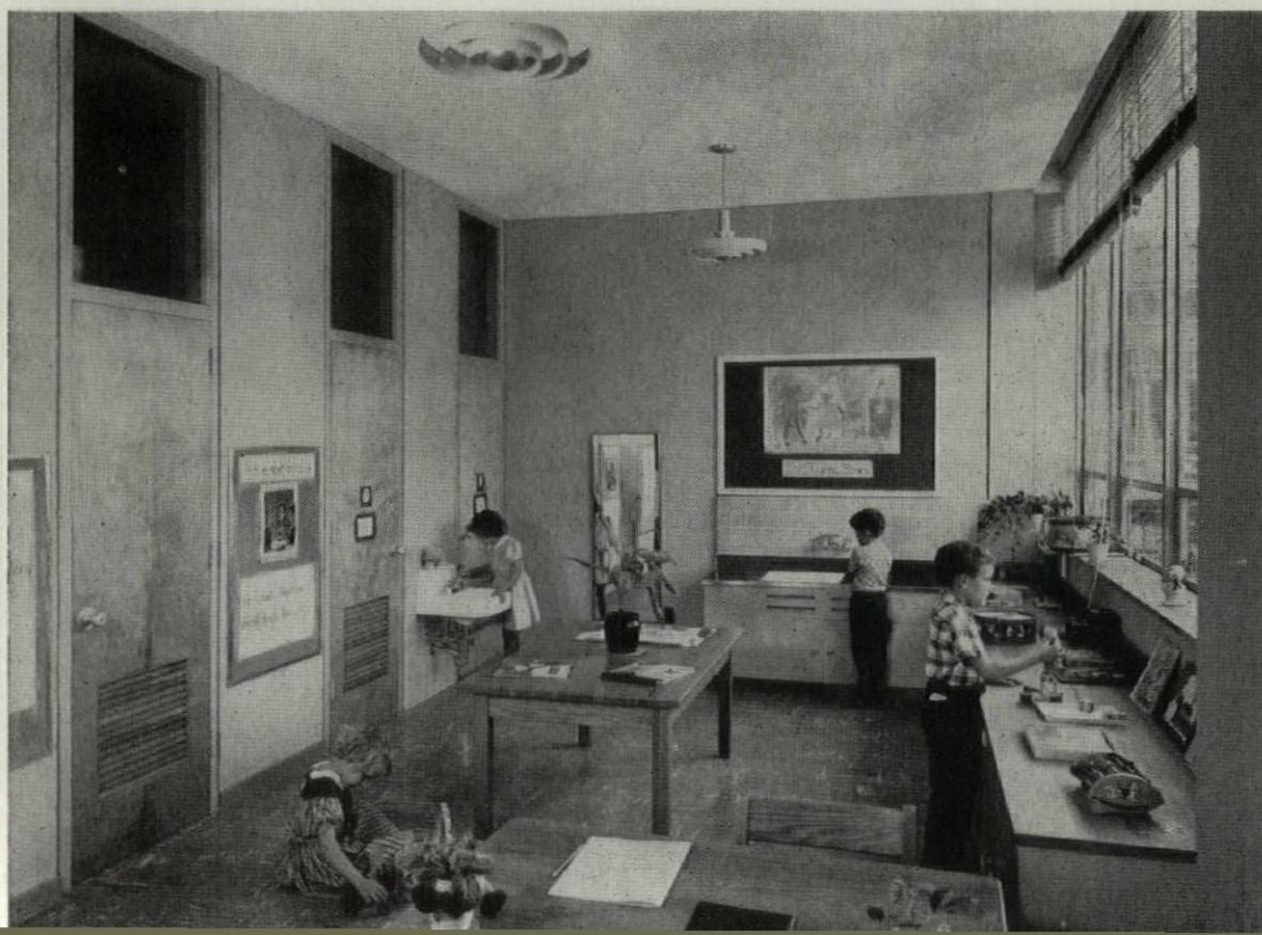
Continuous sill-to-ceiling windows give youngsters a sense of freedom and space in L-shaped primary classrooms, but require teacher-regulation of blinds for light control. Work alcove in arm of L (below) combines sinks, counters, storage space and toilets in compact unit. Note big glass panels which light interior spaces, prevent fear of confinement.
