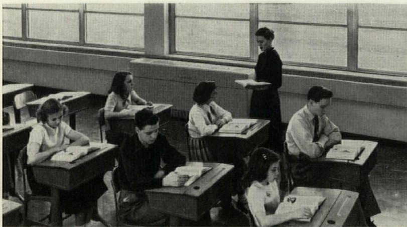
Showing the Nesbitt Syncretizer with Wind-o-line Radiation extending from both ends of the ventilating unit—positive protection against window downdraft.
