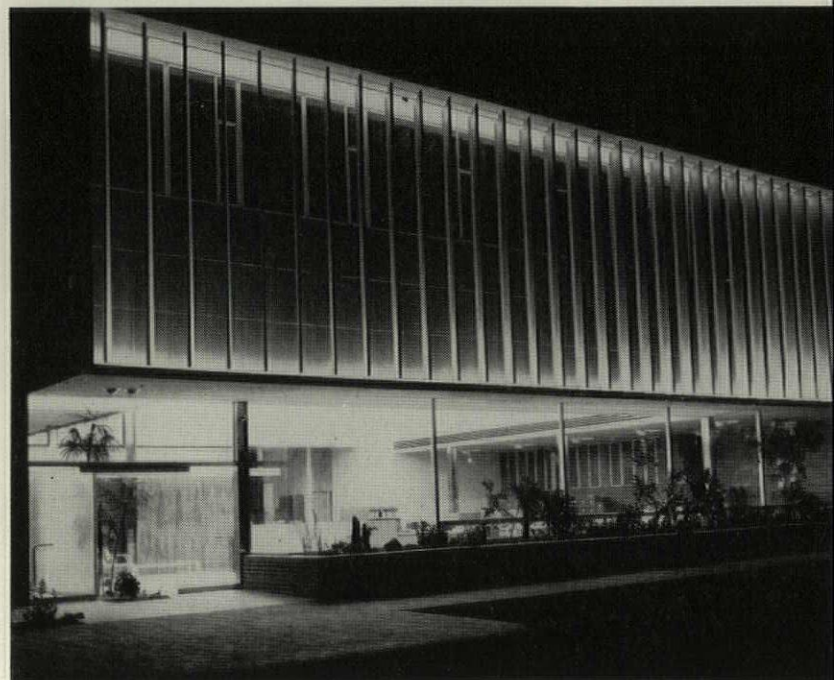
Egg-crate trough in acoustical tile ceiling (above and continuing into the hall, left) lights reception-display room of second floor tenants. After dark (below) fluorescent lights silhouette vertical aluminum louvers—the main exterior design feature.
