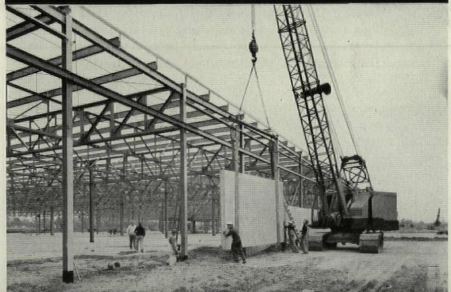
Steel columns are on 20' centers; this sets length of panel. Heavy belt slings are placed around panels for crane pickup.
