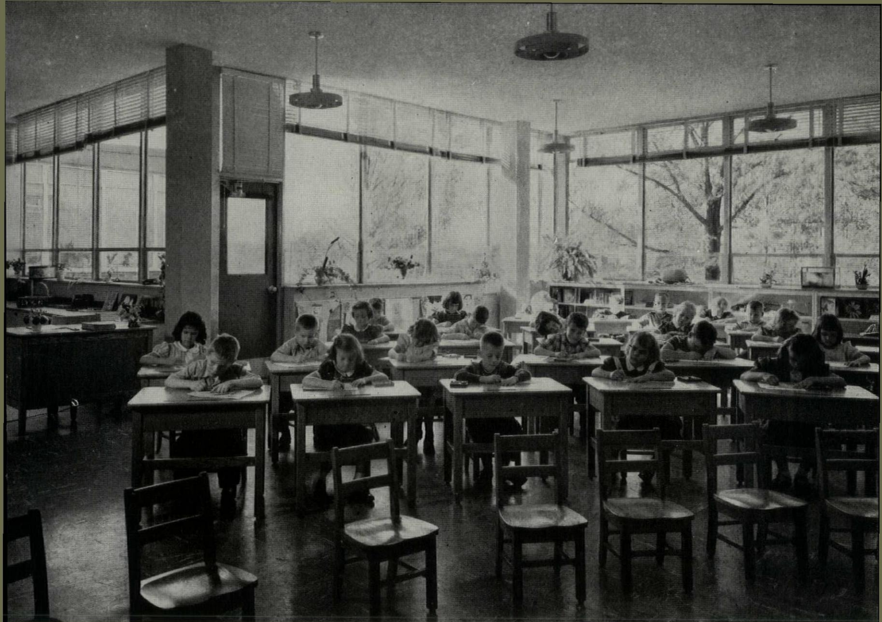
Continuous sill-to-ceiling windows give youngsters a sense of freedom and space in L-shaped primary classrooms, but require teacher-regulation of blinds for light control. Work alcove in arm of L (below) combines sinks, counters, storage space and toilets in compact unit. Note big glass panels which light interior spaces, prevent fear of confinement.
