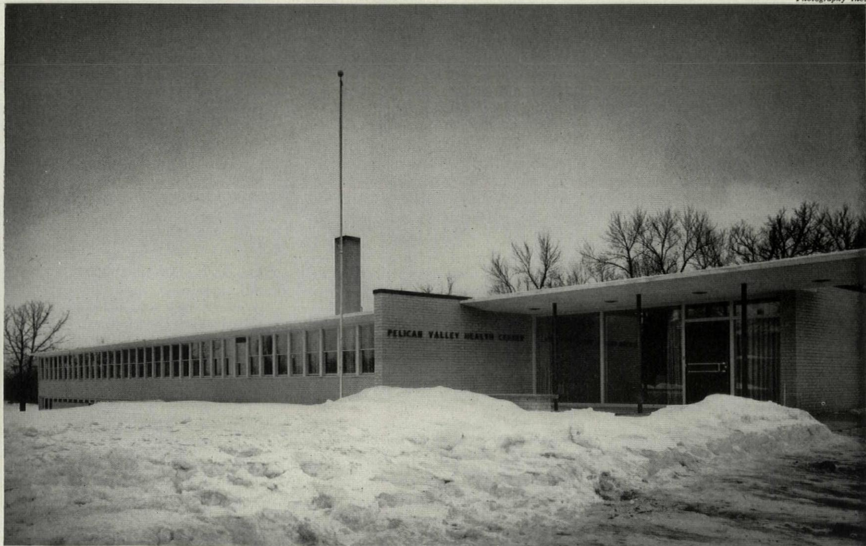
Main entry (left and above) is shielded by a neatly detailed concrete canopy with lally column supports, has a vestibule for weather protection.
