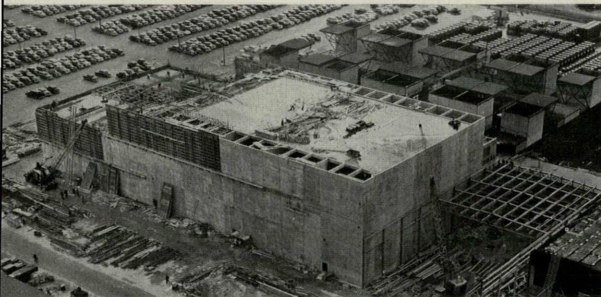
Pratt & Whitney's new test cells are designed for both piston and new jet engines
