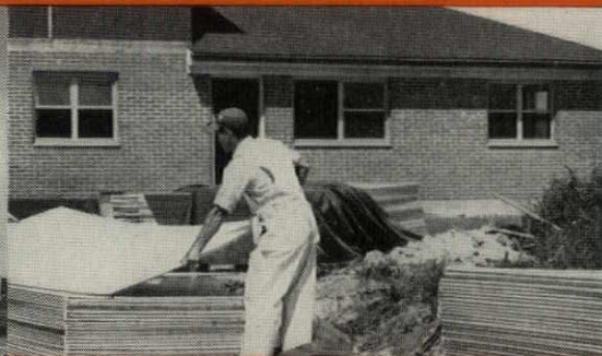
400,000 sq. ft. of \frac{1}{2} " FIRESTOP BESTWALL will be applied on all party walls and ceilings and the stair wells.
