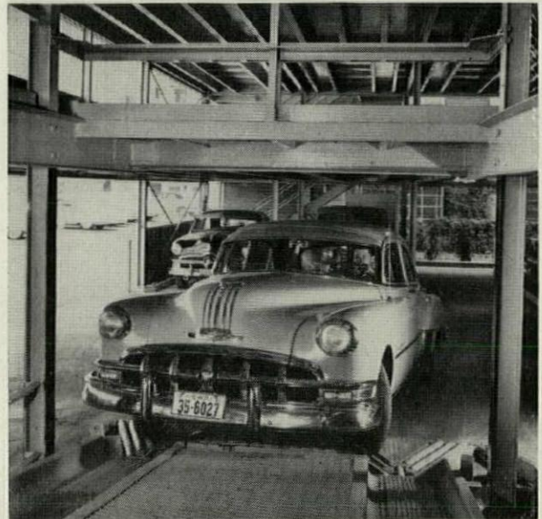
Ramps are prefabricated of a pair of 16" wide steel troughs to take car wheels, separated by light-gauge sheet steel. Drivers are assisted in "finding" wheel troughs by a bed of converging rollers actuated by the forward motion of the car, providing safer operation and a shorter turning radius.
