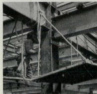
Fig. 2. Detail of Girder running through column. Column top and base are welded to beam flange. Vertical stiffeners provide continuity to column.
