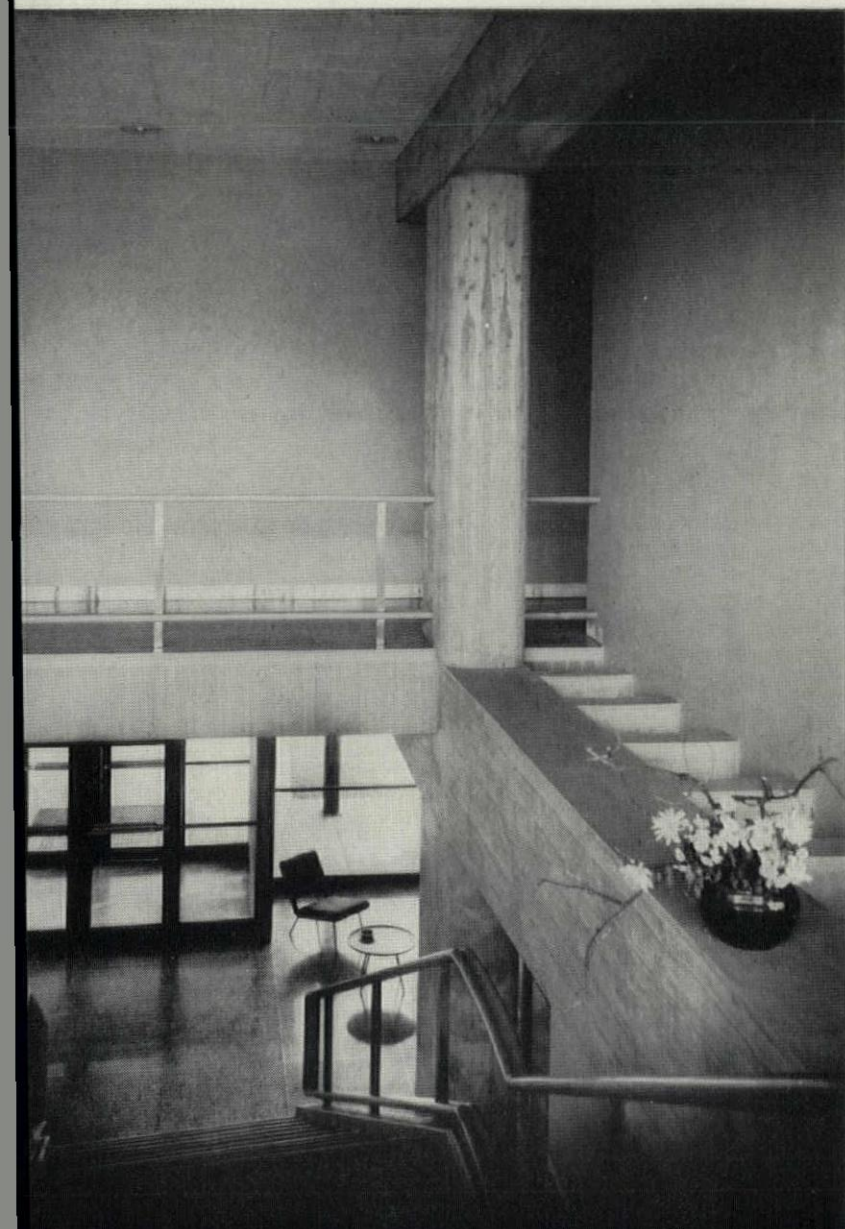
North wall is outside of posts; no louvers needed. Shoji ply panels act as doors. Finned radiator in jacket on floor prevents down draft next to glass.
