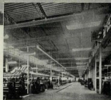
Ceco Steel Joists are practical as purlins in roofs of one story factories and plants.
