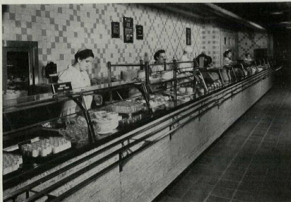
A pioneer stainless installation—not a new one! These are recent photographs of equipment made entirely of Type 430 Stainless Steel, installed in a Montreal cafeteria in 1927.
