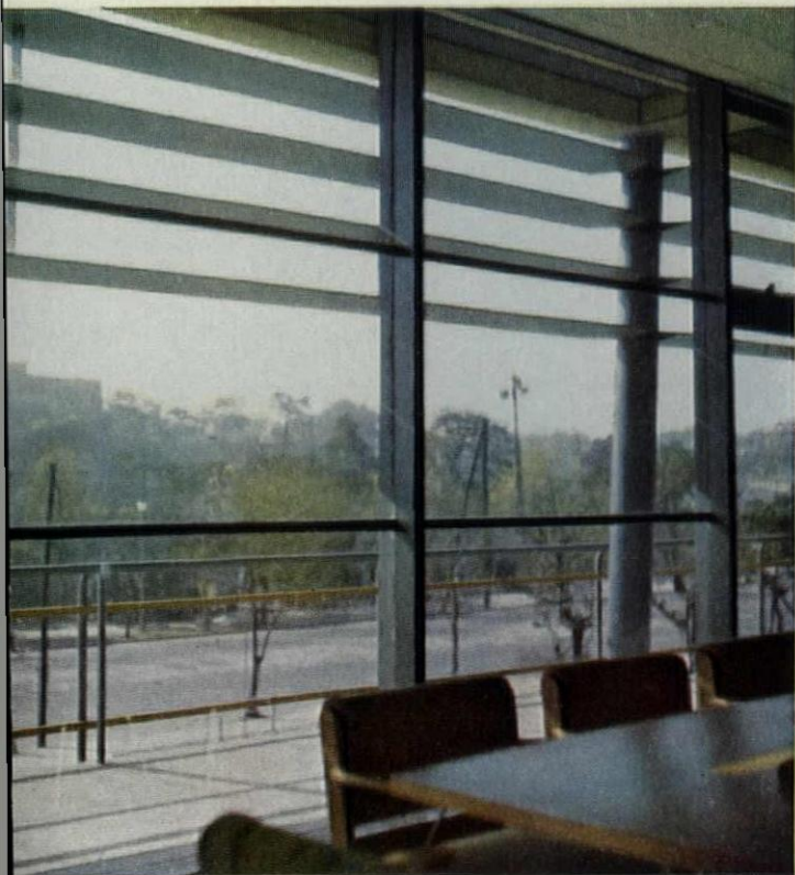
South side posts are outside wall; louvers are for shading
