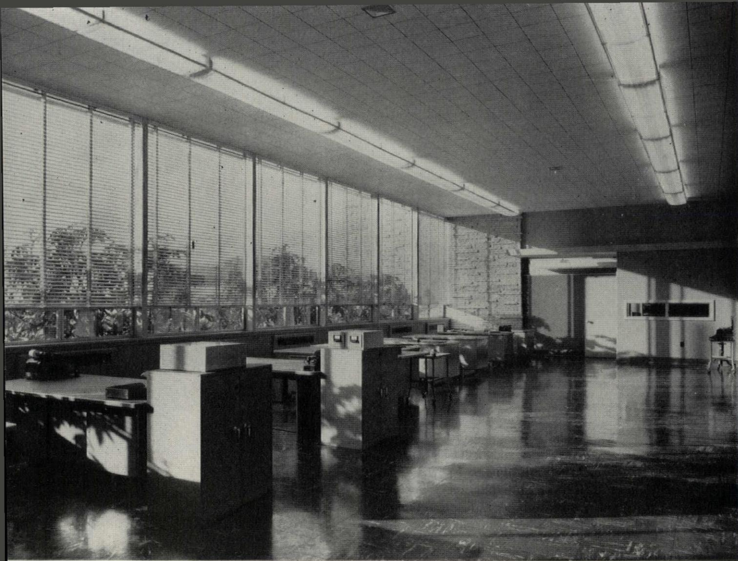
Sun control in general office area is accomplished with aluminum Venetian blinds. Though building has main exposures to east and west, latitude of Seattle makes this unusual orientation most advantageous. Note stone wall carried into far end of room, lush planting just outside.
