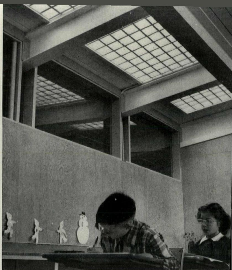
Strip skylights with wooden egg-crate louvers supplement light from classroom windows. Glass-topped classroom partitions bring daylight into corridor.
