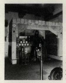
**Precast concrete frames** (left) afford most protection but ¾" steel roofing (above) can be used where there is danger of floors being overloaded. After a direct hit (right) machinery so protected remained undamaged.
