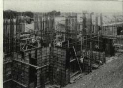
LARGE, LIGHTWEIGHT CONCRETE FORMS OF GPX CAN EASILY BE HANDLED BY ONE MAN FOR COKE PLANT BIN AND BATTERY FOUN-DATION PREPARATION. GPX is an extremely high-grade, solid core exterior Douglas Fir Plywood with a superior plastic overlay applied under heat and pressure when the veneer layers are being molded, becoming a part of the plywood itself.
