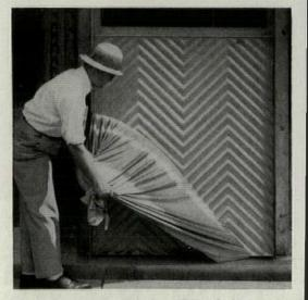
STAINLESS STEEL spandrels-3300 of them-were fabricated with Stainless window frames, windows and fins to form complete assemblies. A temporary plastic coating protected the span-drels during shipment and erection and was peeled off after installation.
