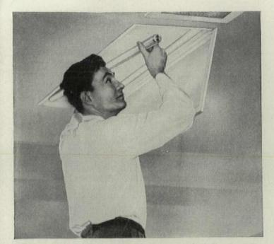
With the 277-volt lighting system, you use standard fluorescent fixtures, standard lamps. Just specify 240-280-volt ballasts.
