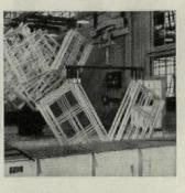
GALVANIZING. Assemblies dip deep into molten zinc, and come up with a thick, smooth, uniform coating. Temperature and timing are automatically controlled with laboratory accuracy.
