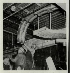
CELLULAR STEEL FLOORS carry electrical and telephone cables that can be tapped at almost any exposed point. In addition, light fixtures, airconditioning ducts, acoustical blocks and even ceilings themselves are suspended from this cellular flooring.
