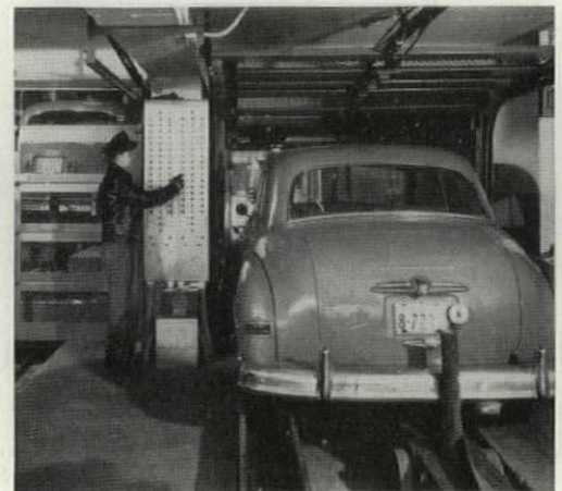
TWO ELEVATORS handle cars on a "positioner" push-button principle evolved by inventor Richard Sinclair after watching the expandable knobbed sizer with which his wife was being fitted for new shoes. Attendant only pushes buttons, positioner and elevator do the rest.
