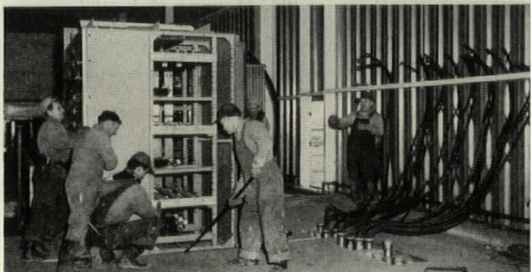
EQUIPMENT ARRIVES in unit form ready for fast installation to conserve skilled manpower. Here, switchgear section of a load-center unit substation is moved into position in penthouse on roof.
