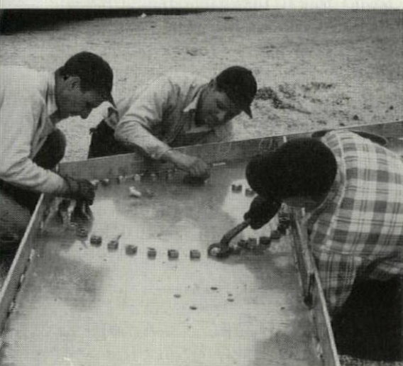
"Sunburst" bolted splice being made at knee joint of structural frames. Made in the web to avoid weakening flange plates, the wide diameter circle of bolts produces the maximum strength for the smallest number of bolts with equal stress distribution between individual bolts.
