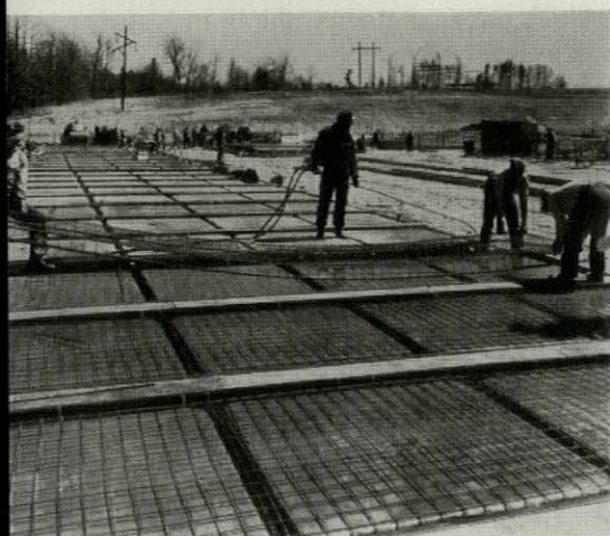
Ribbed roof panels, 22' x 5'-3" and weighing 1½ tons, are also precast. Picture above shows prefabricated wire mesh reinforcing being positioned in the molds.
