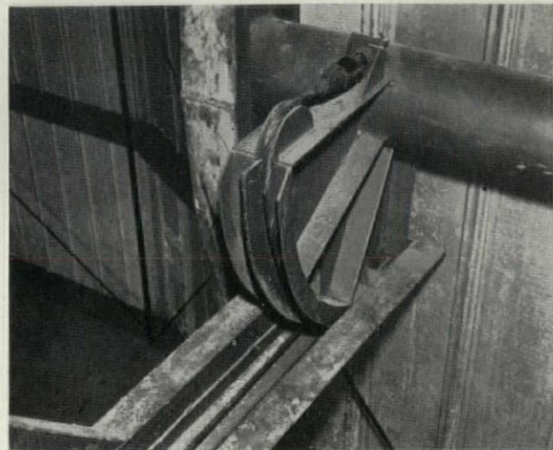
Closeup of one of the supporting quadrant wheels on which the door rotates.
