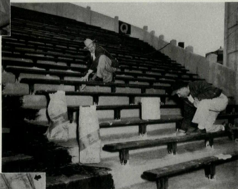
Above photograph shows THOROSEAL FOUNDATION COATING being grouted into upper, or wearing, surface of bleacher seats.
