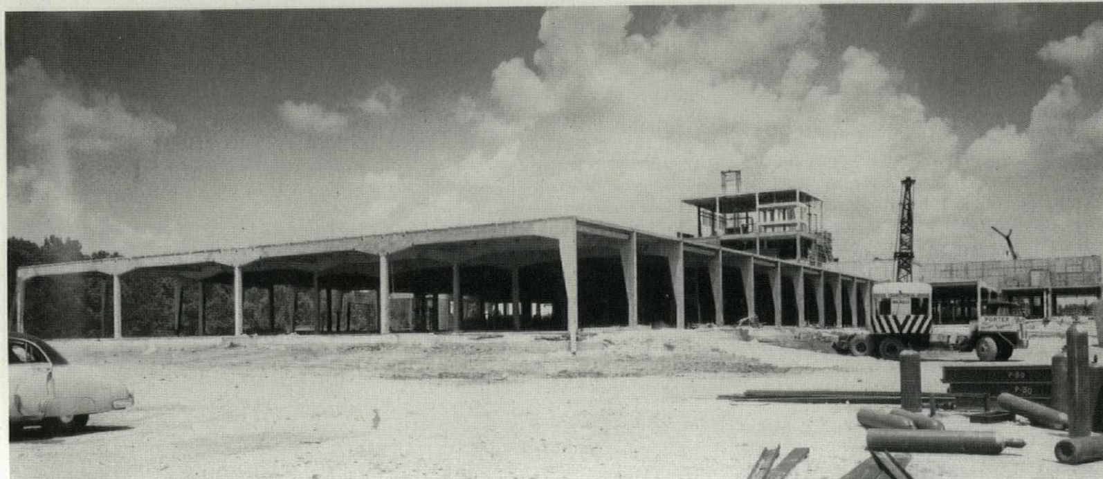
Precast warehouse frame before wall panels were erected.
