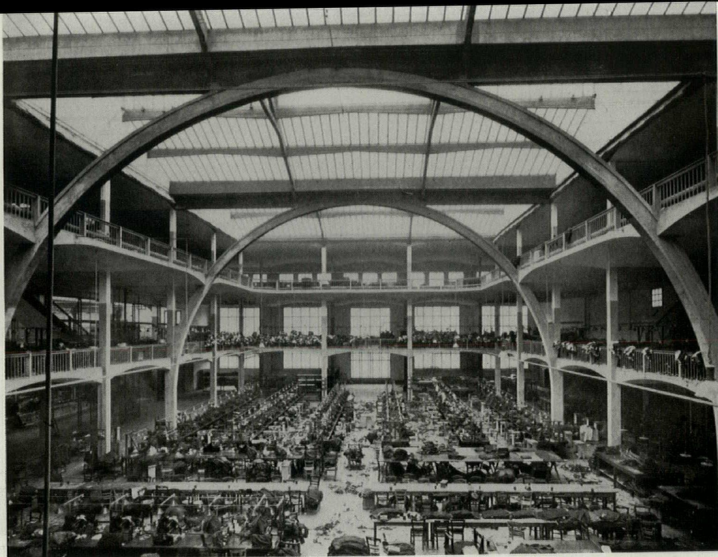
Perret factory in Paris shows light, wide-spanning reinforced concrete arches
