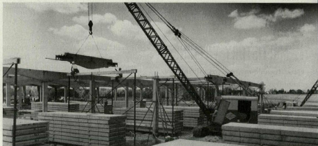
Precast hollow box-section header being hoisted into position atop a column supported by light falsework. Greatest depth of header is 3'-6" at column; it is 18' long and weighs three tons.
