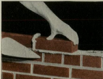
The brick should then be pushed into place.
