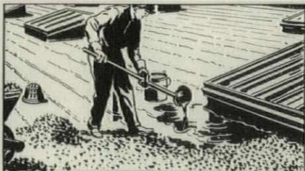
The famous Barrett Armored Surface of a triple-thick coating of pitch plus a top layer of gravel or slag assures extra protection against mechanical damage and fire.
