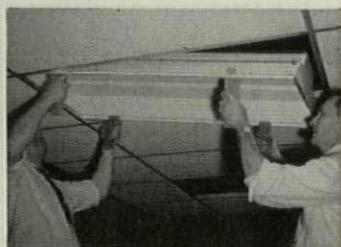
Easy to install. Simply compress the sides of the fixture and insert into grid opening.
