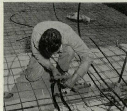
Unlike copper, *Therma-Koil* requires no heat for joints; mechanical fittings are employed.
