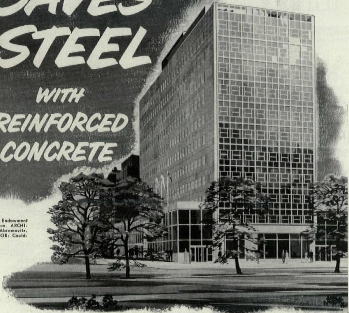
In this impressive Manhattan structure, planned for the use of nonprofit organizations active in promoting international understanding, reinforced concrete was chosen for framing and floors . . . in order to *save steel* for national defense.
