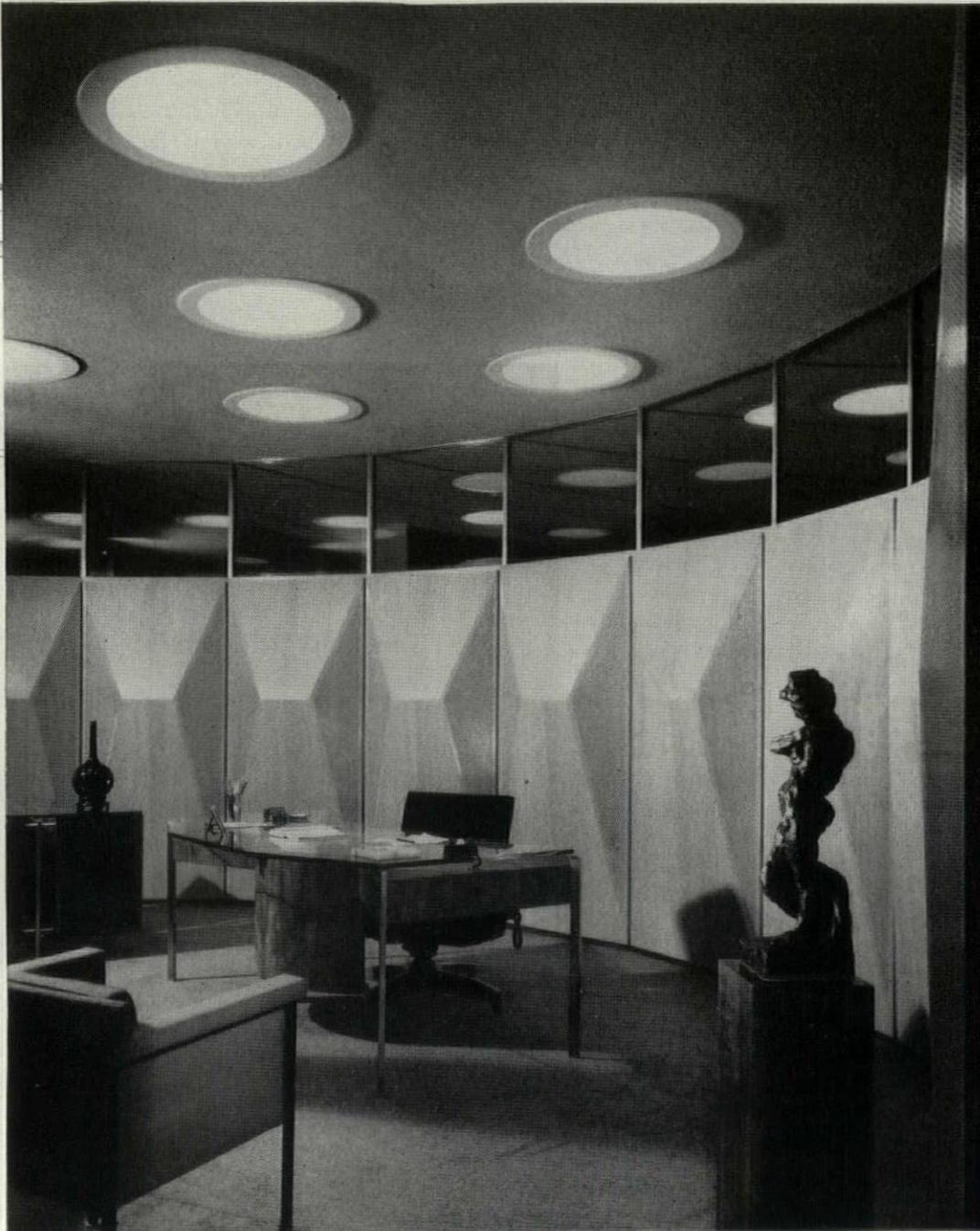
Photo (r) shows wall of faceted panels, outer wall surface of teakwood. Photo below shows perforations in side splays of panels. Horizontal section shows construction of round wall, and vertical section, how sound deflects from panels.
