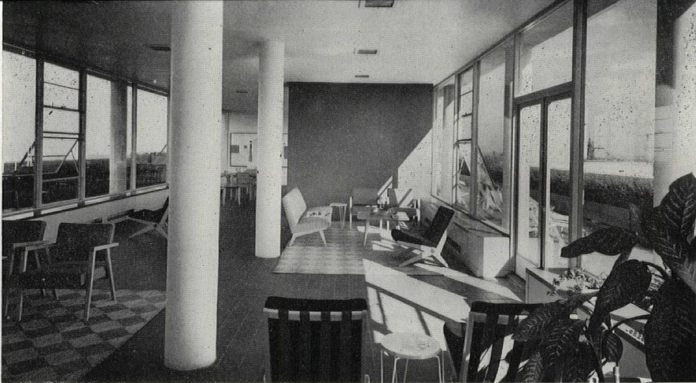
Top floor of Manhattan House is a set of spacious communal solaria and terraces, available for all tenants. Notice how the reinforced concrete columns here have slimmed down in their growth up from the first floor.
