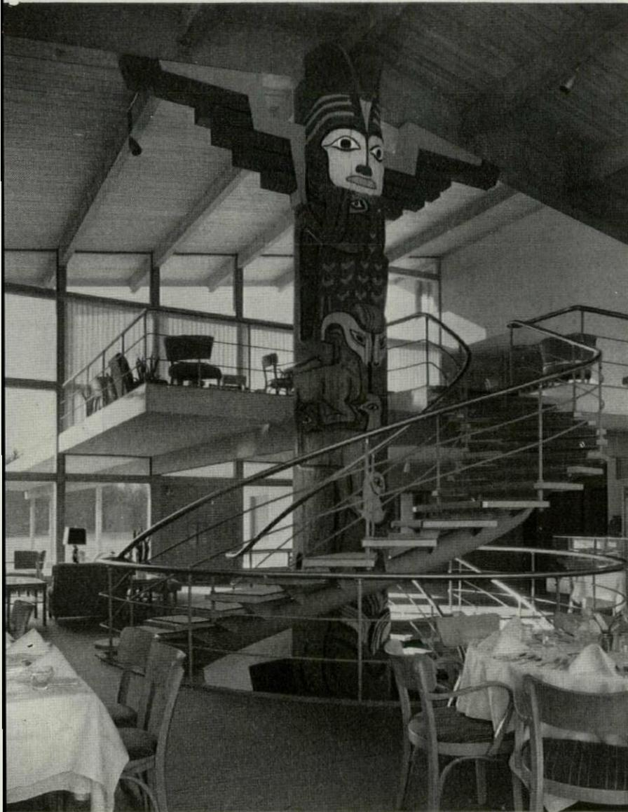
Stairway around structural totem pole is self-supporting on a formed spine of 8" steel pipe. Open carpeted treads of 1½" plywood are bolted to steel angle supports welded to the pipe.
