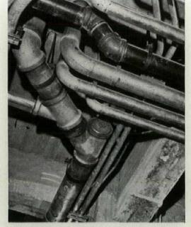
Aluminum pipes constitute about 60% of all piping in Alcoa building, Galvanized pipes here handle waste water, Black steel pipe carries steam condensate.
