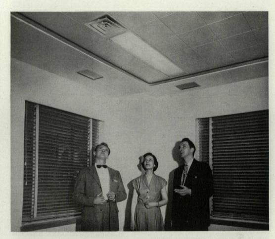
In Alcoa building heating and cooling with radiant panels is supplemented by air supplied through ceiling diffusers strategically spotted in ceiling. Return air is pulled back through rectangular grilles around perimeter of the ceiling.
