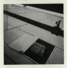
View through ceiling shows how edges of the flexible corrugated plastic are held between ¾"-wide aluminum extrusions above and 1-¼"-wide translucent plastic extrusions below. Occasional incandescent bulbs are nightlights. Photo below shows how ceiling merges into wall at rear.
