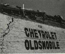
S-SHAPED FLANGES (arrow). One end of anchor bolts kept roof atop this quake-wracked brick wall, said building inspectors.
