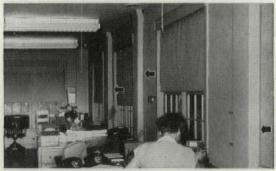
In the general office three ducts on outside walls descend to within a few inches of the floor, introducing warm air where most needed.
