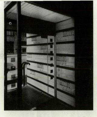
Low entrance ceiling is lighted by fluorescent strips over corrugated plastic. For extra height in the selling area, second floor was removed in favor of a ceiling hung from third floor (see section below). Balcony marks off the separate department for packaged ice cream, emphasizes spaciousness and gives a setting for the main interior sign.
