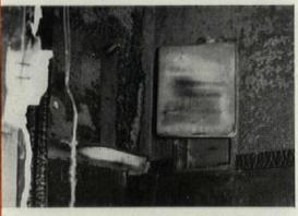
Nowhere has fire broken through the wall, although the tile panels are blistered.
