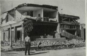
JUANITA HOTEL, where one man was killed, was rated as completely destroyed as was building at right. Construction: unreinforced brick.
