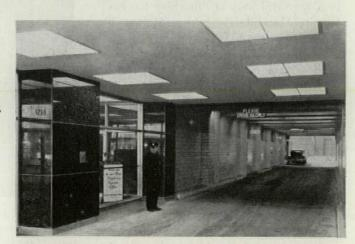
Illustration shows drive-in automobile area (banking) lighted with Garcy Slimline fixtures No. 7449-2 (background) with two 96' 430 ma. lamps, and Garcy No. 7895 4' x 4' square fixtures (foreground), providing high light intensity for effective lighting of drive-in banking area.
