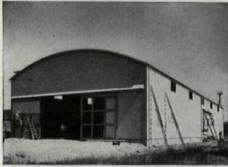
With unlimited choice of building materials, Rusdick Lumber Sales chose plywood siding for its new Tacoma, Wash. warehouse and the builder reports the panels cut construction costs by \$10 per square. "We chose plywood because we like a smooth, flush exterior surface but cost was an important factor and plywood was cheaper" says partsowner Russell Ross.
