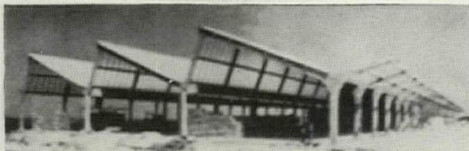
Light steel frames (left) developed by Mopin Co., England, are welded into eight-story units on the ground and hoisted into position where they receive additional rigidity from wall panels in the finished building. Precast concrete frames (above) show promise where repetition can bring down unit costs as in this north light factory.
