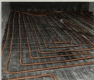
HEAT USED —Shown here is part of the 500 feet of copper coil embedded in concrete slabs in the floor of adjacent plant offices and other areas. This tubing circulates the refrigerant gas to furnish radiant heat.
