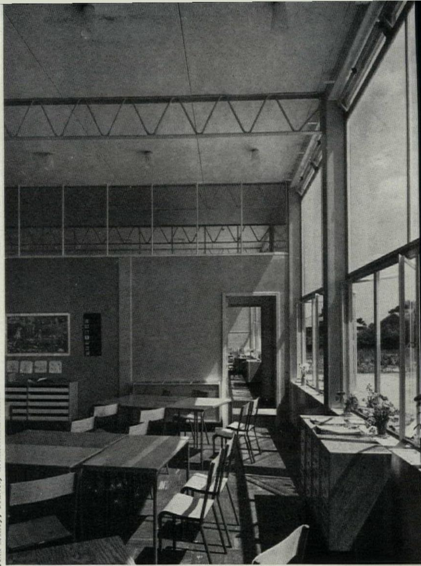
Interior of typical Hertfordshire classroom. Note exposed open-web joists. Glass-topped interior partitions are light, insulated panels. Plainness of finish is alleviated by bright paint.
