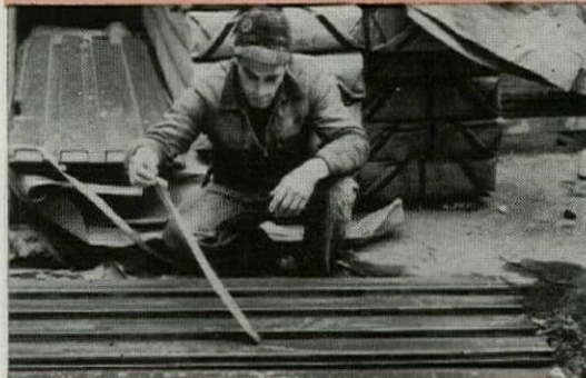
PROTECTIVE PAPER covering that kept the panels completely damage-free during fabrication and shipment is removed with a commercial preparation.
