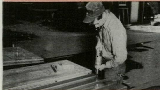
ON THE GROUND , panels are drilled for bolts which are used in erection. Two holes are positioned at the top and two at the bottom of each panel.
