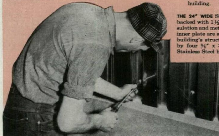
ON THE GROUND , panels are drilled for bolts which are used in erection. Two holes are positioned at the top and two at the bottom of each panel.
