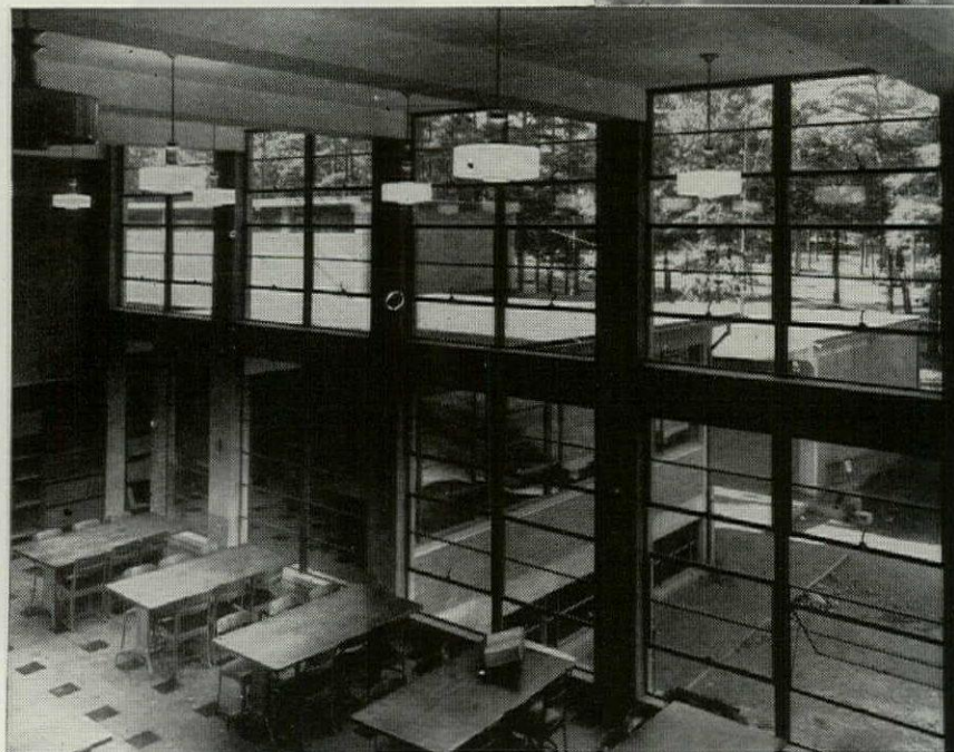
THERMOPANE* insulating glass Daylight Wall in the north Swanson Associates specified Thermopane insulating glass for Daylight Walls in the Birmingham (Mich.) High School to conserve heat and eliminate a cold zone near windows.
