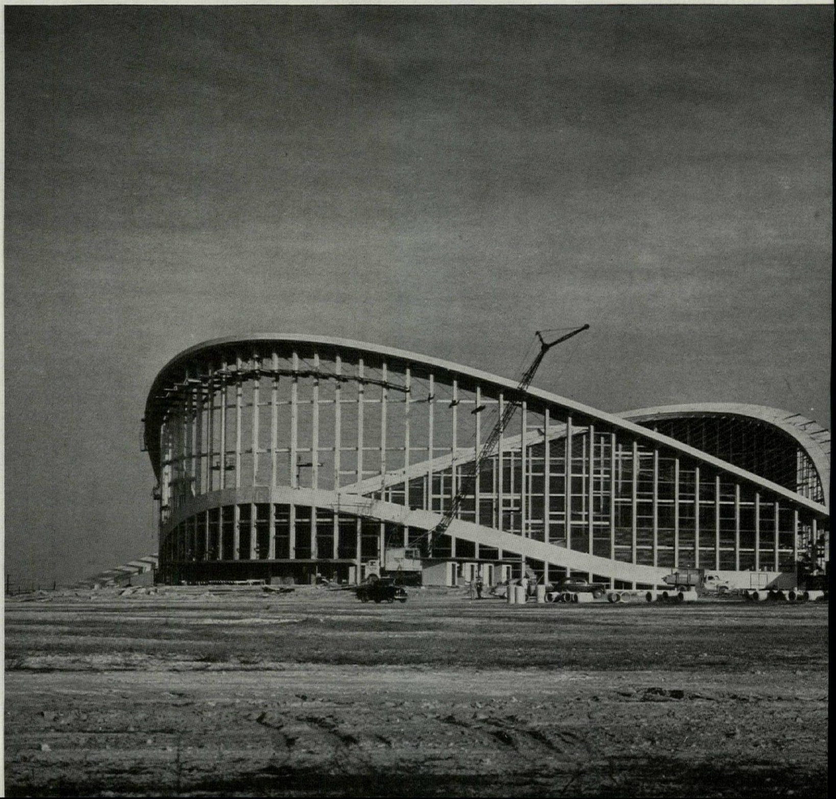
Scheme 1: Nowicki's original conception: few columns, two arches in compression carrying a suspended roof in tension.
