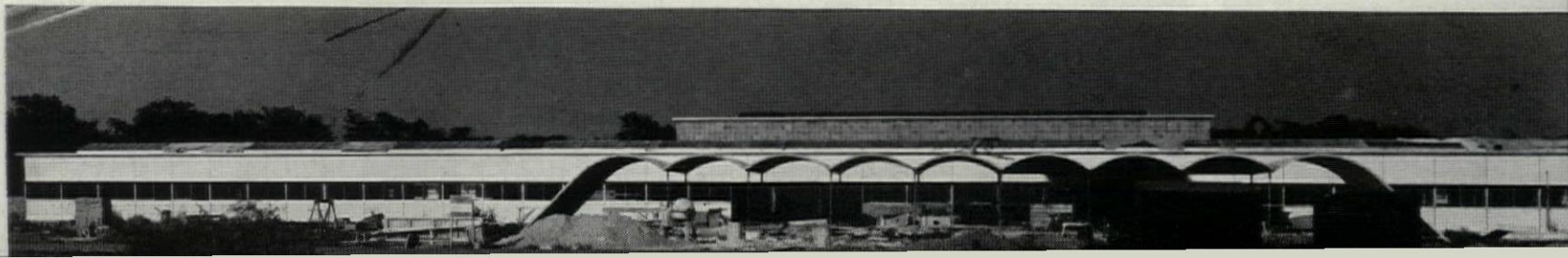
Playful "roller coaster" concrete canopy offsets regimented facade. End slopes of 45°—too steep to climb—shelter bicycle racks
