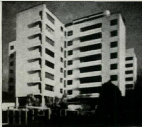
This 232' span timber truss in the US (left) is made possible by lamination and new jointing techniques. Concrete box-frame construction (above) used in a London apartment building by engineer Ove Arup, simplifies formwork by the elimination of columns. It is monolithic.
