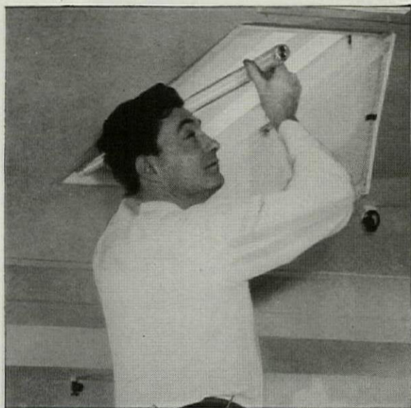
Standard lighting fixtures of any make are used with 277-volt lighting. Simply specify 240-280 volt ballasts. Lamps are the same.
