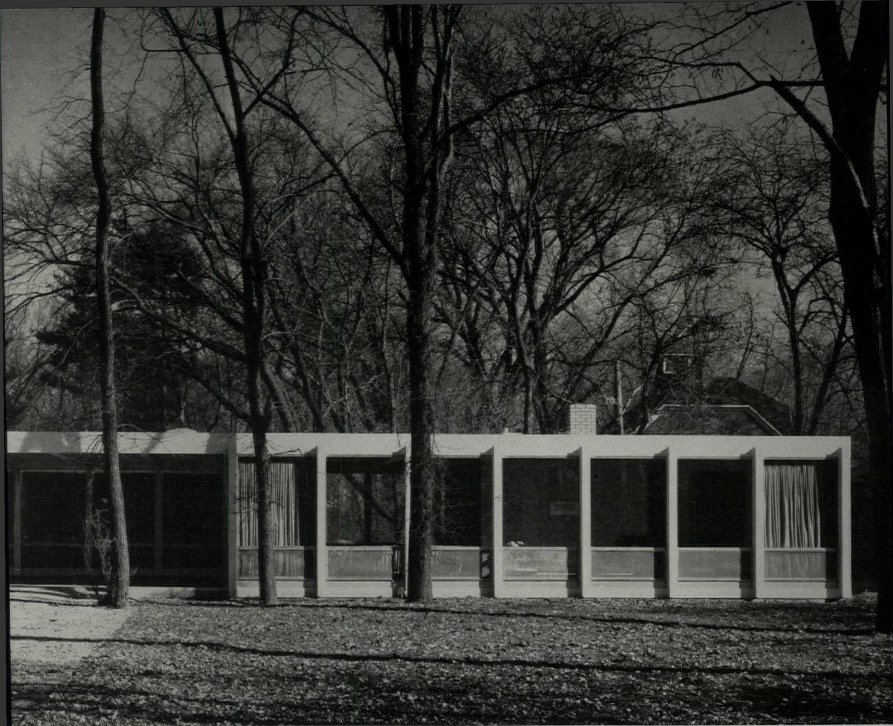
McCormick house is an assembly of two row houses, a prototype for production. Steel wall frames were shop assembled and welded.
