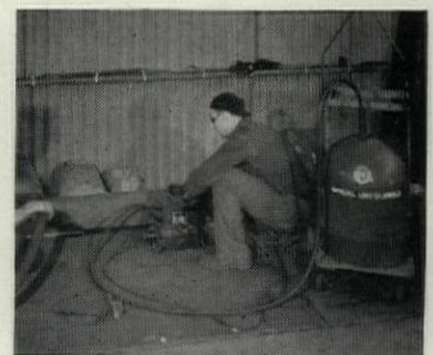
Fig. 2—Speeds Welding—Webs and flanges are fillet welded with "Manual Lincolnweld" at speeds of 26 to 30 inches per minute. Average time to fillet weld one side of 71 foot rafter is 90 minutes.
