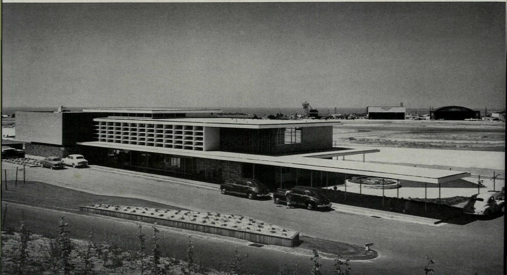
Extended canopies, eggcrate louvers on south side of terminal shield interior from southern sun
