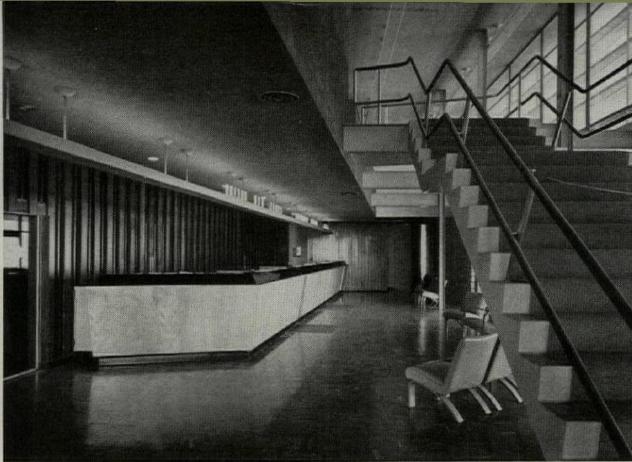
Screen wall of vertical louvers behind counters permits agents to spot approaching passengers through operations offices behind wall.
