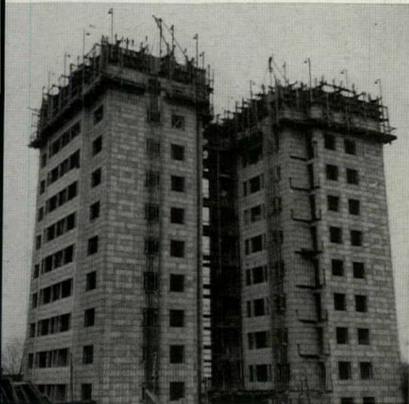
Sixteen-story apartments in Copenhagen were built by moving form construction. Outer walls consist of lightweight insulating blocks placed as the forms move up and backed by reinforcing and cast-in-place concrete.
