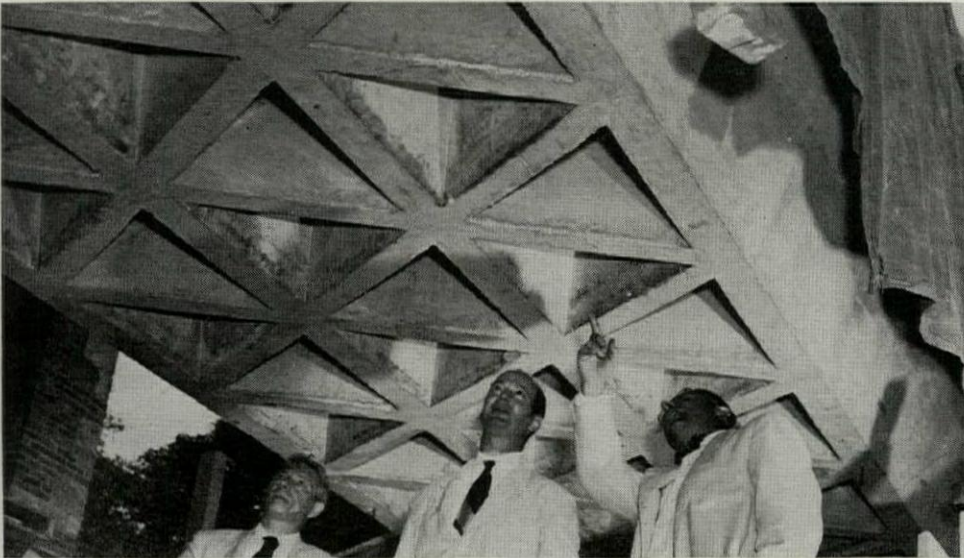
Sloping hollow pyramids of underside of ceiling conceal ducts and lighting gear . . .
