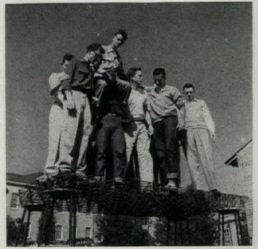
Buckminster Fuller's 4' x 10' tubular steel truss supports 11 husky students.
