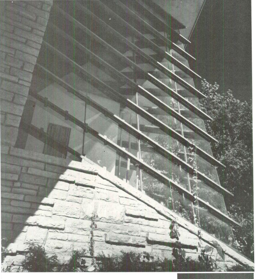
A LAST, CLOSE LOOK AT THE PROW. GLASS ENCLOSING THE APEX IS HELD BETWEEN 2" x 12" LOUVERS AND IS PLACED AT 25% SLANT TO SHUT OUT GLARE
