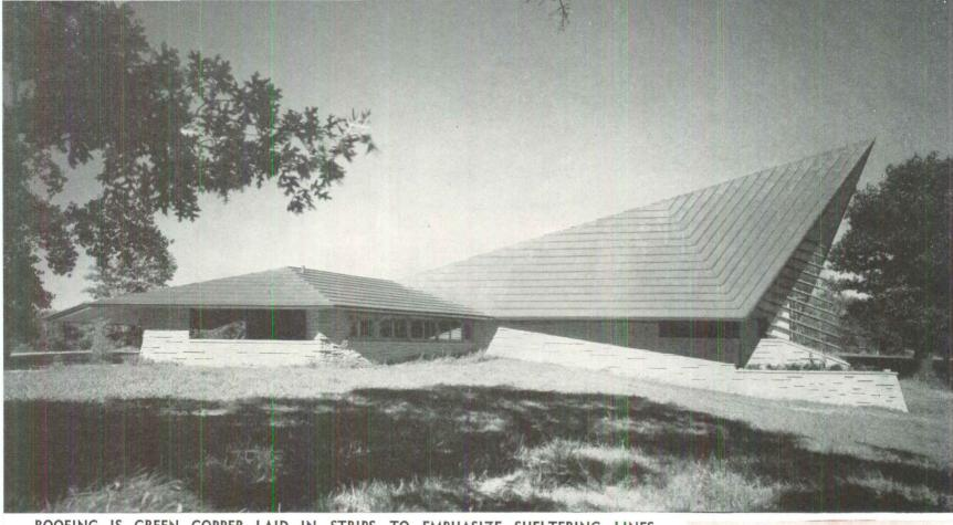
ROOFING IS GREEN COPPER LAID IN STRIPS TO EMPHASIZE SHELTERING LINES
