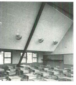
Economical tent construction gives lighting bonus: toplight through north roof slope of each classroom. Foot-candle and foot-lambert readings are almost identical in two wings. Concentric fixtures on slant work well. Side windows provide ventilation; heating is hot water radiant in floor panels.
