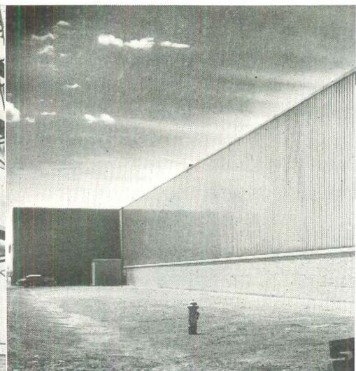
Twenty-five foot, inner (Ferroboard) panels fit on studs fastened to girts at sill line and parallel to top and bottom chord of trusses. Fourth girt, carry additional row of studs is arc welded to inner panels.
