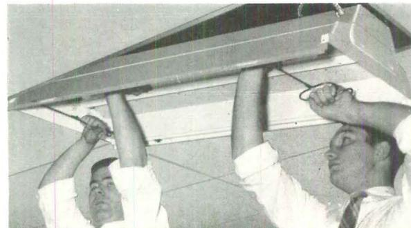
Mobilex is easy to install. Simply compress the sides of the fixture with "Mobilhooks" and insert it into the grid opening.
