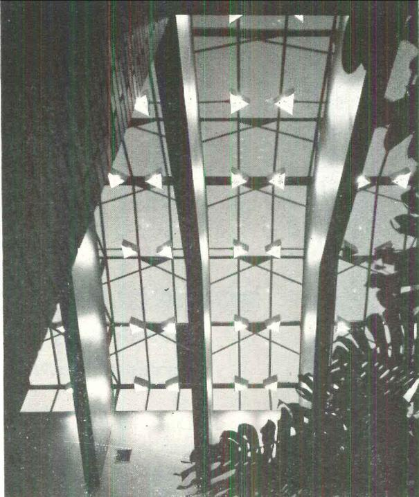
At night, the chancel's skylight effect is maintained with system of reflectors and incandescent lamps.
