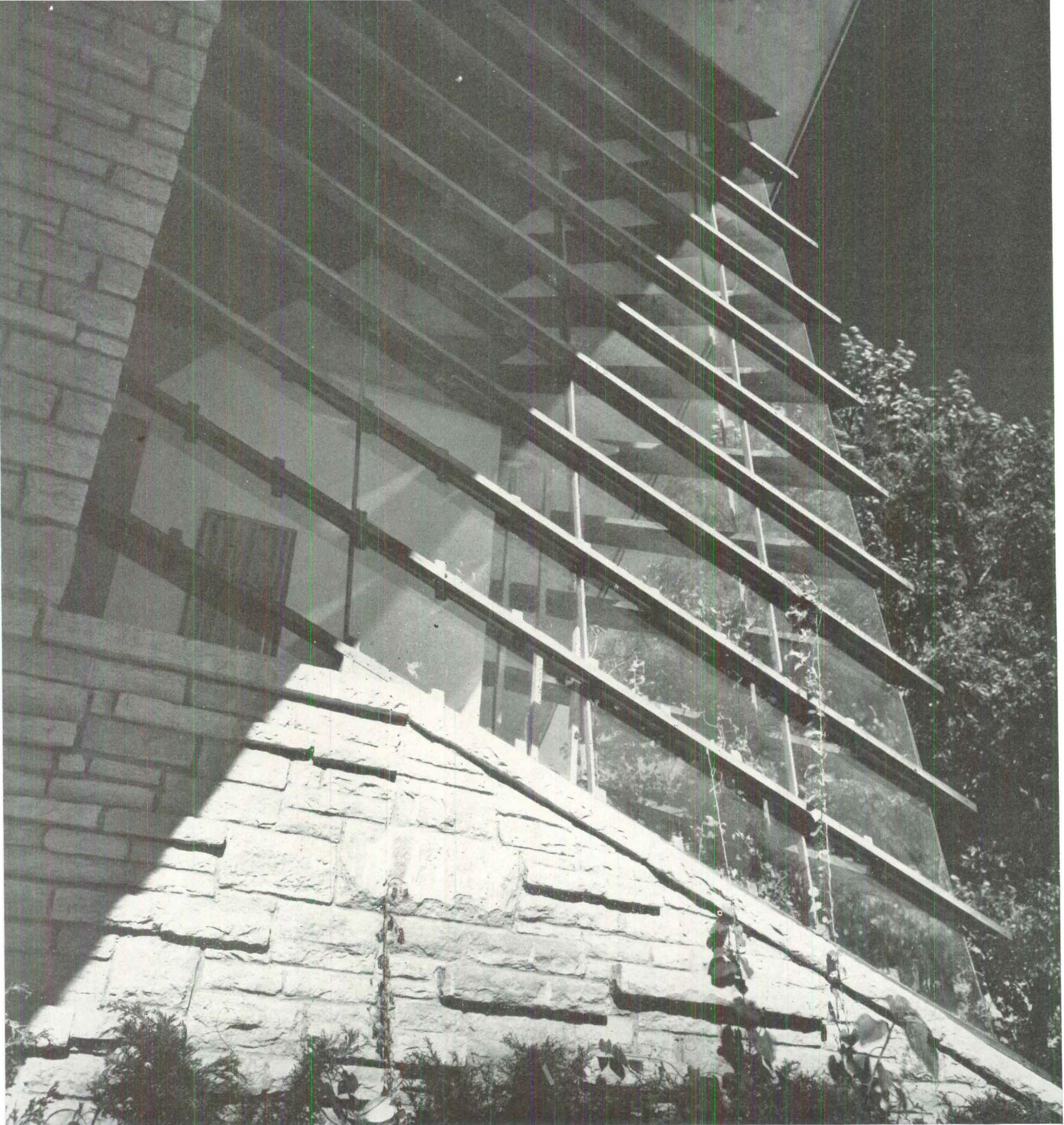
A LAST, CLOSE LOOK AT THE PROW. GLASS ENCLOSING THE APEX IS HELD BETWEEN 2" x 12" LOUVERS AND IS PLACED AT 25% SLANT TO SHUT OUT GLARE
