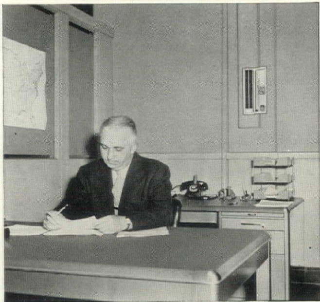
NPB Electric-Centers blend into surroundings naturally, don't have that "electrical look." Wireway extensions replace exposed conduit pipes on wall leading from ceiling to panel cabinet. Column may be extended to floor if desired.
