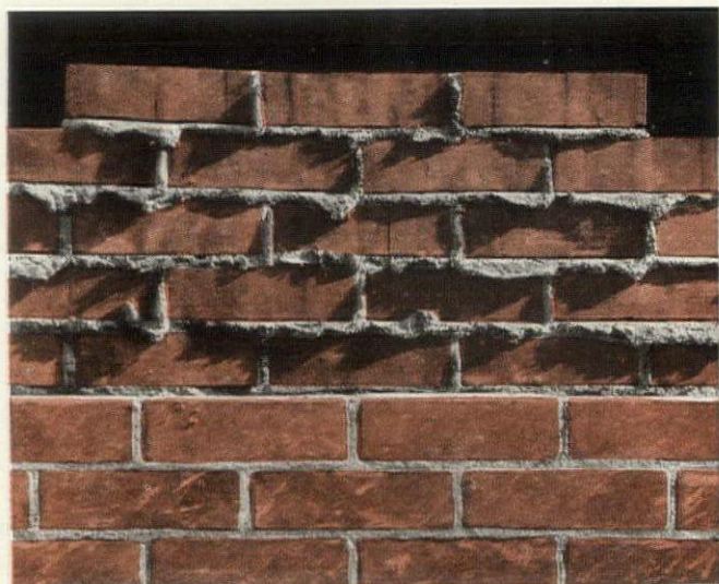
Backplastering should not be attempted over protruding mortar joints.
