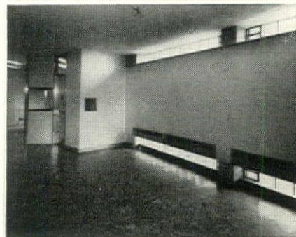
For safe and handsome corridor daylighting: top and bottom glass-block strips
