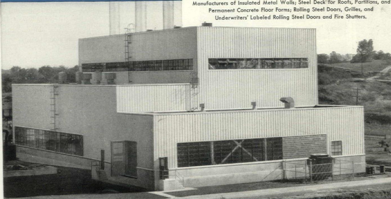
Powerhouse of the new Ford plant, Kansas City, Mo. Mahon Fluted Type Insulated Metal Walls with Aluminum exterior plates were employed throughout in this ultramodern plant. Giffels & Vaillet, Inc., L. Rossetti, Architects and Engineers. Long-Turner Construction Company, General Contractors.
