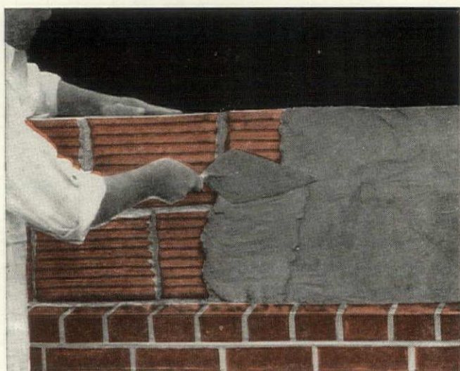
If the back-up units are laid first, the front of the back-up units should be plastered.
