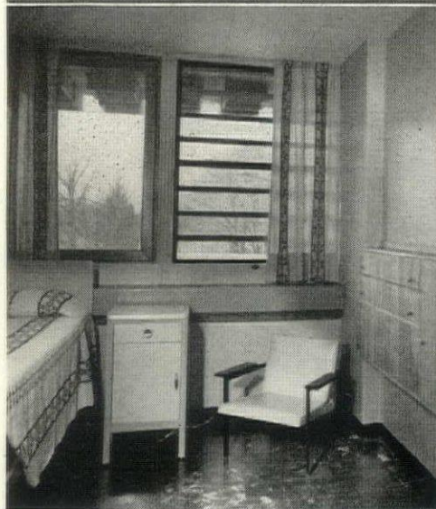
Typical private room. Large window sash is fixed and screened; metal-edged louvers of operative window serve as bars.
