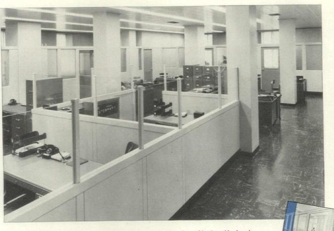
In this layout effective use is made of Mills glazed railings in combination with glazed cornice-high office partitions. Wiring for light, phone and air conditioning controls is easily installed in raceways in base, cornice and panel connections.
