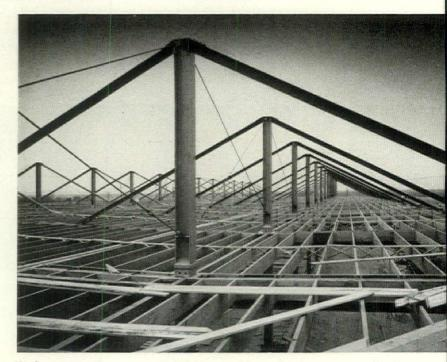
Timber purlins, 2' o. c., span the 22' between main roof girders, are covered with a timber deck and a 20-year built-up roof.
