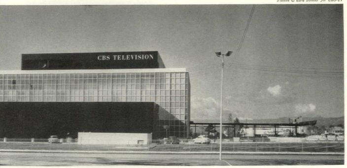
East elevation: dark wall is of demountable steel panel construction. Glass wall also will come down relatively easily when studio must expand.
