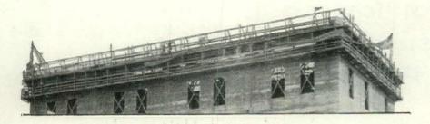
107 ton roof skeleton rises with slipform 99 ft. in 9 days and nights, with 126 jacks and 2 operators
