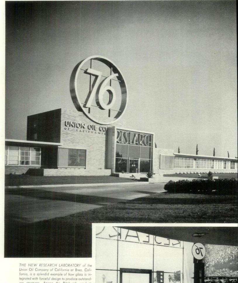
THE NEW RESEARCH LABORATORY of the Union Oil Company of California at Brea, California, is a splendid example of how glass is integrated with forceful design to produce outstanding structures. Among the Pittsburgh products effectively combined here are green tint Solex Heat-Absorbing Glass, Polished Plate Glass, Pittsburgh Doorways, Mirrors, 34" Plate Glass in the lobby display fixture, shown in inset. Architects: Austin, Field and Fry, Los Angeles, California.
