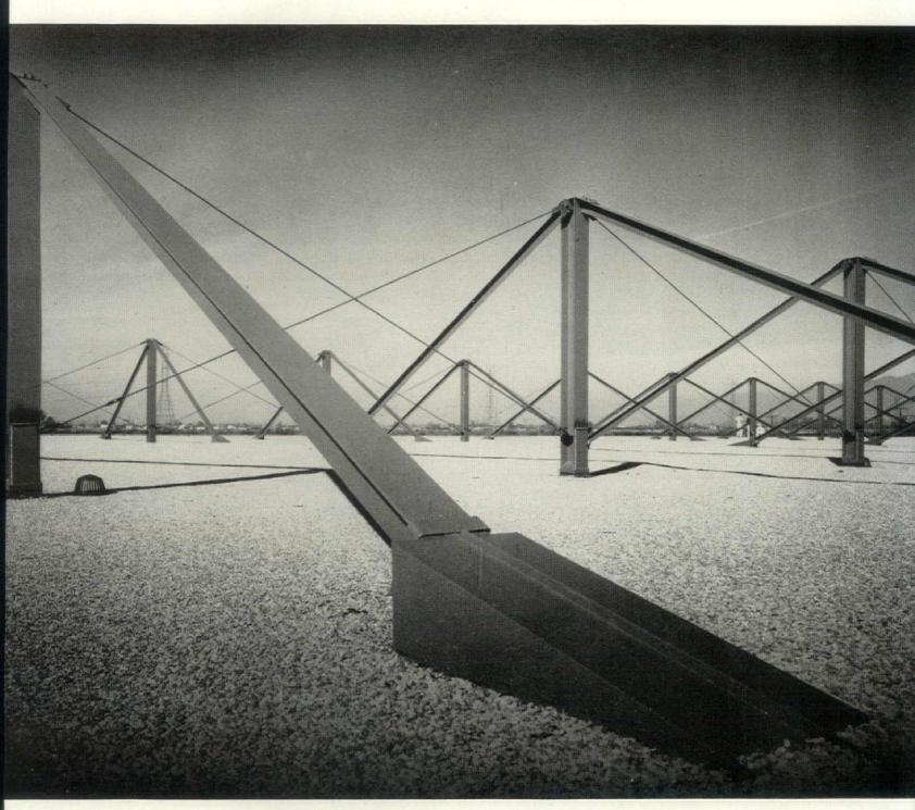
Forest of columns and hangers (above) covers the finished roof. Guy wires and turnbuckles brace structure throughout its length.
