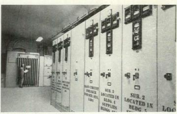
INCREASED PROTECTION of equipment and personnel is provided by G-E metal-clad switchgear. Line-up consists of two incoming-line sections, tie breakers, five sections feeding load-center substations.
