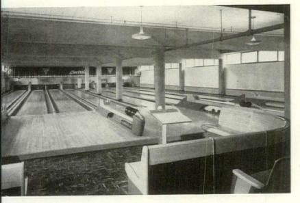
Recreation hall roof is formed by 10' cantilevers and 60' trusses. Center height permits basketball, lower sides make space more intimate for meetings and dances. Optimum range of cantilever vs. truss span fell within hoped-for architectural division of 10'-60'-10'. Note that resolution of horizontal and vertical forces at truss end passes through column footings.
