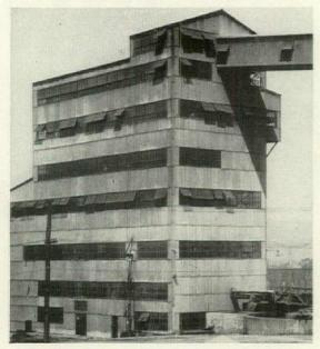
This large coal breaker, roofed and sided with Johns-Manville Corrugated Transite, will provide many years of fire safety and low cost maintenance.
