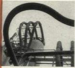
Carey 85% magnesia insulation materials have weathered 24 years of continuous service on the fractionating tower and vapor lines of these atmospheric and vacuum stills at Gulf Oil Corporation's Port Arthur, Texas plant.
