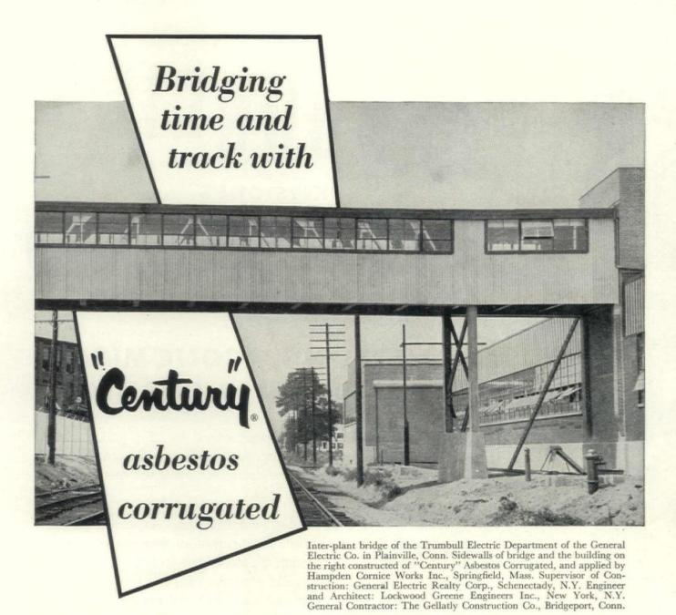
"Century" Asbestos Corrugated makes an ideal siding for this new inter-plant bridge and building because of its outstanding durability and freedom from maintenance. After many years this long-lived siding will still be sound, serviceable, and weather-tight.
