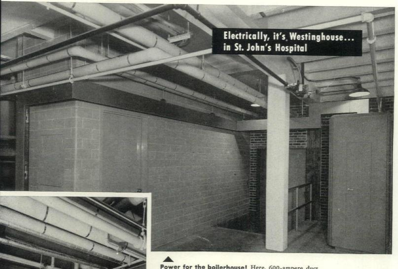
Power for the boilerhouse! Here, 600-ampere duct feeds the 300-kva sub-power center in the boilerhouse. Note how duct hugs the wall. This run is over 400 ft. long.
