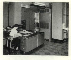
Now available in 3,5 and 71/2-ton sizes, these Frigidaire self-contained air conditioners can actually be employed to handle almost any air conditioning need. With the addition of optional heating coils, they provide year round service.
