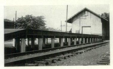
ABOVE—Sonotubes were used for fast, inexpensive construction of this railroad siding platform.
