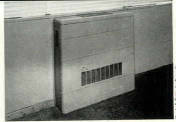
Typical fan-coil unit in Woodner apartments provides cooling and heating, is recessed 5" in wall, extends into room 7".
