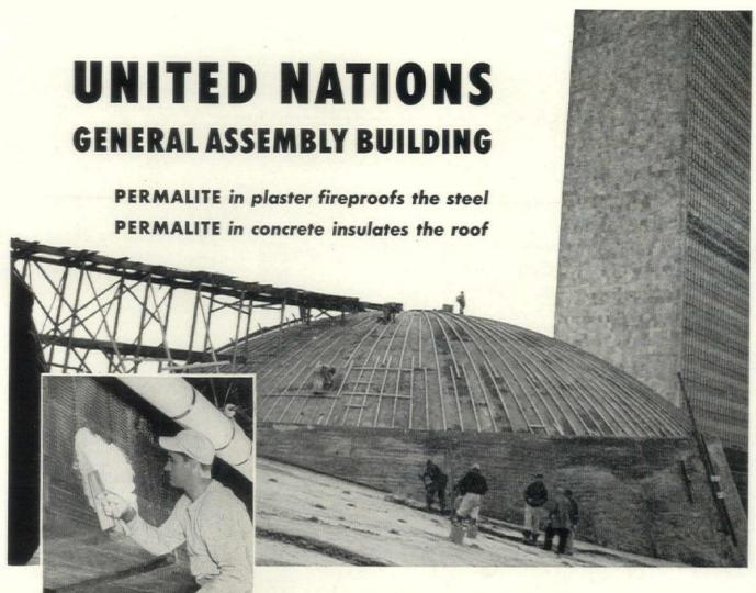
54,000 sq. ft. of plaster with Permalite were used to fireproof steel not only in General Assembly Building but also in two meeting halls. Plaster was applied 1" thick on expanded metal lath over steel beams, girders, trusses.
