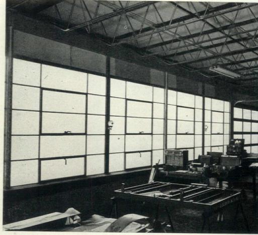
Heat-absorbing windows are welded directly to alternating pipe columns and mullions.
