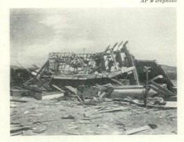
TEST HOUSE No. 1, 3,500' from last month's test atom blast at Yucca Flat, was splintered into this nile of rubble, but . . .
