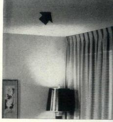
Plywood-formed ceilings were painted after grinding, spackling.
