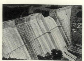
60,000 tons of ice went into Philpott dam, Va. Right, aggregate flow diagram.
