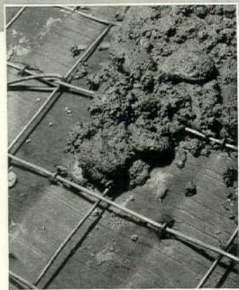
Note, in the cross-section and close-up that the weight of the wet concrete forces the backing away, which permits the galvanized welded wire mesh to assume its proper position in the slab. Steeltex Floor Lath also performs two other functions. It permits work on the floor below while pouring is in progress and retains moisture to assist proper curing.
