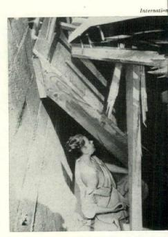
DESPITE COLLAPSE of house No. 1, the leanbasement shelter protected mannequin fro falling beams, although not from radiation.
