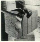
In application the structural concrete may be drilled, nailed, sawed, or chopped like ordinary lumber.
