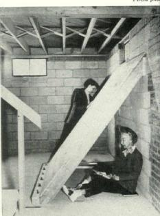
LEAN-TO SHELTER installed in test house No. was a type that a home handyman might bui for about \$40. Seated model (before blast) show how to use it.
