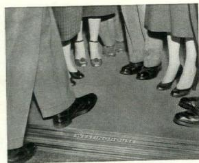
UNIQUE WEIGHING DEVICE SPEEDS PASSENGER SERVICE—an unseen scale weighs passengers, and, when the car is loaded, closes the doors and starts the car . . . this does away with overcrowding, improves service, saves time.
