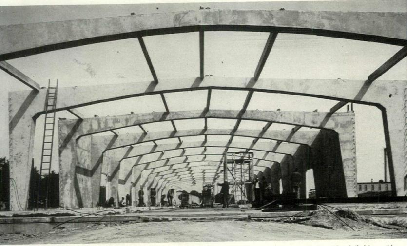
Concrete frames weighing 22 tons each are cast on the floor slab and tilted into position
