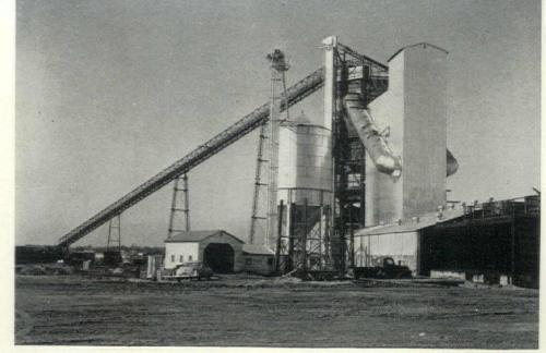
Batching tower at Folsom dam, Calif. contains refrigerating equipment and mixers
