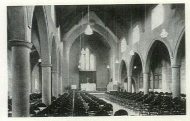
ABOVE—Interior of First Lutheran Church, Seattle, Wash., with Sonotubeformed concrete columns.
