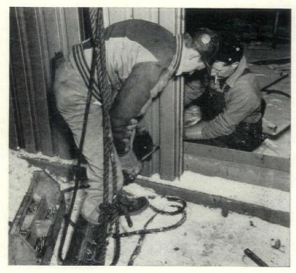
EVEN SEVERE WINTER WEATHER didn't halt erection of Stainless Steel panels on this laboratory and office building. Fast erection will out regard to weather conditions is only one of the advantages of this type of construction.
