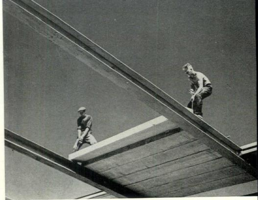
Roof-deck slabs, primarily used for their thermal and acoustical insulation qualities, also provide a pleas white finished ceiling surface. The 12' x 20" x 5" sections of Zeprex are handled easily by two men.
