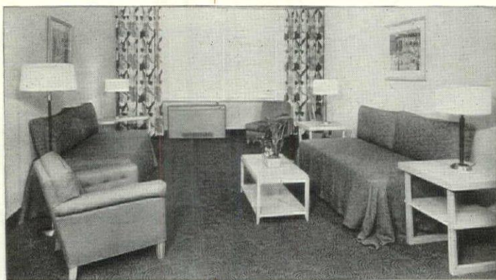
Hotel guest rooms have units supplied, during the heating season, with hot water and, during the cooling season, with chilled water controlled by Johnson Submaster instruments. Many individual offices in the building have Johnson T-432 Heating-Cooling Room Thermostats in addition.
