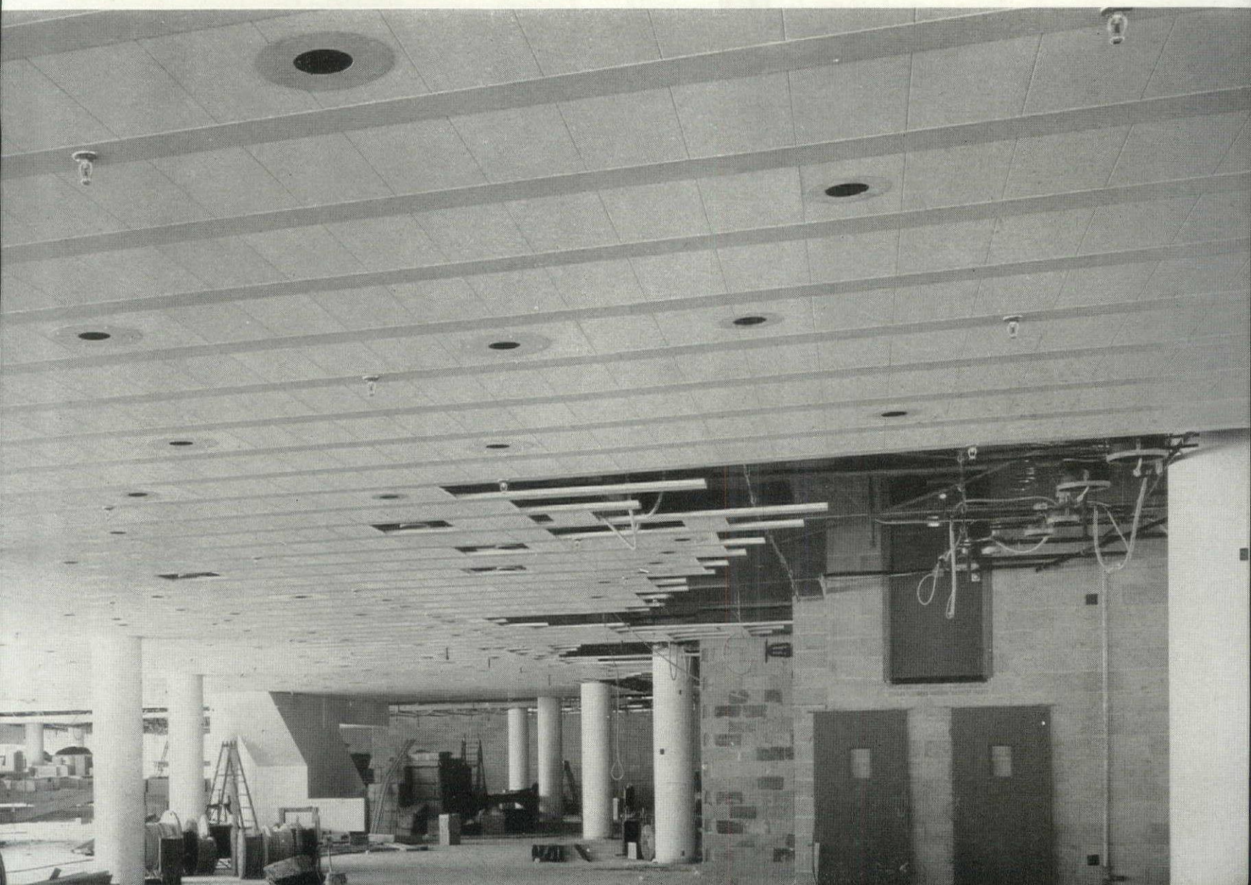
Flexible armored conduits connect each bay's junction box with its lighting fixtures. Slack in conduit permits rearrangement.
