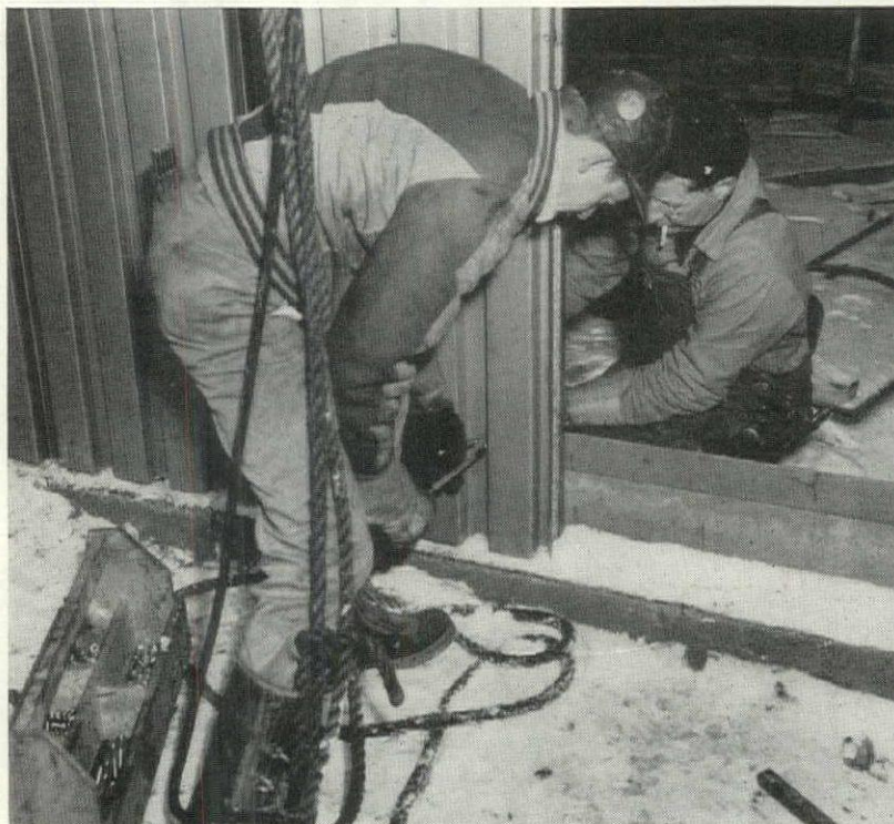
EVEN SEVERE WINTER WEATHER didn't halt erection of Stainless Steel panels on this laboratory and office building. Fast erection without regard to weather conditions is only one of the advantages of this type of construction.
