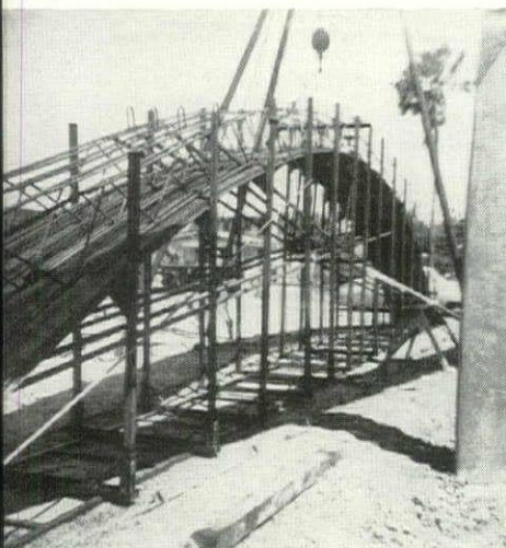
Welded reinforcing is placed for four 50' arches to be cast simultaneously.
