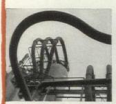
Carey 85% magnesia insulation materials have weathered 24 years of continuous service on the frac-tionating tower and vapor lines of these atmospheric and vacuum stills at Gulf Oil Corporation's Port Arthur Town Very Lines Port Arthur, Texas plant.
