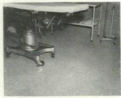
flebacked and 1/4" thick, it conducts static electricity from tile to tile through the tightly butted edges. It is available in three pastel tones in 9" and 1' squares at \$2.50 per sq. ft., in place. Waxing-which tends to reduce conductivity after several applications-is not required for maintenance. Heavy-gauge aluminum foil laid beneath the tile assures faultless and permanent conductivity.
