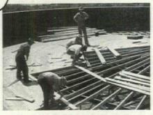
nanized lumber, on steel framing, gives lasting otection and insulation to this Orlando, Fla. reservoir.
