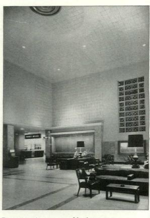
Proper acoustics were assured for the spacious main lobby of the terminal by installing Travertone not only on the ceiling area but on sections of the walls as well.
