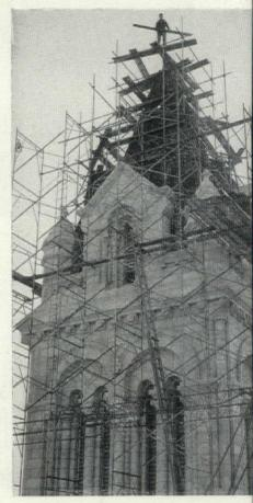
One of the largest churches west of the Mississippi, St. Louis Cathedral has been undergoing renovation for several months. The twin towers rise 157 feet above Lindell Boulevard. Old wood stripping, which can be seen through the scaffolding, was put on at the turn of the century with handmade nails.
