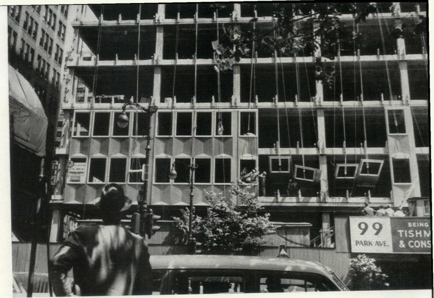
Two-story aluminum panel is picked up off floor and hoisted into place by three men with aid of block and tackle
