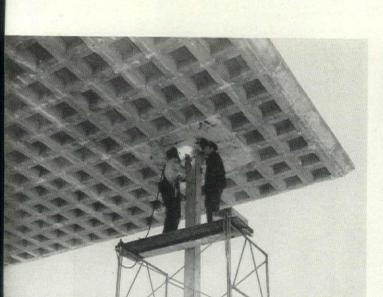
"Waffle" block slabs are welded atop 24' steel columns. Underside of slab (right) shows four-piece, 2' square coffer blocks on which slab is poured.
