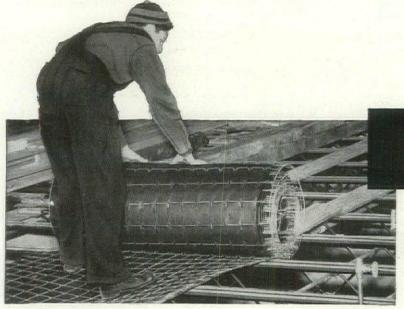
One man can roll out a 125' roll of Steeltex in a few minutes. Steeltex provides both waterproof form and steel reinforcement for concrete floors.
