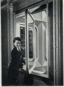
Aluminum windows will be closed and locked except for cleaning, effected from the interior by pivoting window on vertical axis. In cross section, windows contain sections ¼-inch-thick plate glass, ½-inch air space and ¼-inch-thick heat-absorbent plate glass on the weather side.
