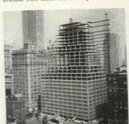
prise two 4'-6" high spandrel sections, diepressed into a 5" deep concave pattern for rigidity, and two 6' high aluminum window frames with stainless-steel weatherstripping, all shop-welded between a pair of 23'-3" extruded aluminum "mullions."
