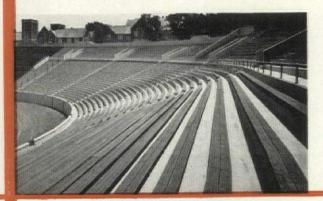
WATERPROOFING Grant Field, Georgia Institute of Technology. Problem: Concrete stands were deteriorating and even steel reinforcing rusting. Solution: South stands, comprising some 65,000 square feet were completely resurfaced with SURCO Yellow label roofing mix.
