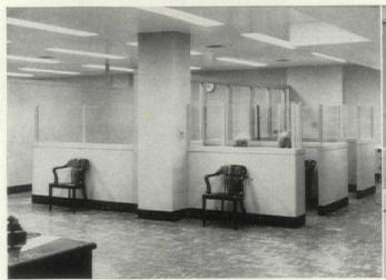
There will be no dust or debris when these semi-private offices are rearranged. Whole sections of Mills Walls may be moved intact, all parts used over and over again.
