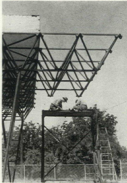
Erector-set space-frame is the latest development of the industrialized school (AF, Nov. '51). This steel classroom frame at the University of Michigan is loaded with 60 psf of water (contained in plywood bulkheads). Strain gauges showed that the three-dimensional bolted truss, made of light uniform members, has tremendous strength. Weight of finished roof: 16 psf.
