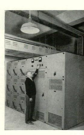
Low-impedance bus duct riser carries power from low-voltage switchgear to panelboards, located in wire closets on each floor.
