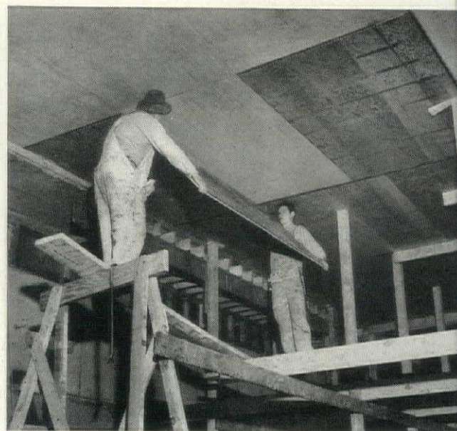
View shows stripping off ceiling forms. Smooth fir plywood panels permitted structure and finish surface to be cast simultaneously. Exposed concrete surfaces, both inside and out, were painted direct after a minimum of rubbing, eliminating expensive plastering on ceilings.
