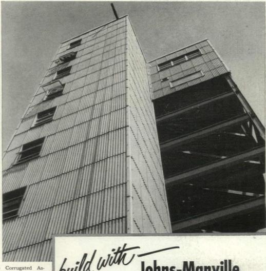
Johns-Manville Corrugated Asbestos Transite gives this airport control tower an attractive, fireproof exterior that offers years of maintenance-free service despite exposure to extreme weather conditions build with Johns-Manville
