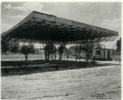
Erector-set space-frame is the latest development of the industrialized school (AF, Nov. '51). This steel classroom frame at the University of Michigan is loaded with 60 psf of water (contained in plywood bulkheads). Strain gauges showed that the three-dimensional bolted truss, made of light uniform members, has tremendous strength. Weight of finished roof: 16 psf.
