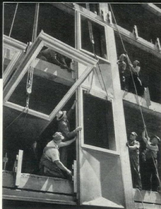
Workmen operating from inside of building, putting aluminum panel into position ready for bolting to steel brackets on framework.
