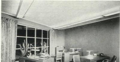
**FLEXIBLE!** Completed offices in the new Sinclair Oil Building will have handsome, sound-absorbing ceilings like the typical Travacoustic installation shown here. The Gold Bond "J" System, used with kerfed and rabbeted Travacoustic, is adaptable to designs that include recessed light troffers and complex stepped ceiling assemblies. It can also be used with gypsum board bases to which acoustical materials may be applied.
