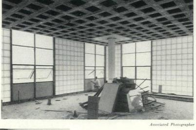
Waffle lift-slabs in Peoria, Ill. school by Architects Hewitt & Bastian provide wide, flexible spans for \$2 per sq. ft. erected (AF, Sept. '53). Lightweight blocks in each slab were left exposed, giving 50% noise absorption. Construction cost of the two-story school: \$11.48 per sq. ft.
