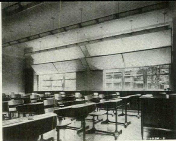
Contemporary daylighting comes to old classroom (left) with installation of woven glass-fiber panels set at an angle along the windows to diffuse harsh sunrays.
