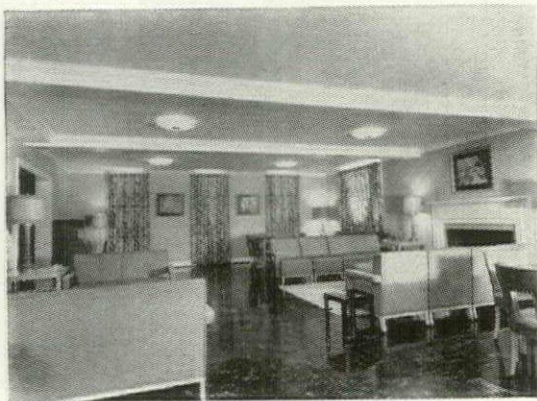
High acoustical efficiency rather than dignified appearance was the requirement for the sound conditioning in the Informal Lounge. Here, low-cost Armstrong's Cushiontone, a perforated wood fiber tile, was chosen to do the job.
