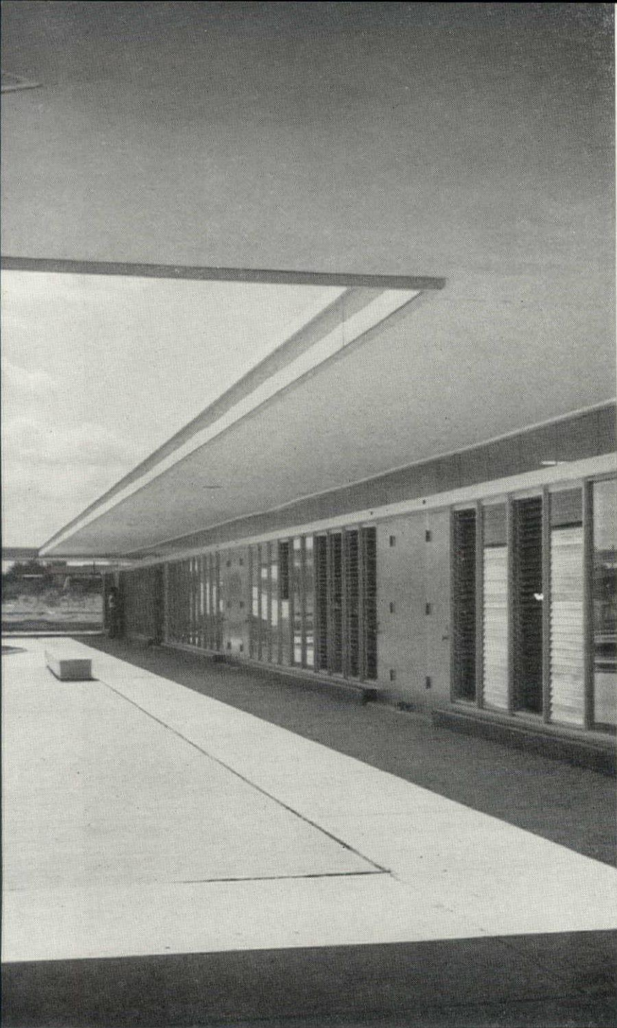
Under plaza overhang is classroom wall made principally of glass jalousies. Overhangs shade glass, also shelter exterior corridors.
