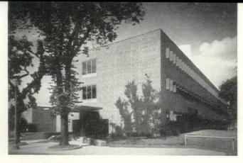
Short windows leave good vertical surface for upholstering with acoustical absorbent, important in view of wide use of television and other teaching aids in this laboratory high school. Note that wall over windows is painted light color and has luminaire close to it to diminish contrast with light through windows.
