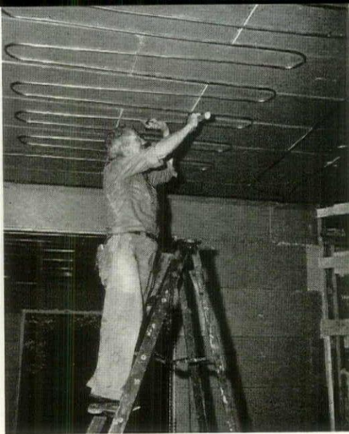
FACTORY-FORMED COPPER GRID knocks 4¢ per lin. ft. off cost of radiant panel; one size adaptable to entire system
