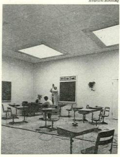
Experimental mock-up of typical classroom in Hillsdale High School shows two of the ceiling light wells that are topped with glass-block skylights. Also integrated in the hung ceiling are air-conditioning ducts and grilles, recessed lighting and acoustical treatment.
