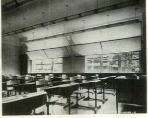
daylighting comes to old classroom (left) with installation of woven glass-fiber panels set at an angle along the windows to diffuse harsh sunrays.
