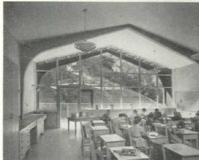
Three-hinged, Y-shaped frames are independent of walls and partitions. Deep roof overhangs, plus trees outside glass gable end, provide plenty of shade (see cut). Glass gable ends face northeast and southwest (but on northeast side glass is limited to clerestories above corridor roof). Partitions between classrooms could be knocked out to create bigger spaces.
