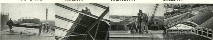
Pre-cut, pre-curved (if desired) sheets, up to 22 feet in length, in 18 inch widths, permit fast easy, handling. Grooved for simple end-overend attachment, Tri-Rib sheets go down quickly, save valuable building time. They fasten quickly, too, either by clipping or welding. No complicated dovetails or attachments to slow down work.
