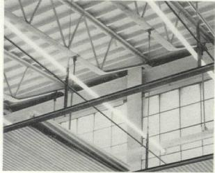
Brightness without glare results when this luminous ceiling of corrugated plastic merges with all-glass wall. Fluorescent tubes are hung above plastic diffusing panels. (See text.).
