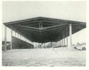
Inverted truss in Compton, Calif. school by Architect H. L. Gogerty is achieved with low-pitched laminated beams. Vented attic space is available for utility ducts and piping while sloping ceiling gives excellent lighting and acoustics. Construction cost: \$14.62 per sq. ft.
