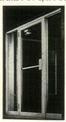
and double-acting models, feature plastic glazing channels which, by eliminating putty, are said to cut glazing costs. The bolts connecting the corners through top and bottom rails are held securely by vibration-proof locknuts. Each door unit is equipped with pull handle and push bar, concealed floortype closers, threshold, and standard 1-5/32" lock cylinder. Installed cost of a single-acting door is about \$215.
