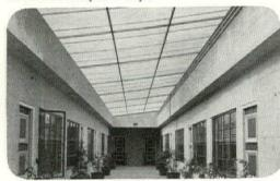
**alsynite** provides unlimited daylighting . . . skylights, side walls, etc. No framing needed.
