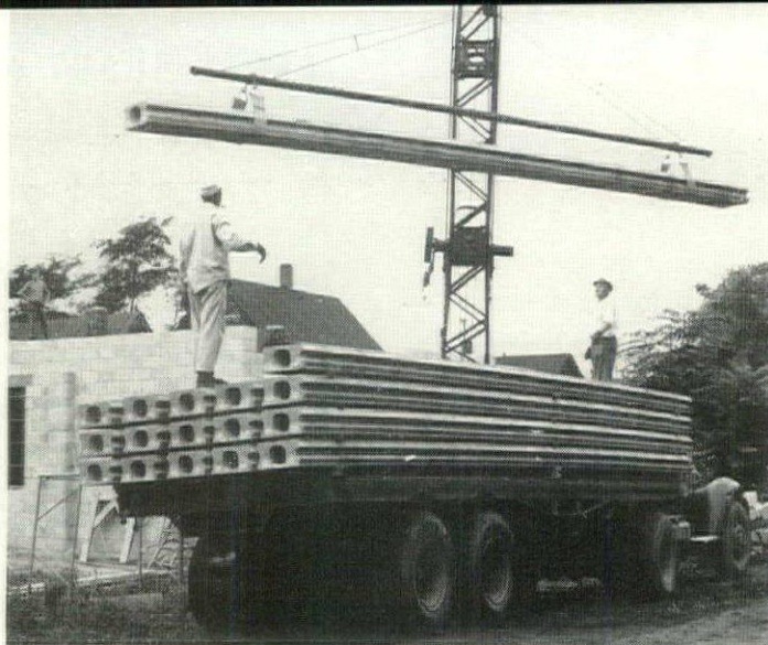
From truck to deck. Lifted by crane as they come from the factory, the concrete beams are set in place side by side to make up the structural roof or floor deck.
