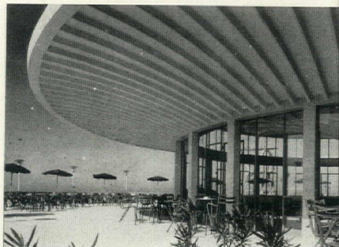
One thick central column supports main roof of restaurant at Ostia. Circular terrace roof is cantilevered outward from a circle of small concrete piers. Both roofs are formed with thin precast concrete pans like vault of room C at Turin (left). Mushroom roof of the dining room required 144 precast pans (detail left) of six different sizes and shapes. Architect: Attilio La Padula. Design was done in 1951.
