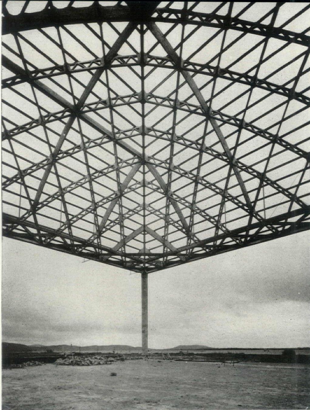
Later version of hangar (1942) uses prefab ribs with light, open quality of steelwork
