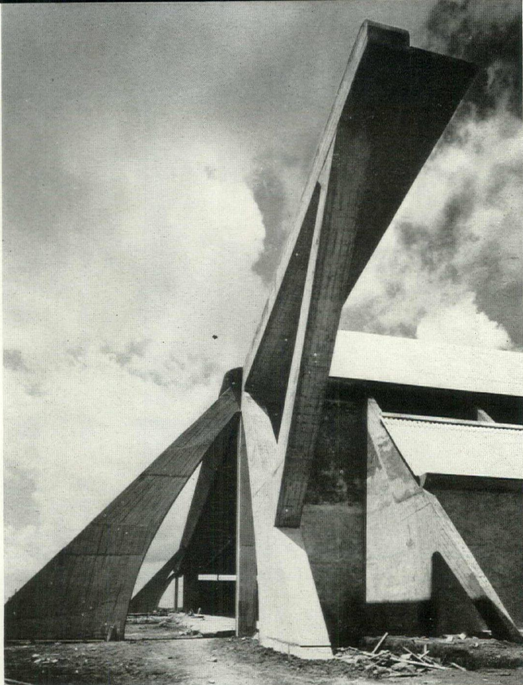
Early hangar (1938) needs massive buttresses to hold up heavy vault of poured-in-place ribs
