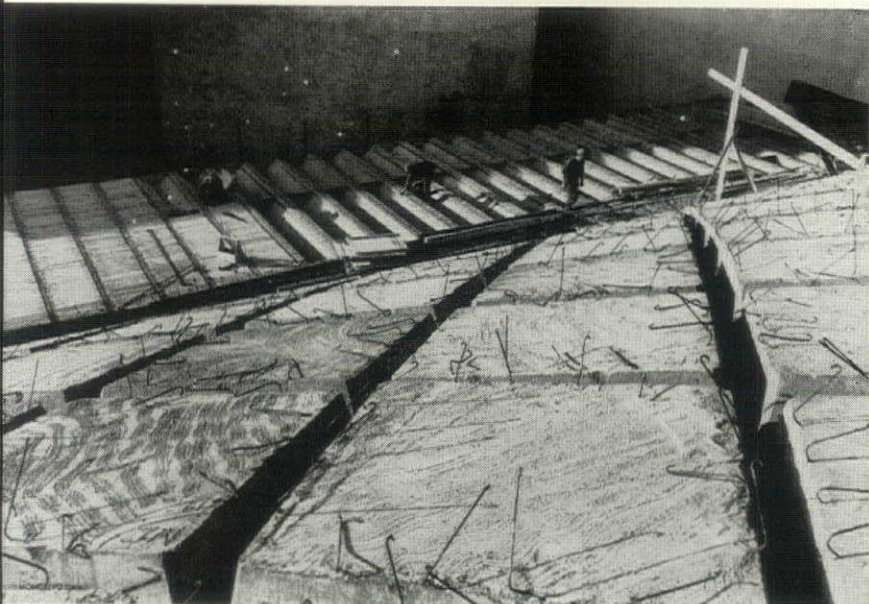
Construction view of room C shows framework of vault in place: inverted pans between and over which concrete will be poured to form ribs and roof. In background are undulating beams over peripheral aisle, some of which have been covered by flat slabs and are ready for grouting.
