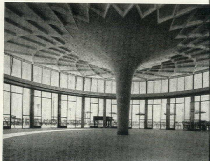
One thick central column supports main roof of restaurant at Ostia. Circular terrace roof is cantilevered outward from a circle of small concrete piers. Both roofs are formed with thin precast concrete pans like vault of room C at Turin (left). Mushroom roof of the dining room required 144 precast pans (detail left) of six different sizes and shapes. Architect: Attilio La Padula. Design was done in 1951.
