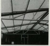
annoyance of surface glare. Cost of Spun-Lite will run around \$1.25 per sq. ft. not installed. For application to wood, the manufacturer recommends the use of aluminum nails with neoprene washers. For fastening to metal framing, brass or galvanized nuts
