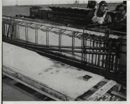
Reinforcing steel is prebent to speed installation. Solid prestressing bars, each 11/8" diameter, are sheathed against bond.
