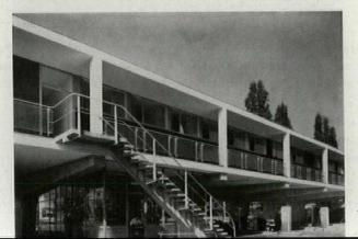
SUSPENSION of outdoor ramp consists of series of 1½2"-diameter steel rods anchored in projecting ends of roof beams and in 7½2" ramp slab. Ramp is 14' wide, has gradient of 14.5% up (14% down). Note ramp down to basement in foreground of photo at right.
