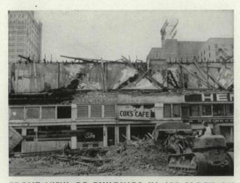
FRONT VIEW OF BUILDINGS IN 400 BLOCK ON FRANKLIN STREET shows the terrible toll the tornado took of buildings whose frame construction was less rigid than reinforced concrete. This is typical of the fate of the load-bearing wall-type of structures in the twister's path!
