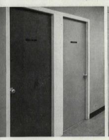
Weldwood Fire Doors in Lever House, New York City. These wood-faced doors carry the U.L. label for Class B and C openings. Should a fire break out, the mineral core is an effective fire-check. Arch: Skidmore, Owings & Merrill.
