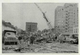
DEBRIS IS ALL THAT REMAINS OF 5-STORY R. T. DENNIS BUILDING. This and four other buildings in the immediate area were obliterated by the storm. The buildings in the rear both have a reinforced concrete frame.
