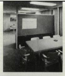
Conference-room wall (view is toward architect's office) is glass-topped, has pin-up panel of fiber-board covered with burlap, lower panel of painted plasterboard. Negative joints emphasize panel treatment. Dropped ceiling, housing air cooling, stops short of old office-building windows.
