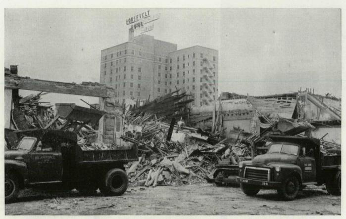
ROOSEVELT HOTEL STANDS ALONE AMIDST WRECKAGE. Although located in the heart of the tornado's path, The Roosevelt Hotel stands unyieldingly in a block that was more than 50% destroyed by the rampaging winds. Engineers reported "no structural damage" to this 12-story reinforced concrete frame building.
