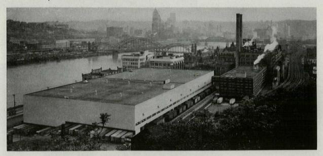
Platoon of old buildings, arranged on grid beside river, was restudied in 1947 by Skidmore, Owings & Merrill (AF, May '49). New buildings are designed with eye to possible floods, with no vulnerable underground cubage, and with most machinery on upper floors. SOM's master plan will guide future work.
