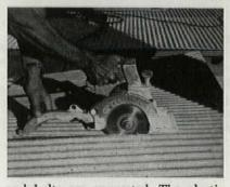
and bolts are suggested. The plastic can be cut with a handsaw or power saw.
