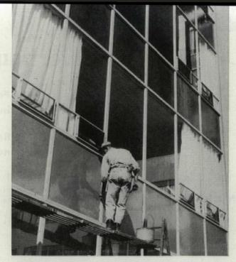
Spandrels at central block and playrooms (below, left) are 3/8" curtain wall of blue porcelain-enamel steel on aluminum honeycomb core. Architects first experimented with heat-resistant glass spandrels.
