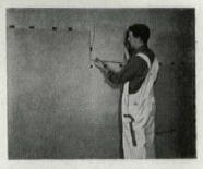
wall for a remodeling job or onto furring strips or studs in new construction. Allowance is made in the joints for concealing either kind of fastening device (see drawings below). The 16"-square Marlite Block are put up the same way. Besides the ten
