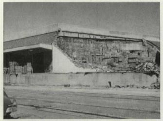
DRAMATIC ILLUSTRATION OF THE ABILITY OF REINFORCED CONCRETE TO WITHSTAND THE TWISTER is the Waples Platter Co. building. At right is all that remains of the brick portion of warehouse, but reinforced concrete section, left, is structurally unaffected by the storm.
