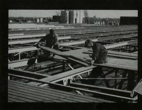
Time is money on every building job! Milcor Steel Roof Deck gets operations under cover fast at low labor costs, gives ideal base for permanent roofs.
