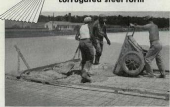
for concrete floors and roofs...stronger by far than conventional corrugated steel of same shape and weight... functions as a base for thin concrete slabs in steel joist floors and roofs...economies of construction are a result of thinner, stronger slabs...concrete saving through lack of sag, stretch, bend or leakage...speed and ease of placing Corruform also adds to construction economy.
