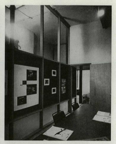
Conference room is separated from reception hall by partition consisting of 1' x 3' x 2" panels of cold-storage insulation cork set between 2 x 4s, with obscure glass below, clear glass above. Room has skylighting plus cylindrical floods.
