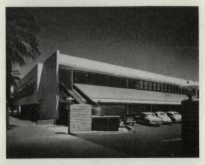
Main stairway to second floor leads from parking lot on west. First-floor framing is reinforced concrete with 20' spans; second-floor, light steel.
