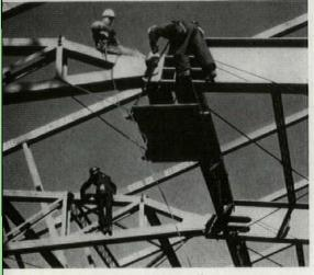
Pin-connected joint allows maximum vertical movement of 115' long trues.
