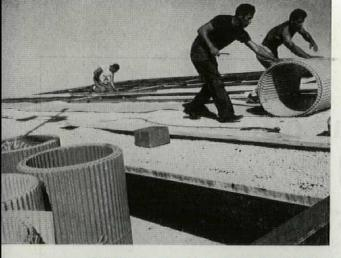
Rolled out from a 100' strip, the transluscent plastic sheeting is easy to handle and apply.
