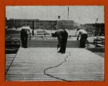
Unique design permits sections to be nested and lapped quickly and easily. Plates interlock firmly, providing an unbroken roof surface that is adaptable to any degree of insulation.
