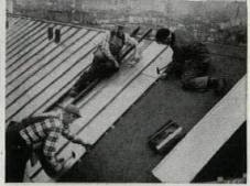
PREFABRICATED PANS of 16 oz. Revere Copper being fastened into place with cleats, using two nails per cleat, Pans are 17 ¼" wide by 8' long and attached top and bottom with loose lock cross seams
