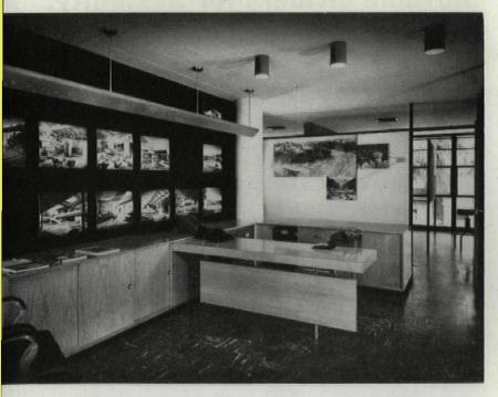
Reception area is divided from work space by display walls. Most partitions, like that behind desk, go to 7' with glass above for space continuity. Same 7' height with glass was used for masonry portions of first-floor exterior walls to give floating quality to second floor.
