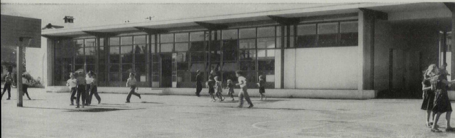
Playgrounds and windows go together and dangers and hazards of vandalism are reduced by using Tuf-flex in these windows at Beresford School, San Mateo, Calif. Architects, Kump and Falk, San Francisco.
