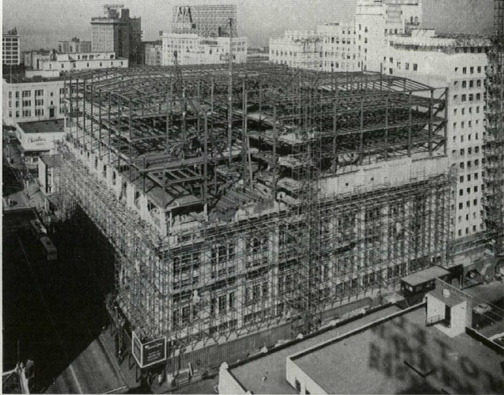
Five-story welded frame, weighing 10.9 psf (1,756 tons, 321,000 sq. ft.) and fully continuous in both directions, is built atop five-story, 38-year-old reinforced concrete structure.
