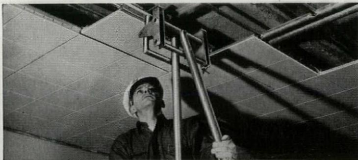
WORK-SPEEDING METHODS , such as this new way of crimping aluminum ceiling panels to water-circulating aluminum tubing resulted in fast completion.
