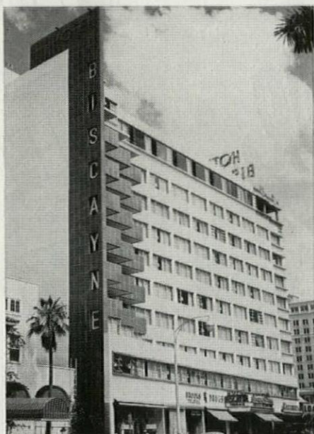
Biscayne Terrace Hotel in downtown Miami has 200 rooms, 10 stories, cost $2 million. 250,000 square feet of Steeltex in floors and roof. Albert Anis and Melvin Grossman, Architects. Edward M. Fleming Construction Co., Contractors.
