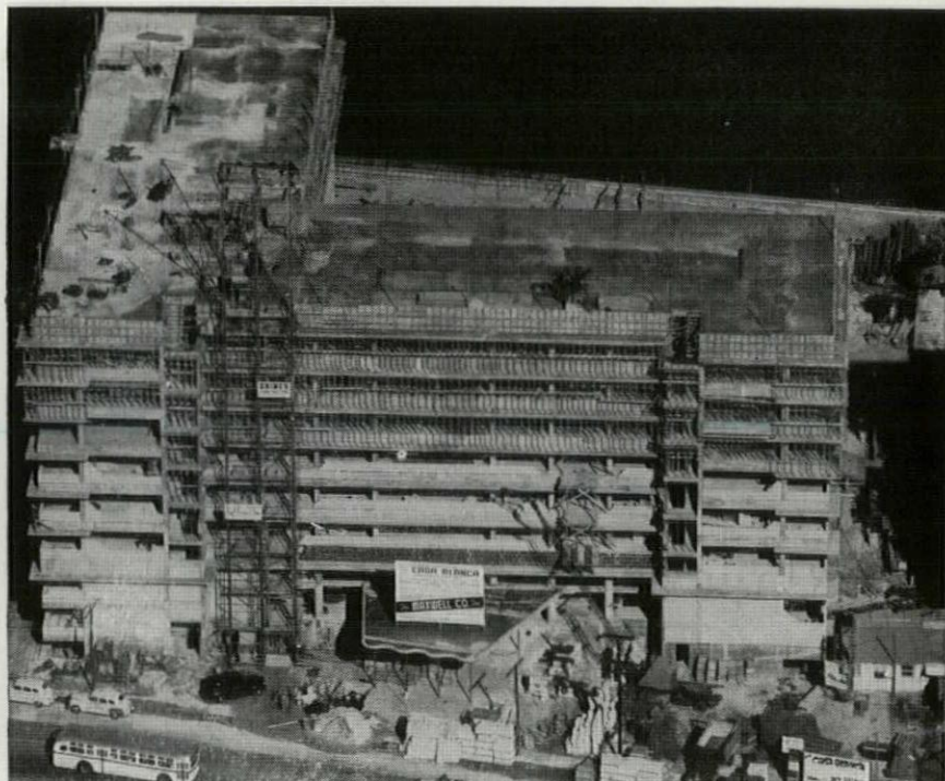
The 9-story Casa Blanca Hotel, Miami Beach, shown here while under construction, is now in operation, cost $2.2 million, has 250 rooms. Steeltex used in all floors and roof. Roy F. France & Son, Architects. Gaines Construction Co., Contractors.
