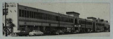
Construction above and below vision strip on Woodward Avenue side of building consists of enameled glass outer face, air space vented for condensation drainage, FOAMGLAS adhered to transit and backed up with composition wall board. End wall construction is similar except that enameled porcelain is used in place of enameled alass for the outer face
