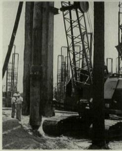
Twelve-ton vibration machine is suspended from crane, ready to start a fresh compaction, one of 3,350 made 8' o.c. throughout phosphate plant.
