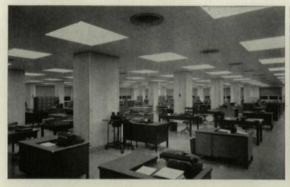
Mistakes are held to a minimum in the company's Underwriting Department. Here, the distracting clatter of typewriters, business machines, and voices is effectively muffled by the Arrestone ceiling. This material offers a maximum of sound absorption.
