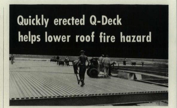
The many unique features of Robertson Q-Deck make it of special interest to the architect and engineer who is concerned about the fire hazard aspect of his flat roof design. To begin with, Robertson Q-Deck is designed with tight side and end laps to eliminate the need for an inflammable vapor seal. Its two-foot width and long span characteristics mean fewer joints, and its zinc-coated surface (or basic Galbestos) eliminates the need for field painting.
