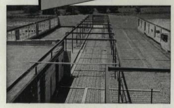
TWO VIEWS of the radiant Panel heating layout before concrete slab was poured. Floor area over 17,000 sq. ft. System was imbedded in slab 4". Gravel fill is 6" deep. Coils are 12" OC. System is divided into 4 zones, with all supply and return lines also of copper. Note edge insulation at right in large photo.
