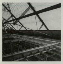
By day natural light is filtered to glass diffusing ceiling through adjustable plastic louvers to give maximum daylight without glare.
