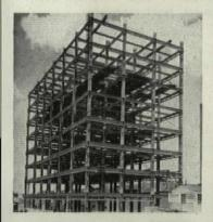
Life Ins. Co. Bldg. shows partial erection of structural steel. Cofar placing followed immediately. Cofar units weigh only 2 lbs. per sq. ft., are bundled for individual bays, arrive at job site cut to fit building frame.
