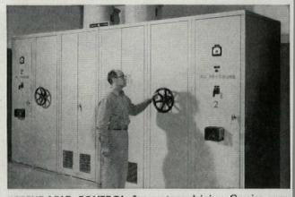
**DEPENDABLE CONTROL** for motors driving Carrier compressors is provided by this 5000-volt G-E unit, which was ready for operation upon installation.
