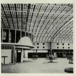
structure, 145' span, with precast concrete roof slabs, designed for the Rotterdam's Grain Exchange building by the writer in 1937. The concrete slabs have incorporated circular skylights specially designed for diffused light which is necessary for examination of grain quality. J. F. Staal was the architect.
