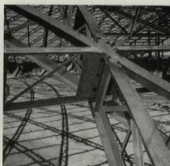
Identical connections throughout arch simplify erection. The 260 ton, 65,000 sq. ft. frame was completed in 25 days.
