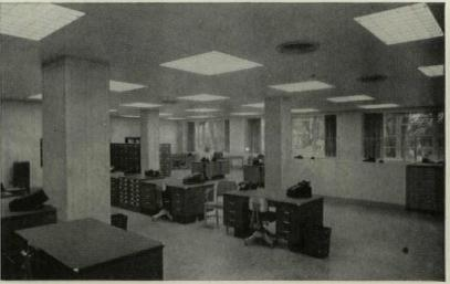
Modern recessed lighting in the Accounting Department and throughout the building helps prevent tiring eyestrain. The white, baked-on enamel finish of the Arrestone ceiling helps diffuse the light evenly all over the room, without annoying glare.
