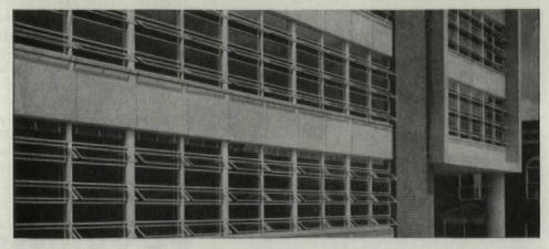
Notice how the vents of these Fenestra Intermediate Steel Windows protect the interior of the Clemson College chemistry building in Clemson, S. C. Here is fresh air ventilation even when it's raining outside. And these vents operate so that you can wash them from inside. Screens also go on from inside. Architects Hopkins, Baker & Gill designed the building and Industrial Builders Inc. built it. Both are in South Carolina.
