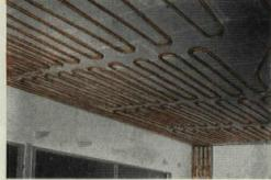
Note close tube spacing near outside wall where heat loss is greatest. Tube spacing is progressively increased as grids are installed nearer the
