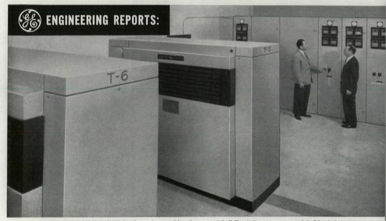
**COMPACT POWER DISTRIBUTION** for the entire new May Co. store in Lakewood is provided from these "packaged" units. G-E dry-type transformers, foreground, step down incoming voltage,
