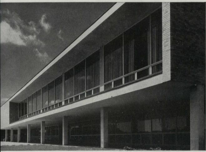
Main entrance elevation of St. Vincent's Home. Truscon Intermediate Projected Windows combine with Truscon Picture Windows in second floor facade; Truscon Intermediate Steel Casements on ground floor.
