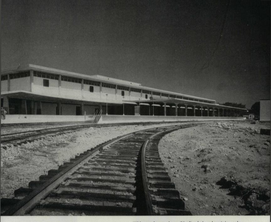
Wide overhangs along rail loading docks and at windows reduce Florida sun glare and offer protection against sudden southern downpours. (Glare is further reduced on east and west elevations by use of tinted glass.) Railroad still is big factor in Biscayne Annex, but trucking dock space is daily usurping RR importance in nearly all such terminals for handling mail in bulk.
