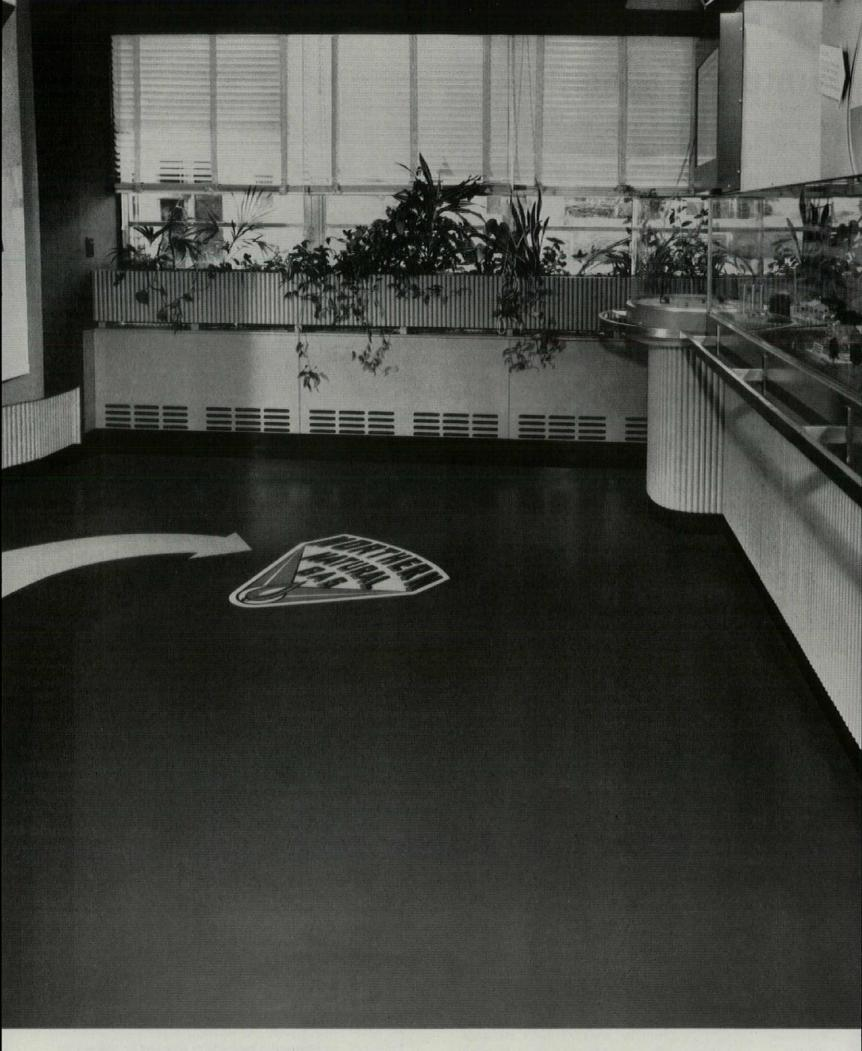
The moderate cost of Armstrong's Linoleum, along with its ability to withstand concentrated traffic, makes it a favorite floor for showrooms and lobbies. Decorative insets are easily worked into this flooring. Since this material comes in rolls 6' wide and up to 90' long, it provides a smooth surface with few dirt-catching seams.
