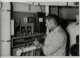
ig cost-saving factor is B-C "Control Center" in boiler room. lere, at one central junction point, are prewired accessories and numbered terminal strips for connecting all electrical components of each unitary control system.
