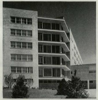
Interesting corner detail shows Truscon Steel Picture Windows combined with Truscon Intermediate Combination Steel Windows. Adjacent wall sections fitted with Truscon Steel Double-Hung Windows.
