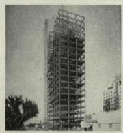
August 24. Steel framework is completed! Note that Cofar has already been placed on 13 floors providing a safe, unobstructed working platform for construction activities. Trades can move in, complete their work without delaying concrete operations.
