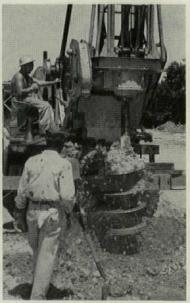
Oversize spiral bit (left) drills a 20' hole in 9½ min. Bottom of hole is reamed out by special tool (below); reinforcing steel is then placed and footings poured. Footings: McKinney Drilling Co. Gregson & Ellis, architects; Harry Hunter structural engineer; George A. Fuller Co., general contractor.
