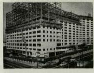
On the new Statler Hotel, Los Angeles, (above) PLYGLAZE concrete form panels averaged 15 re-uses. Huge Parklabrea apartment project, (below) required over 750,000 square feet of PLYGLAZE for ceilings and exterior walls. Concrete was so smooth that ceilings were merely painted and left exposed.
