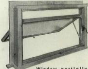
Window partially opened to 45° angle (Right hand stop re-moved)
