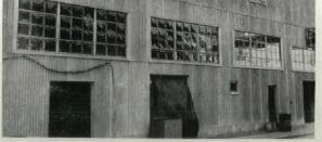
Explosion-vent windows that are lightweight and easily installed are used on Emery Industries which houses process using hydrogen.
