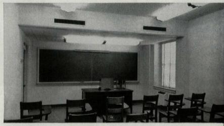
Classroom in Kirby Hall, Perkins Quadrangle. In this new Quadrangle, seven new buildings have been equipped with Barber-Colman Air Distribution products since 1950. Note double deflection "MA" Sidewall Diffusers which have integral volume control, easily removed cores.
