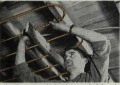
s are furnished with one end of the tube expanded. After cleaning and fluxing, PG's are connected by soldering or brazing. Many fittings are eliminated.
