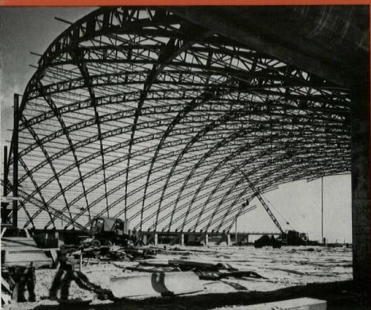
LAMELLA CONSTRUCTION—unusual in that the main members span supports on a skew, forming diamond-shaped areas between the intersecting members.
