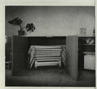
Built-in storage cabinets include space for aluminum cots stacked on dollies. Cork-tile wain-scoting runs around two sides of room, is used as tackboard.
