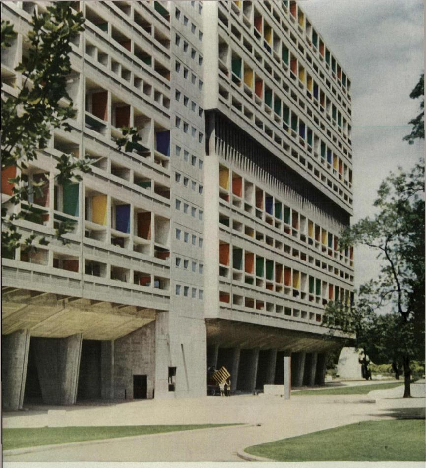
A colorful honeycomb, the 337 apartments and private balconies rest on 38 massive piles, each of which carries more than 2,000 tons. These piles, four men high, create a sheltered play area on the ground floor and are intended to make the big building seem lighter. The central vertical strips of small windows mark the stair well; the horizontal strip of louvers marks the commercial area,
