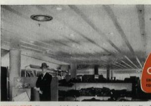
HUTZLER'S, Towson, Md. (above), uses special Kno-Draft High Pressure Air Diffusers that permit the air supply in a given area to be changed without unbalancing the air delivery of the other outlets, or creating objectionable noise. Installed cost comparable to conventional system.
