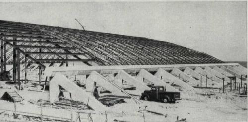
THE MAIN MEMBERS—circular steel arches—spring from concrete buttresses along the sides of the building. They span 224 ft. with a rise of 30 ft., providing a 42 ft. clear height at midspan. Main and intermediate purlins are spaced about 6 ft. apart.
