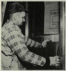
Workman easily cuts FOAMGLAS blocks to fit between steel frame members of sub-structure.
