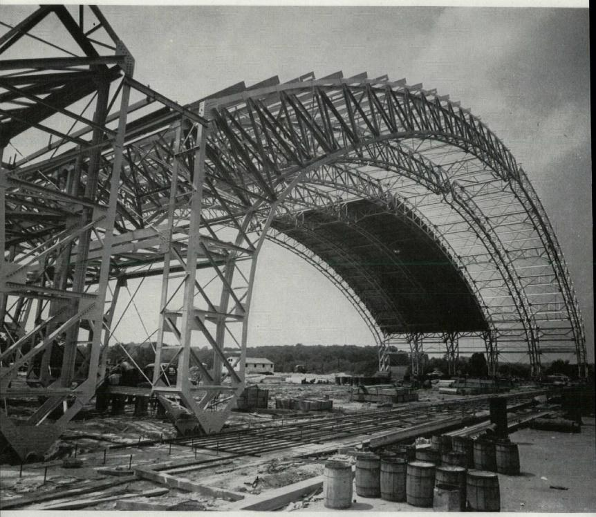
Completed frame (above) is roofed with ribbed galvanized steel sheeting and suspended glass-fiber insulation boards. Note longitudinal bracing.
