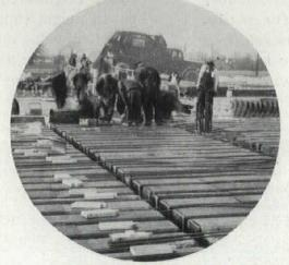
One-way Ceco-Meyer Steelforms also save steel and concrete, thus reducing dead load.
