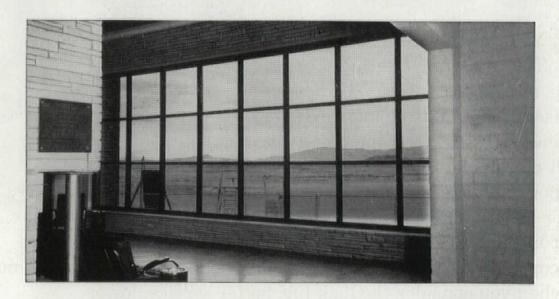
Thermopane insulating glass in the Prescott (Arizona) Municipal Air Terminal Building helps insulate the building against both heat and cold... saves on heating costs.
