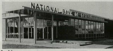
National Bank of Detroit. Architects: Hawley, Ellington & Day, Detroit, Mich. Featured is Alumiline Curtain Wall Construction (60% of total wall area). The Curtain Wall contains both glass and porcelain insulating panels, with the construction based on  $2'' \times 5''$  tubing. This Alumiline Curtain Wall was sent to the job completely prefabricated.
