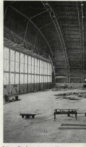
Bottom-rolling doors, 40' high and 255' long, are electrically driven, nesting into pockets at sides. Each hangar is fully sprinklered, heated by unit space heaters.
