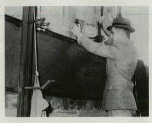
Grouting machine forces mortar into stonework (p. 194)
