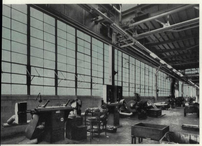
Filtered Daylight through Frosted Aklo Glass in the Goss Printing Press Co. plant, Chicago. Architects: Olson & Urbain, Chicago.
