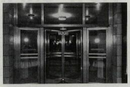
alone is \$4,700.) Since the units will fit under or against transom bars (usually 7' to 7'-6") without tricky alterations, and connections between mullions of revolving doors and swing doors are already engineered, the packaged entrances are especially economical for remodeling work.
