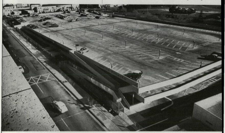
Diagonal parking on 4% slope means only 1.6% slope in direction of parking stalls. Bumpers between stalls are 27" wide and 3" high
