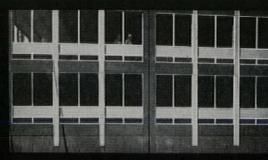
CAST ALUMINUM SPANDRELS are lightweight yet sturdy. They are easily handled, quickly anchored in place. Maintenance costs are extremely low.
