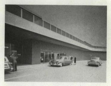
Pickup station at Hudson's receives packages on underground conveyor, has them ready for customer car pickup 15 minutes after purchase. Ramped bus road is above. Supermarket has pickup at ground level, also serviced by an underground conveyor (see plan).
