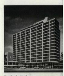
Hartford Statler, now nearing completion, expresses conventional construction with aluminum cover plates over spandrel beams and columns. Dallas Statler's cantilevered structure is revealed on lower public floors (photo, opp.) and concealed behind curtain on upper floors.
