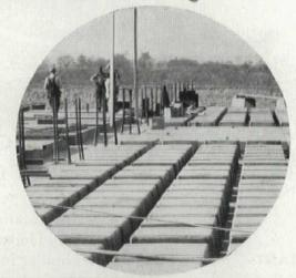
Two-way waffle design using Ceco-Meyer Steelforms permits longer spans, resulting in larger uninterrupted floor areas.
