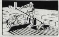
Excessive amounts of asphalt are eliminated on Robertson Q-Deck because the adhesive is applied to the *insulation* . . . not to the steel deck. This also results in a better bond between the steel and the insulation.
