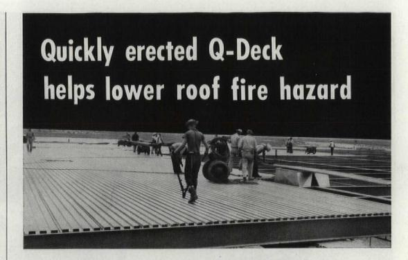
The many unique features of Robertson Q-Deck make it of special interest to the architect and engineer who is concerned about the fire hazard aspect of his flat roof design. Robertson Q-Deck is designed with tight side and end laps to eliminate the need for an inflammable vapor seal. Its two-foot width and long span characteristics mean fewer joints and its surface is either zinc coated or basic Galbestos.
