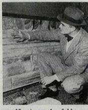
limestone, 15 minutes for fieldstone, to 30 minutes for granite and marble. After each setting, the machine is released, leaving stone and seams smooth and clean, and raised to the next level. Units can be interlocked in tandem around an entire building for really fast production. Walls built with the Foam-O-Matic have been found to conform to strict building codes.
