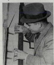
stonework and let a pressurized steel form faced with foam rubber do the work of forcing the grout in and around the stones or brick. Concave joints and stone faces need
