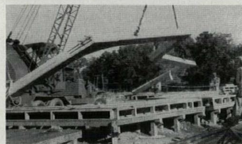
Hoisting of frames is done by truck crane
