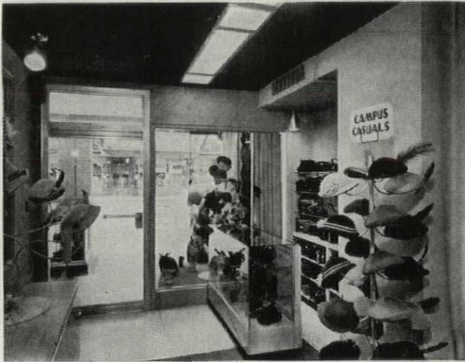
CEILING MOUNTED Type BT Cabinet, connected to duct with inlet at floor level, replaced a bulky, unattractive cast iron radiator that formerly was located below show window.
