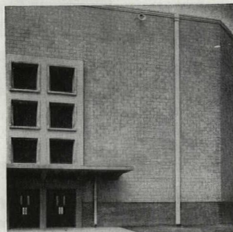
42'-HIGH wall shows fine masonry wall of Duraplastic-made block. True edges, pleasing color and texture of Duraplastic block help assure better-looking block jobs.
