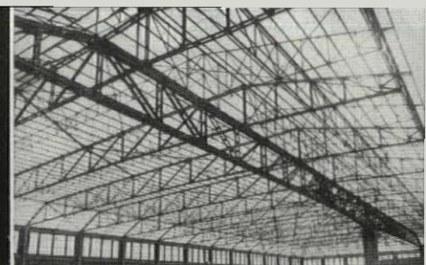
Prestressed girder spans 502' over single column in Belgian hangar. Two sets of high-tensile cables are used, a set anchored at each end of the lower ends of the truss, extending over the central support and terminating at about the third point of the other span.
