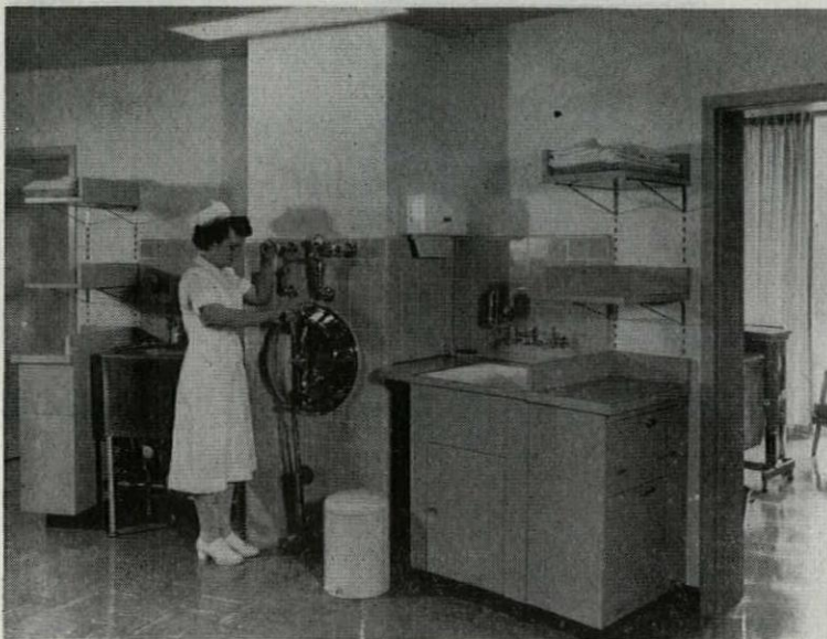
Utility unit (designated D on plan, p. 108) has sink, instrument sterilizer, bedpan washer and sterilizer, waste can, storage and same receptacles for bedpans and soiled linen as other units.
