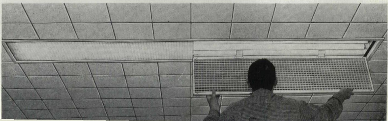
No screws or other devices mar the appearance of the troffer trim
