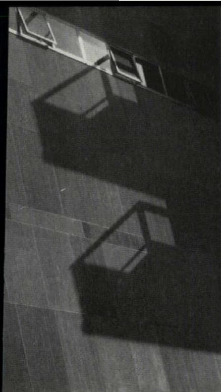
Stone veneer of Philadelphia Youth Center is laid vertically like veneer.
