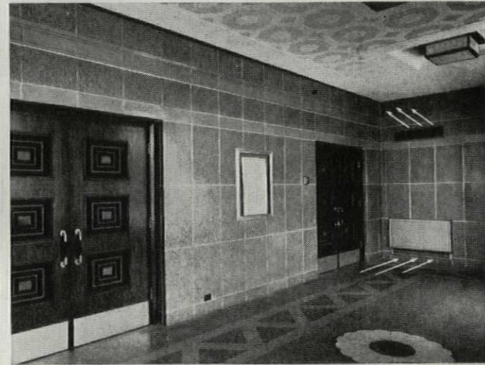
HARD-TO-HEAT CHURCHES offer no problems for Modine Cabinet Units. Here cold air, drawn into opening in bottom of unit, is heated and discharged through wall grille.
