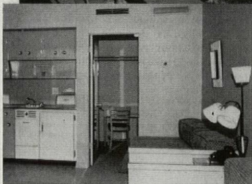
Typical apartment of Sahara Motel, showing outlet (over door) for conditioned air and return air grille. Occupant can adjust thermostat to secure temperature desired, or shut off cooling or heating entirely.
