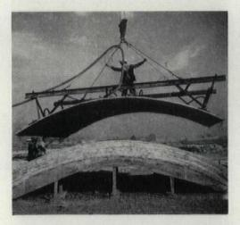
Precast barrel shells, 16'-8" wide, 17' long and 11'4" thick are cast atop one another using the rapid-curing vacuum process. Each barrel acts as formwork for the next.
