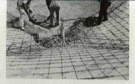
Topside reinforcing of umbrella roof shows diagonal steel layout, with extra stiffening of main compression beams.
