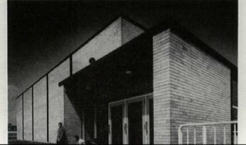
Handsome entrance to auditorium-gymnasium wing. Bents of structure are left exposed in brick exterior wall. Central courtyard is sunk below ground level of classroom wing, functions as service space for the shop wing (right). Gym-auditorium wing (at left) has wide gallery windows.
