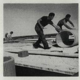
than conventional 4'-wide panels. Fewer joints not only mean less labor but also less chance of leaks on outdoor applications and neater jobs indoors. Flexible enough for a 100' strip to curl into a 25" x 3' carton, the material has high impact resistance. Made in 1'-to-5' widths, it can be ordered flat or corrugated, shiny or dull, rippled or smooth at \$1.25 psf. Spun-Lite Corp., Miami, Fla. (Jan. '54, p. 192).
