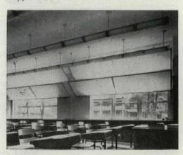
GLASS-CLOTH PANELS. Simple white shades of woven glass yarn soften intense sunlight and distribute it throughout a room. Easily constructed for old and new classrooms with large windows, the durable cloth diffusers are fireproof and rotresistant. The fabric comes in light and heavy weaves (for different orientations) at 17¢ and 23¢ psf. Owens-Corning Fiberglas Corp., 16 E. 56th St., New York, N.Y. (Oct. '53, p. 248).
