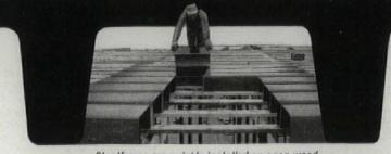
Steelforms are quickly installed on open wood centering. Cost is reduced because same lumber and Steelforms are re-used from floor to floor.
