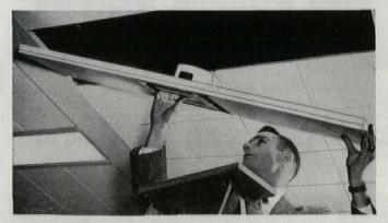
**EASY TO INSTALL** as the acoustical tiles themselves, Kno-Draft panels snap quickly into place. Ducts and flexible connections are readily accessible and connections can be made in a matter of minutes.
