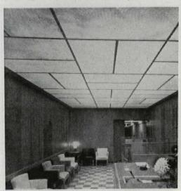
HONEYCOMB CEILING. Expanded sheets of 3/32"thick aluminum honeycomb on standard suspension supports comprise Honeylite fireproof dropped ceiling. Masking overhead pipes and ducts, the light (1 oz. psf) cellular panels also diffuse harsh glare from bare-bulb fixtures above into flattering illumination, and break upthereby softening-noise from below. Honeylite Co., 576 W. Grand Ave., Oakland, Calif. (May '54, p. 204).
