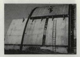
Precast lower panels, 22' high and 16' long, facilitated construction of this 85'-wide 200'-long and 41'-high St. Louis Waste Material warehouse in Fort Worth, Tex. Upper part of shell and the ribs between them were cast in place using traveling formwork. Consulting engineer: Eric C. Molke.
