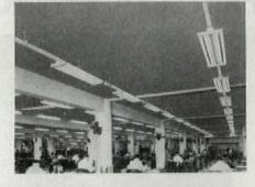
In this building, UNISTRUT channel was used to support and wire a lighting installation on a concrete ceiling. Savings over conventional methods of installation were estimated at 50%! Note the neat, perfect rows of fixtures.
