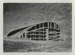
Circular coliseum is spanned with 286' span ribbed arches springing from footings 375' apart at the Alabama Livestock Coliseum. A 3½"-thick shell is carried by 2' x 3½' ribs 28'-4" o.c. Architects: Sherlock, Smith & Adams; structural engineers: Ammann & Whitney.
