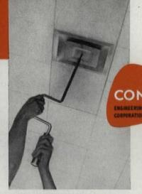
DAMPER ADJUSTMENT to control air volume can be made quickly and easily after installation. Exclusive Kno-Draft sleeve type damper regulates volume without affecting air velocity.
