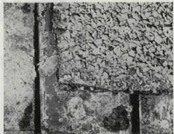
Conventional roof after fire shows how vapor barrier has disappeared, revealing deck joints.
