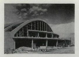
Ribbed arches span 253'-8" at the newly completed Denver Coliseum. The 400' long shell roof is 4" thick, built with traveling formwork in six 56' long units, each supported by three 20" x 41/2' deep ribs. Architects: Lorimer & Rose; engineers: Roberts & Schaefer Co.
