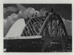
Coupled hyperbolic-paraboloid shells, %" thick, span 33' over the Cosmic Rays Pavilion at University City, Mexico.
