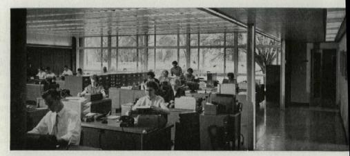
General office has all-purpose ceiling (radiant panel heating and cooling, acoustic control). Chosen late in program, it faced delay, "but was worth it."
