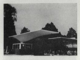
Asymmetrical umbrella roof is cantilevered 36' to one side and 14' to the other. The structure is balanced by 8" concrete in short span.
