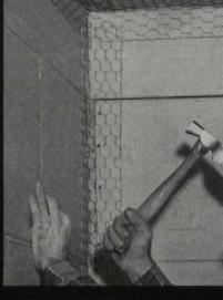
Preformed—Keycorner is preformed for corners, joints, ceiling junctures. Flex it and it fits right in.
