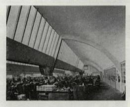
North-light shell framing applied to a Zeiss-Opton optical plant at Oberkochen, Germany. Engineers: Dyckerhoff & Widmann.
