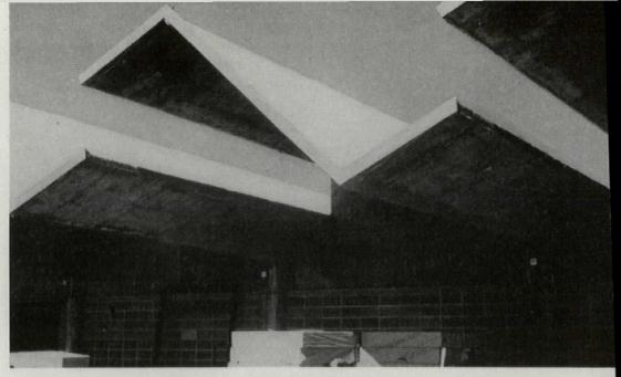
Z-shaped slabs are contilevered 22' at each end from their supporting columns. Each slab is carried on two columns spaced 75' apart. Shells are 4" thick and are laterally braced by
