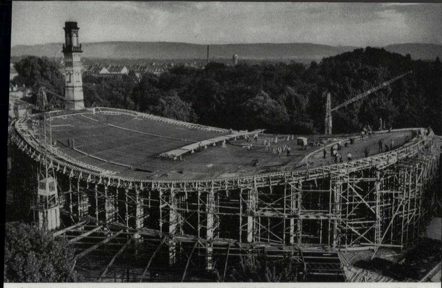
Reversed dome under tension is suspended from a peripheral compression ring to roof a 160' x 240' assembly hall at Karlsruhe, Germany. Held by prestressing cables between outer columns, this catenary surface has a slight countercurve at midspan to aid drainage. Engineers: Dyckerhoff & Widmann.
