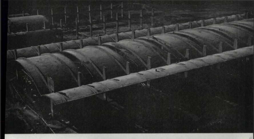
Short barrel shells of 66' span and with 20' cantilevers on each side compose a 720'-long Custom House warehouse in Mexico, D.F. In the background (above) can be seen the traveling formwork, which could be used by placing the tie bars above the roof (right). These tie bars are of high-tensile steel and are tensioned by jacking (below).
