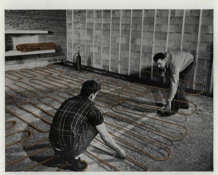
YOU CAN EXTEND or contract ¼" PG's easily by hand to meet all desired c-c spacing requirements within a range of 6 to 18". William Sincox, Heating Contractor, Union, N. J. says: "My men find PG's install faster...make a neater job"
