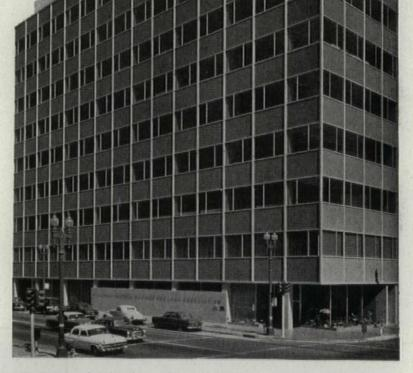
SEAPORCLAD\* Insulated porcelain panels (flat-as-glass) are of sandwich construction combining the use of various cores laminated under high pressure to skins of diversified metals. It is available in the widest range of textures and colors to harmonize with practically every type of structural material and architectural mood. SEAPORCLAD is permanent and of lasting, indestructible beauty.
