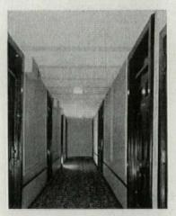
5. New false ceiling hides ducts with new lighting and acoustic tile.
