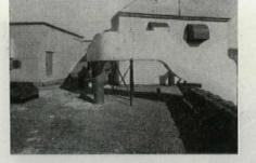
1. Penthouse fanrooms supply 58° air to two vertical main ducts at 4,000 fpm.
