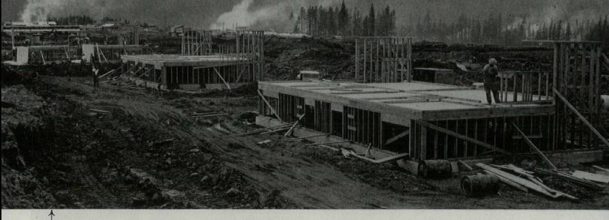
Houses, 300 at a crack, are produced by Johnson & Crook's expert building operation. Made of prefabricated sections, the houses are set one-half story into the ground.
