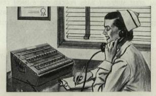
No more running to patient's bedside to reset station when nurse releases "talk" button after completion of call, station automatically resets... cannot be accidently reset.
