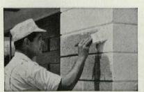
FOR POROUS SURFACES... Latex paints have excellent sealing properties over cinder block, concrete block and many other porous surfaces.
