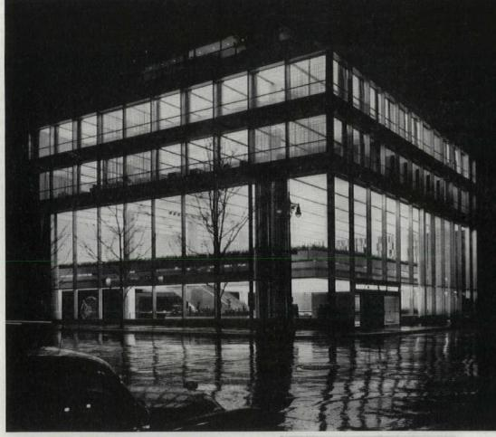
GOLD IN A GOLDFISH BOWL resulted when Manufacturers Trust gave its architect a free hand to design a new branch. Big windows hang between thin aluminum mullions. The vault is separated from the sidewalk only by 1/2" of glass, 10' of air (and a 30-ton door). It has snooperproof numbers on the rim of the combination knob. George A. Fuller Co. was general contractor.
