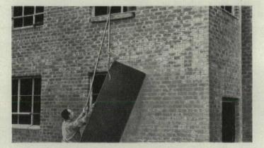
**7.** All set. Lather inserts baling hook into bundle and hoists with block and tackle to desired floor. Every sheet is uniformly rectangular. Every corner a perfect 90°.
