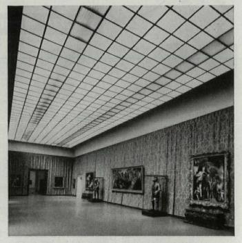
Ceiling in this room is of specially designed panels of waterwhite crystal by Corning. Louvers of Alba-Lite shield directional lighting used to highlight centers of attention.
