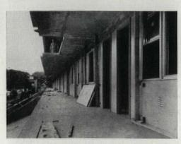
Interior of wall is ready for lining and partitions. Louvers in panel beneath windows are inlets for
