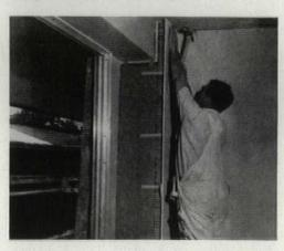
Plaster board finish is applied to column fireproofing. Partitions are clipped to shoe and header then plasterboard is glued to both sides.
