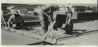
concrete fill is placed over welded-in-place deck and steel mesh. This insulating slab weighs only 5 lbs. psf for a 2½" average depth. (Insulation value equivalent to 1" of insulating board.)
