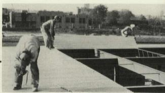
steel sheets are quickly placed and secured by welding or by clips attached to top of joist. Attachment of sheets makes roof rigid, provides working platform. Special Granco tough-temper steel takes construction abuse—adds safety factor.
