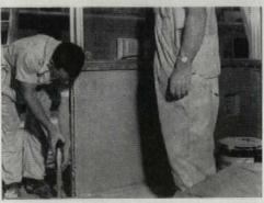
Porcelain enamel wall panels are joined to wood shoes by plugs driven into floor slab by powderactuated tool.
