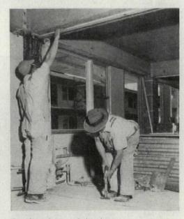
Wooden shoe and header for partitions are fastened to concrete floor slab and beam by powder-actuated fastening gun.
