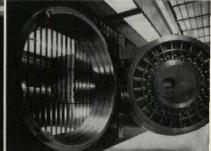
Special round vault door at new Manufacturers' Trust building in New York was a three-way collaboration among Mosler, Architects Skidmore, Owings & Merrill and Designer Dreyfuss. Thrusting tons of steel 8' out from the hinge, such a unit costs 50% more than a standard model.
