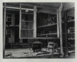
Window frames are hung from soffit beams. Alongside window frame is lagged chilled water pipe and steel column.
