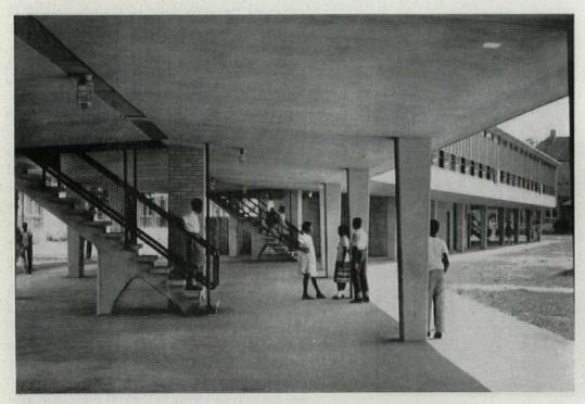
Stairs lead from playspace to entrance and utility core between each pair of rooms. Pipe stack can be seen behind stair. Larger ground-floor enclosure toward rear houses toilets.
