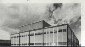
Simple wall components are varied and rearranged to produce a variety of effects. Among the most cogent is the glass topped and bottomed window wall in the shop above, with a ribbon of porcelain enamel in the middle to kill glare. Top glass adds ventilation and daylight for inner part of deep room.
