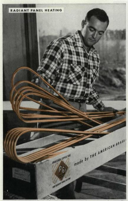
PG's are lightweight and easy to handle. They come packed in cartons, ready to install.
