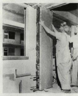
Column fireproofing is honeycomb core with granular perlite filling. Paper core panels are easily cut to fit around conduits.
