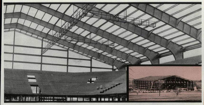
UNIVERSITY OF KANSAS BUILDS NEW FIELD HOUSE: More than 2,700 tons of structural steel went into the framework of new field house at the University of Kansas, Lawrence, Kansas. The structure features 10 rigid frames which provide a clear span of 250 feet. The frames, which weigh 80 tons each, are completely welded, and were produced simultaneously in Allied's three plants at Chicago, Illinois, Ham-
