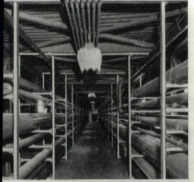
In this tunnel between two buildings, pipes of all sizes and types are supported on strong UNISTRUT framing. Exact slope and pitch are easily attained because of the adjustability of this system.
