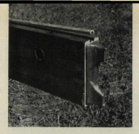
Laminated framing members,  $91/2'' \times 21/2''$  and 12' to 14' long, are fitted with steel shoes that butt against 1" dia. pin in each joint. Members are secured by cables around joint.
