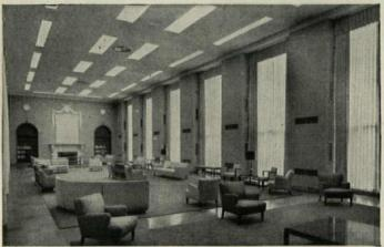
Spacious "browsing room" with Venturi-Flo Ceiling Diffusers above, Uni-Flo Sidewall Diffusers and Return Grilles on the firred panels between windows. Each ceiling diffuser has integral volume control for simplified balancing of system.
