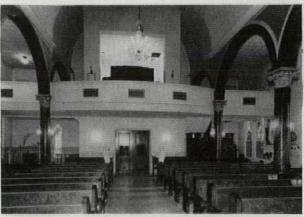
Five discharge grilles at rear of church and two large return grilles are the only visible signs of air conditioning inside the building.
