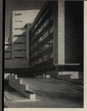
MAIN FACADE is mostly marble. It is %8" thick, backed up by 1" airspace, then 4" perlite block, metal lath and plaster. Building is completely air conditioned, and windows on sun walls are kept small.
