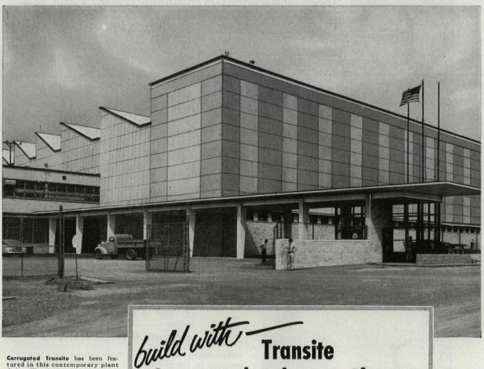
Corrugated Transite has been feacorrugated transite has been fea-tured in this contemporary plant design. The shadow lines of the cor-rugations provides decorative inter-est for the large wall areas.
