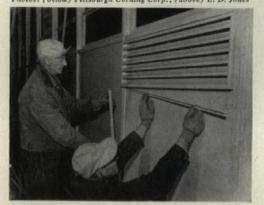
Erection of panels, each weighing 180 lbs., is carried out by two-man crews, who average 6.9 sq. ft. of spandrel wall per man-hour. Sand-colored porcelain enameled panels are caulked, then secured by steel angles at top and sides.
