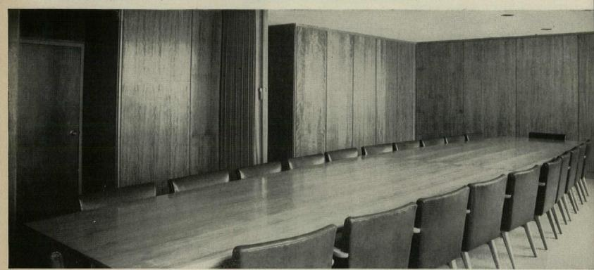
HALF-INCH RED BIRCH WELDWOOD was used to achieve this unique method of paneling in conference room,  $\frac{3}{4}$ " recessed joints are backed by strips of white birch plywood. Stay-Strate Door is birch. Sliding door acts as room divider when necessary.
