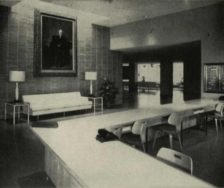
BIRCH WELDWOOD was used to construct this ultra-functioned reception desk. Wearproof, easy-to-clean white Micarta was used for top. Weldwood panels in various thicknesses and wood faces are especially suitable for built-ins.
