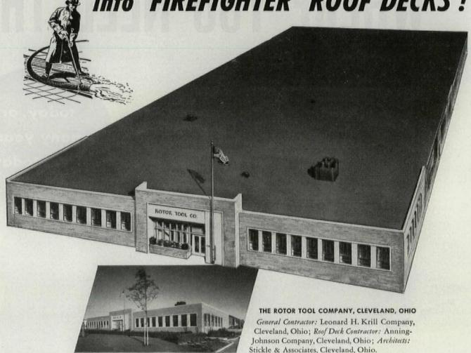
One of Rotor Tool Company's best protections against fire is the Gold Bond "Firefighter" Roof Deck poured over its new Cleveland plant. Incombustible gypsum—39,000 square feet of it—covers the building with natural fire-resistance. Gold Bond Insulation Formboards also provide this installation with a heat reduction coefficient of .18.
