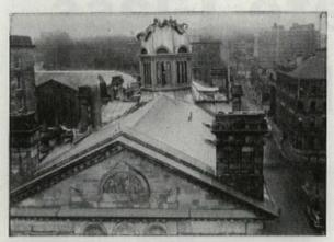
Changes under way. Workmen begin demolition of cupola atop the Old Post Office Building in Halifax, N.S. The entire slate roof is scheduled to be replaced by an all-Monel standing seam batten roof.
