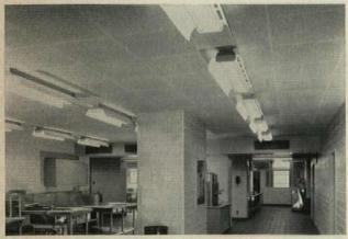
This low-cost ceiling material is not only completely fireproof and easy to clean, it's also highly efficient. Noise, bouncing off the many hard surfaces in the kitchen, could build up to disagreeable levels were it not for the ceiling of Armstrong Perforated Asbestos Board.
