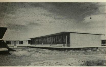
Deep 7'-6" overhangs shade window walls, create covered walks for maintenance staff and for guards checking on prisoners. Crawl spaces may be sealed off by skirt of precast concrete planks. Contractors: R. P. Farnsworth & Co., Atlas Construction Co., S. J. Lemoine Co.
