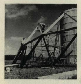
Erection of space frame is done from light scaffold after silos are built inside dome. Because framing members are connected by rigid joints, they exert no lateral thrust on foundations.
