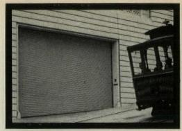
25'x 19' Cookson Power Door (Type FCM-B) with special sloping footpiece. 1 hp motor supplies ample power for .67 ft./sec. operation.
