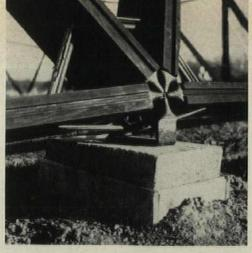
Perimeter joints atop footings are braced with steel spacers as well as cables, to prevent horizontal members from being forced upwards. The dome is mounted atop 20 such footings.
