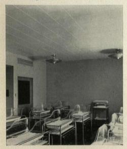
In the new unit of Lancaster's St. Joseph's Hospital, three distinct sound-conditioning problems prompted the use of three different acoustical materials—Armstrong Travertone\*, Arrestone®, and Perforated Asbestos Board.
