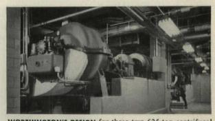
**WORTHINGTON'S DESIGN** for these two 625-ton centrifugal refrigerating units called for special finned aluminum tubes for condensers and coolers.
