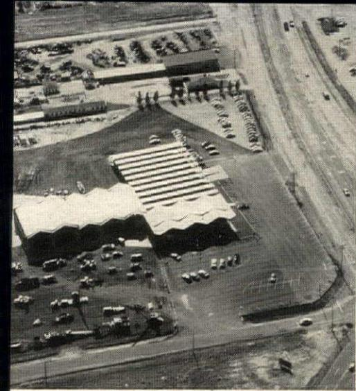
**Air view** of equipment factory shows shop area on left, with 36' x 80' folded plate slabs, a display area in front with 40' x 80' folded slabs cantilevered 28' forward of supports, and an office and parts area in rear with Z-shaped north-light slabs.
