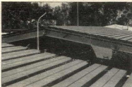
**PANELS** are laid over the rigid steel frame during course of erection, combining in one unit acoustical ceiling, joist and deck. Be sure to investigate before you plan your next building! Once your building is started, it's too late!
