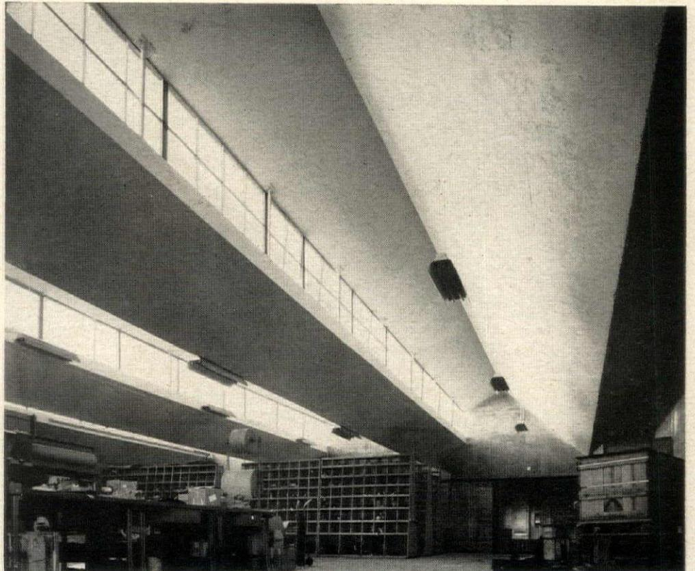
**"Z"-slabs** 18' wide and spanning 75' between columns cover parts department. Folded slabs, only 4" thick, are braced by transverse diaphragm walls between columns. Continuous clerestory windows between Z-slabs are 33" deep.
