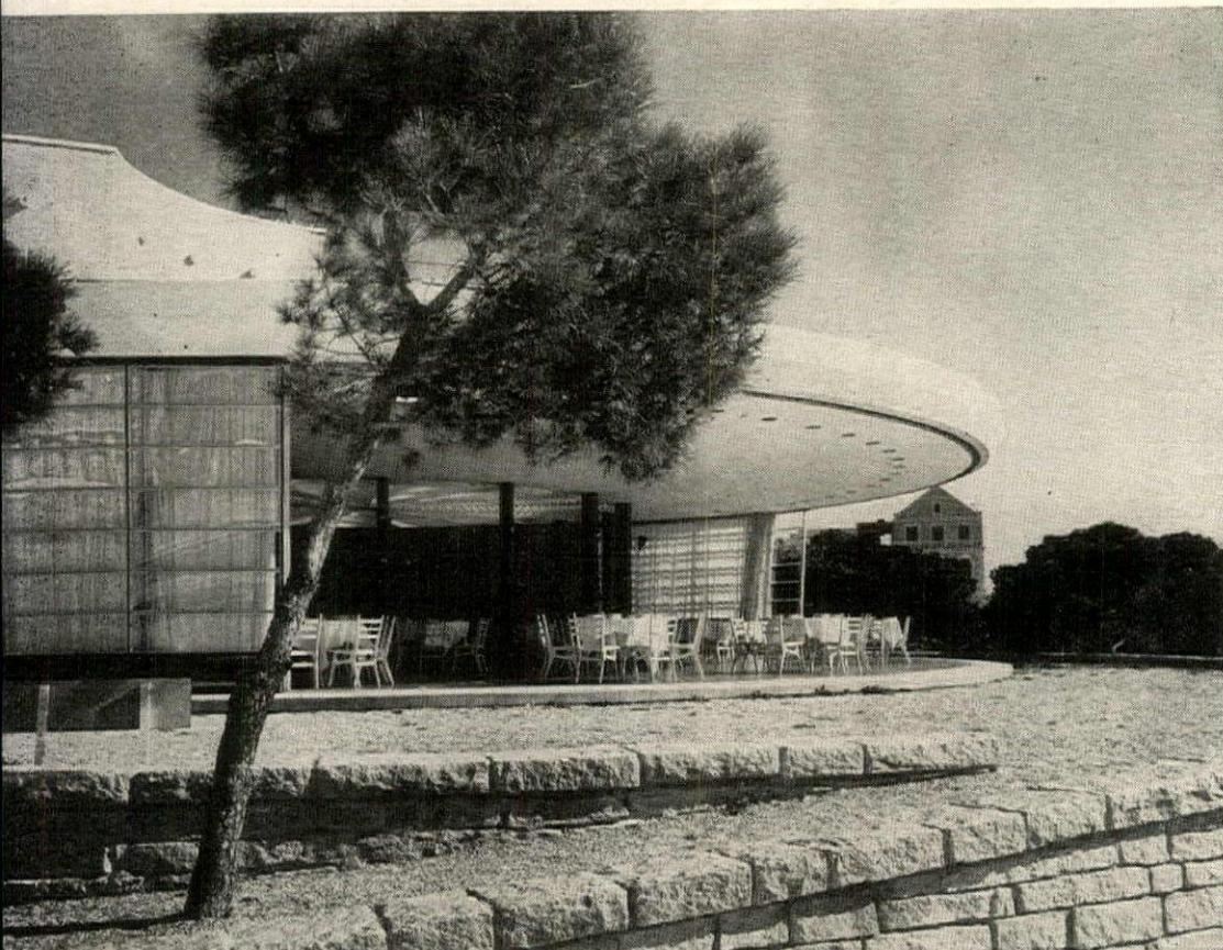
**CIRCULAR RESTAURANT** at Madrid's Concrete Institute is built like a huge mushroom—the roof is cantilevered out about 23' from a central ring of columns. By rolling back the glazed wall panels, more than half of the big room becomes an outdoor dining terrace (above). At the center, inside the ring of columns, is a fountain and a planting area
