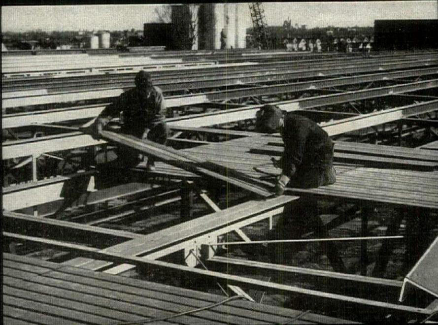
Time is money on every building job. Milcor Steel Roof Deck gets operations under cover fast at low labor cost, gives ideal base for permanent roofs.
