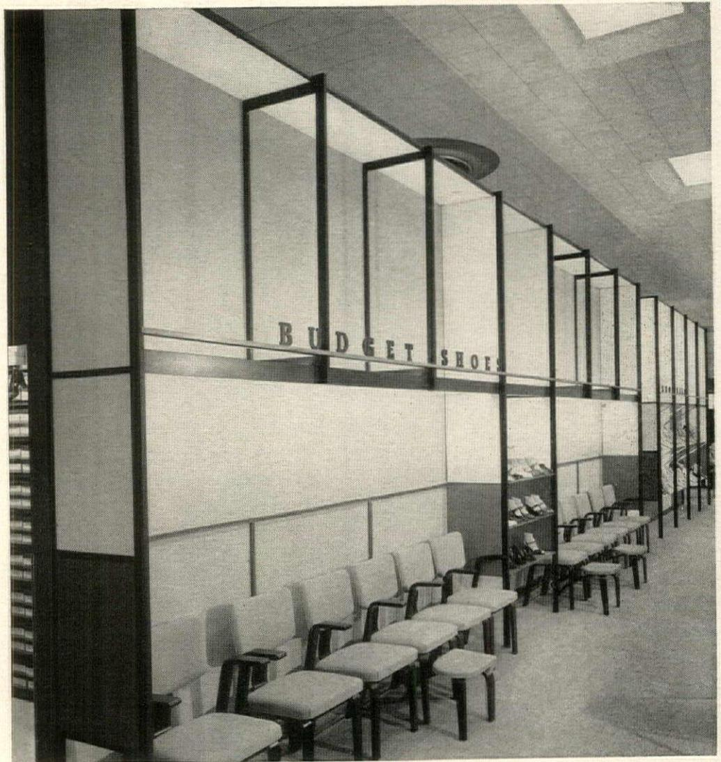
**ONE-WAY FIXTURES** are backed by stock cabinets to form storage-display partitions. Photos show design variations to accommodate shoe-fitting chairs, sporting goods and glassware. Note wide variety of materials used with standard hollow metal framework.
