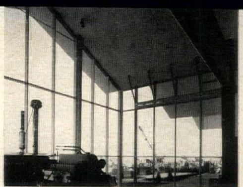
**Display room** is roofed with cantilevered slabs. Thrust is taken by tie beams between columns (seen at right of photo).
