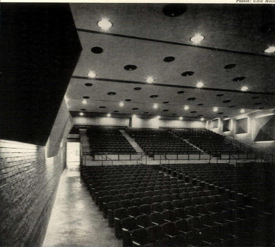
**AUDITORIUM** has 1,100 seats, a sloping "stadium" balcony that does not separate the audience sharply in half. Acoustical "pyramids" of varying sizes and depths were introduced to break up reverberations between parallel walls, conceal indirect background lighting. Roof and hung acoustical ceiling is carried on 84' steel trusses.
