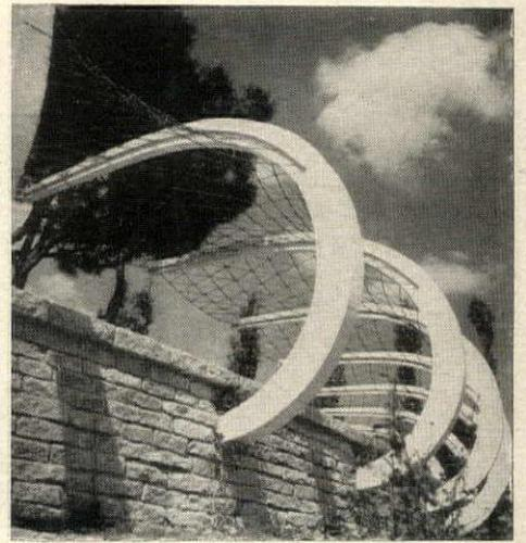
subtle but important elements of the design. The frames are about 16' long in plan and, like many other parts of the project, were prefabricated in a central casting yard.
