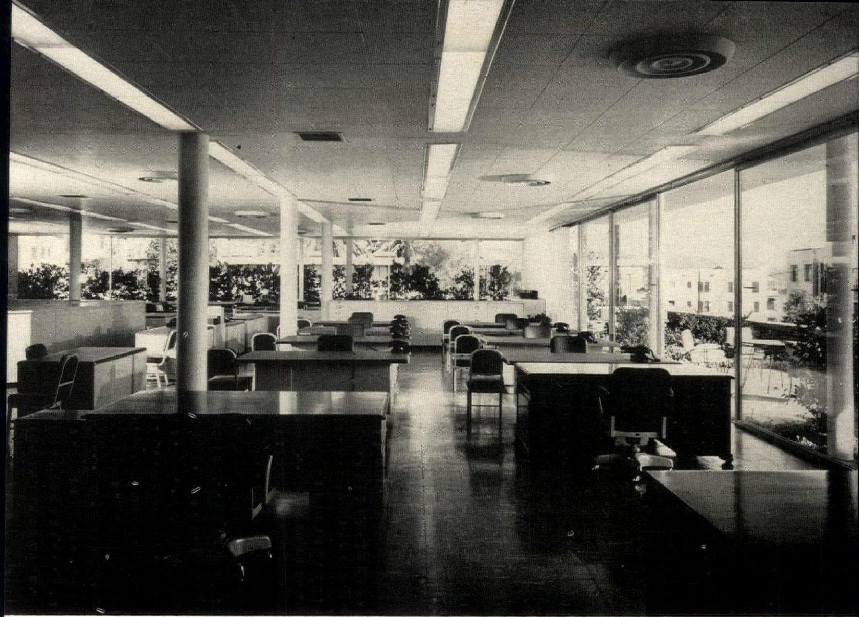
**GLASS AND GREENERY** are the walls. Glass walls on two sides of the big one-room office let the occupants enjoy the greenery of the planting strip (beyond) and the terrace (right). File cabinets (left) are kept low. Openness preserves the inspiring characteristic of the lift-slab construction.
