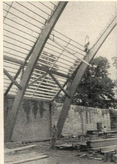
**K-trusses** of laminated timbers up to 9" x 24" in section span 25' between arches.
